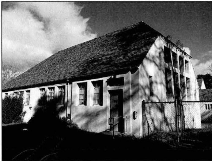
Photograph A.147. Looking north, showing the southwest elevation. A grouping of multi-light windows is shown on the southeast elevation.
