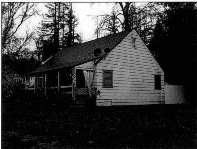
Photograph A.184. Looking southwest, showing the front, east elevation and the side, north elevation.
