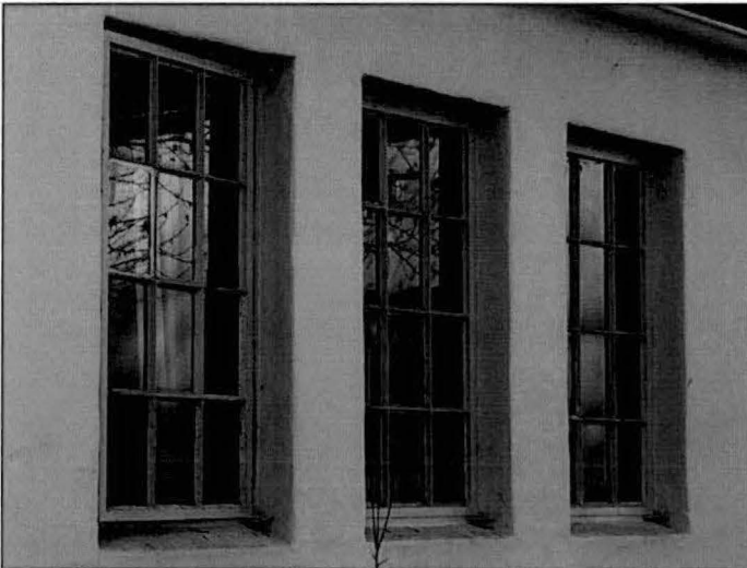
Photograph A.221. Detail of metal multi-light casement windows.
