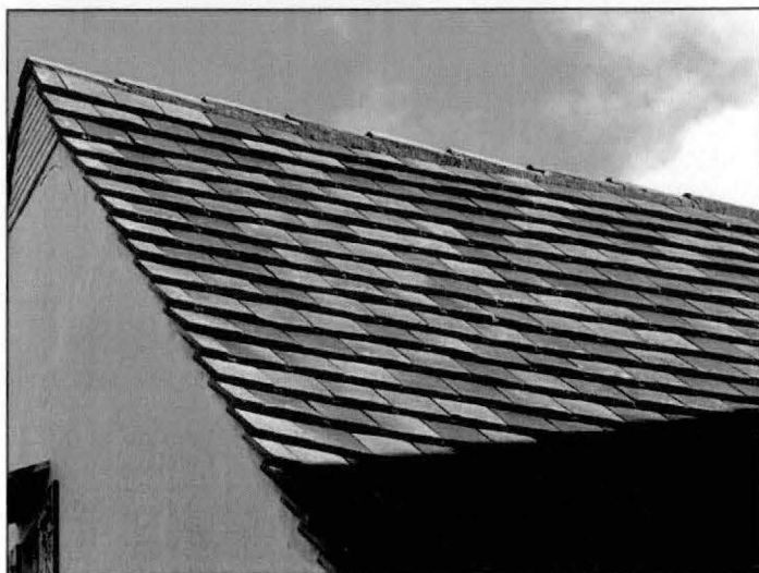
Photograph A.78. Detail of the ceramic flat tile roof and eave-less gable.
