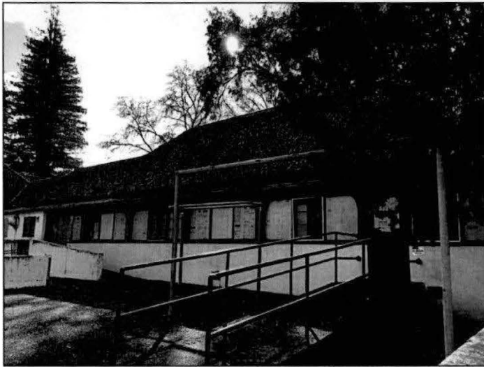
Photograph A.49. Looking south, showing the northeast elevation of Finnerty Cottage, which faces the inner courtyard.
