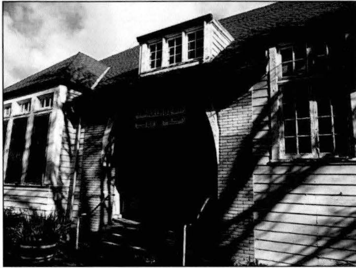
Photograph A.230. Looking north, showing the main entry at the southwest elevation.
