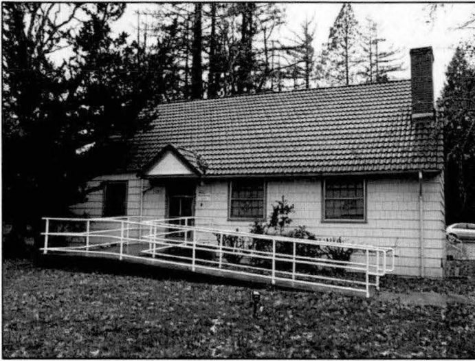
Photograph A.187. Looking west, showing the front, east elevation.
