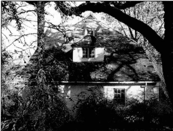
Photograph A.3. Looking northeast, showing the southwest elevation.
