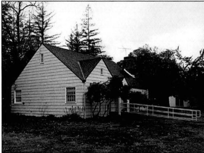
Photograph A.181. Looking west, showing the side, southeast elevation and the front, northeast elevation.
