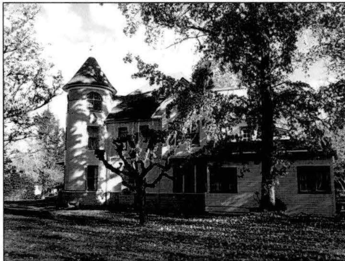
Photograph A.203. Looking northeast, showing the southwest elevation.
