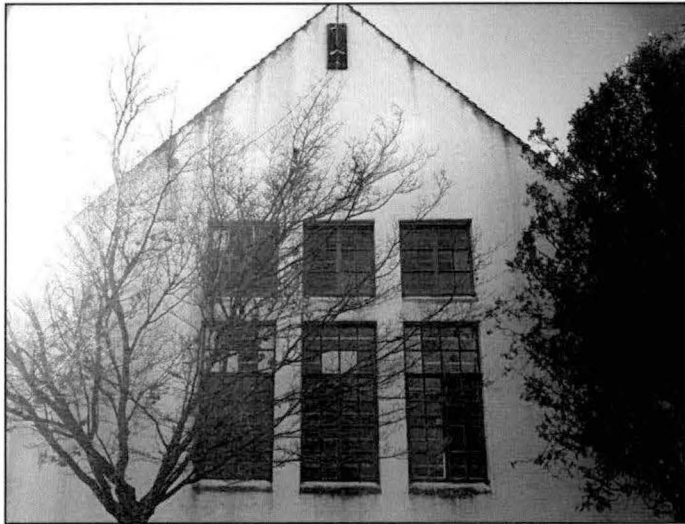
Photograph A.68. Looking south, showing the north elevation, and a grouping of multi-light windows.
