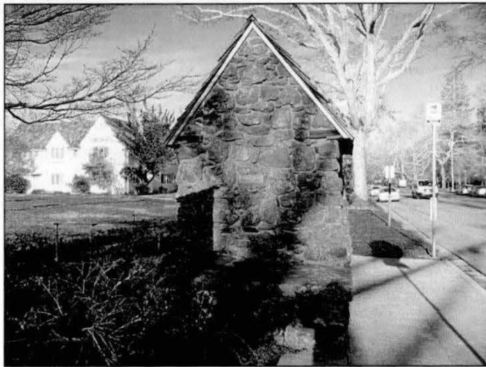
Photograph A.29. Looking northwest, showing the southeast elevation.
