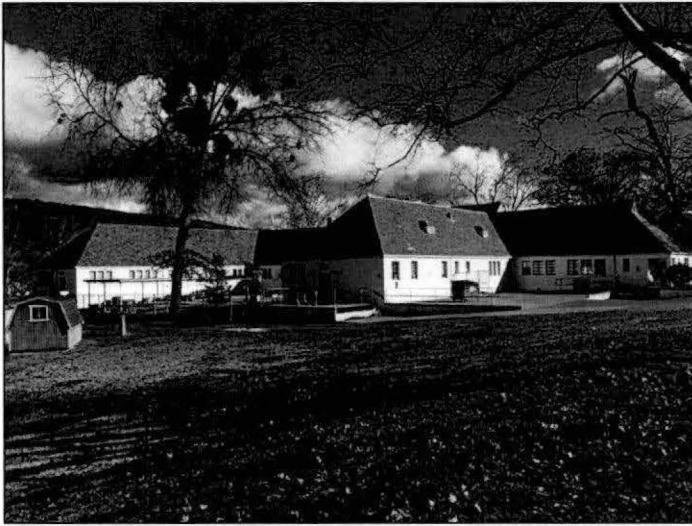
Photograph A.94. Looking west toward the southern end of the rear wing.
