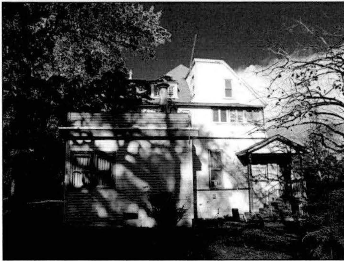
Photograph A.202. Looking northwest, showing the southeast elevation and side entry.
