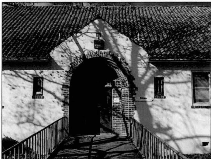
Photograph A.226. Looking northwest, showing the main entry at the southeast elevation.
