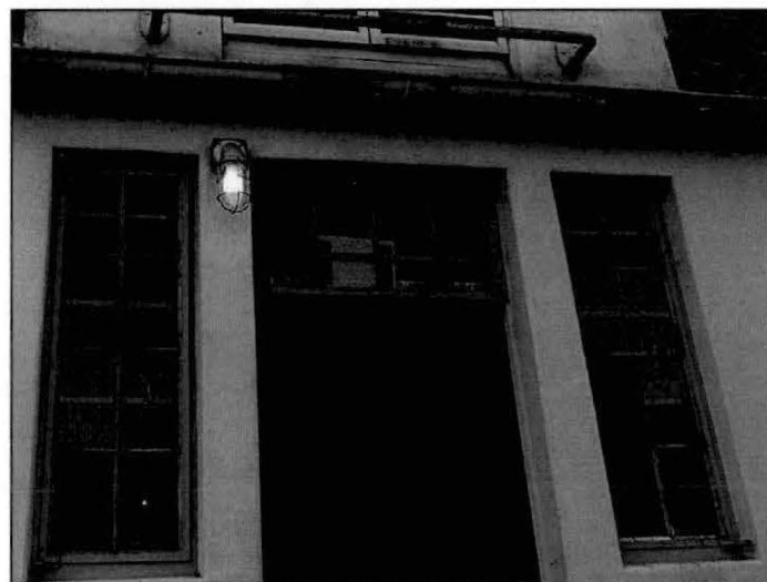
Photograph A.167. Detail of the metal multi-light windows on the north wing. Metal bars can be seen spanning the window reveals.
