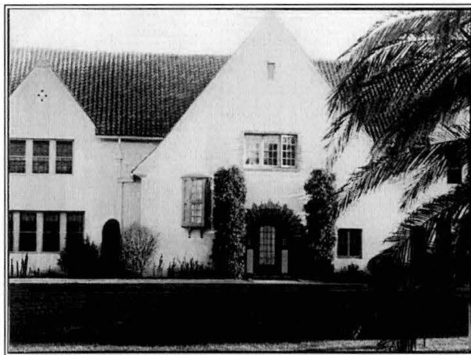
Photograph A.79. Undated historic photograph of Hatch Cottage, showing the northwest elevation. The oriel can be seen clearly in this photograph. 3
