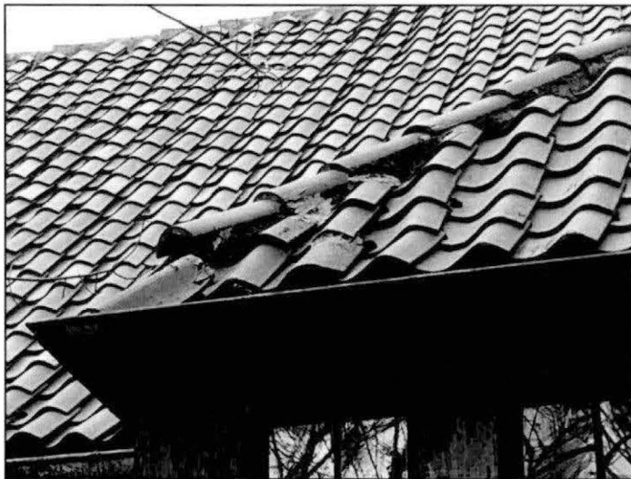
Photograph A.53. Minor biological growth on roof tiles.
