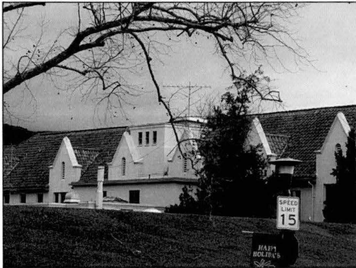
Photograph A.36. Looking east, showing the parapeted gables on the rear, northwest elevation.
