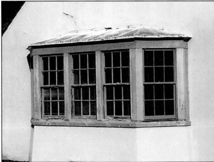
Photograph A.239. Detail of the 6/6 double-hung wood windows located in the projecting gable of the southwest elevation.
