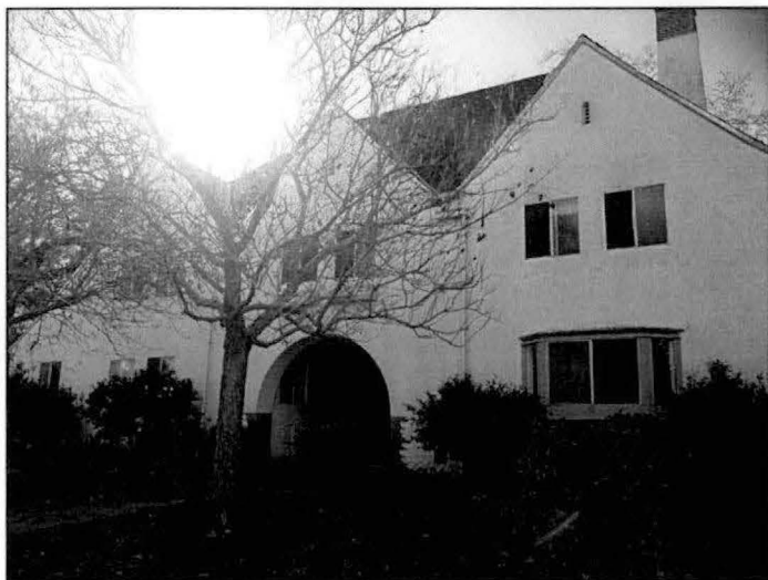
Photograph A.172. Looking south, showing the three prominent front gables and main entry.
