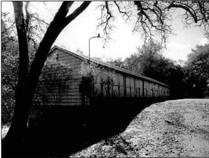
Photograph A.10. Looking south, showing the northeast elevation and the upper level garages on the northwest elevation.
