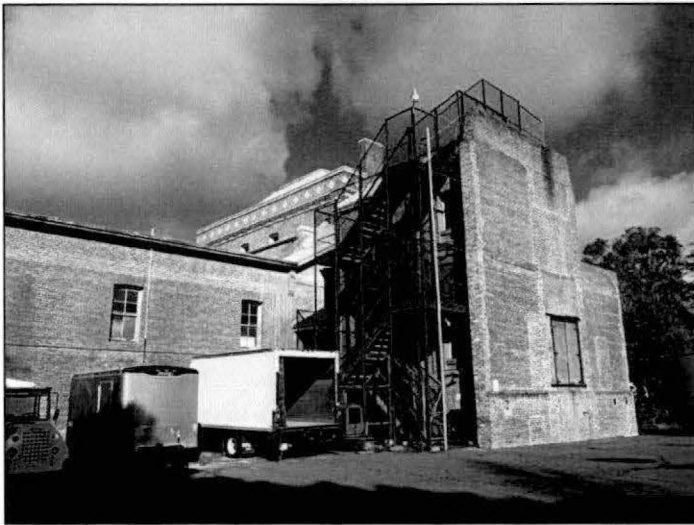
Photograph A.100. Looking north, showing the southern wing of the central core (1891). Remnants of the Judah Hall wing (now demolished) can be seen.
