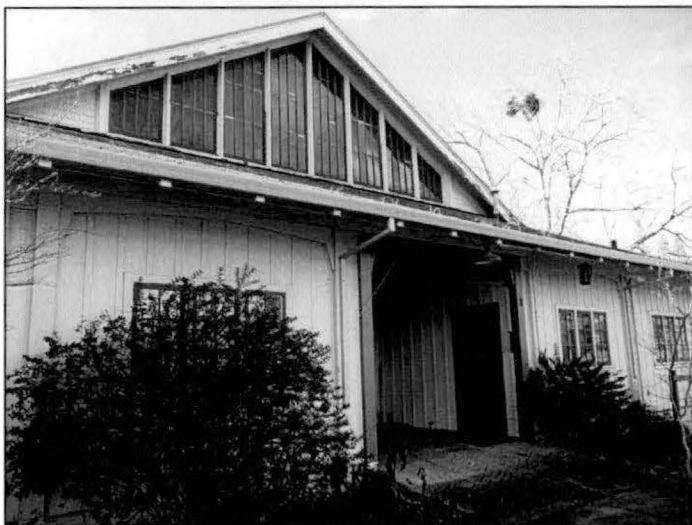
Photograph A.19. Looking west, showing the northeast elevation and the inset porch at the main entry.
