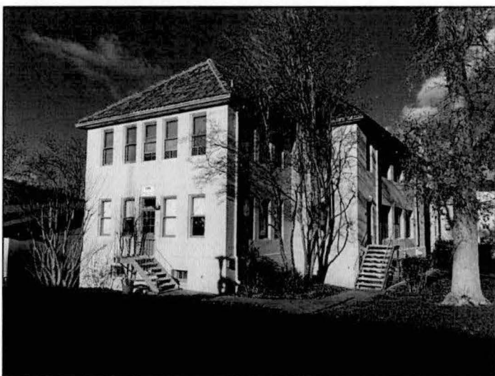
Photograph A.35. Looking north, showing the southwest side elevation and the southeast elevation.
