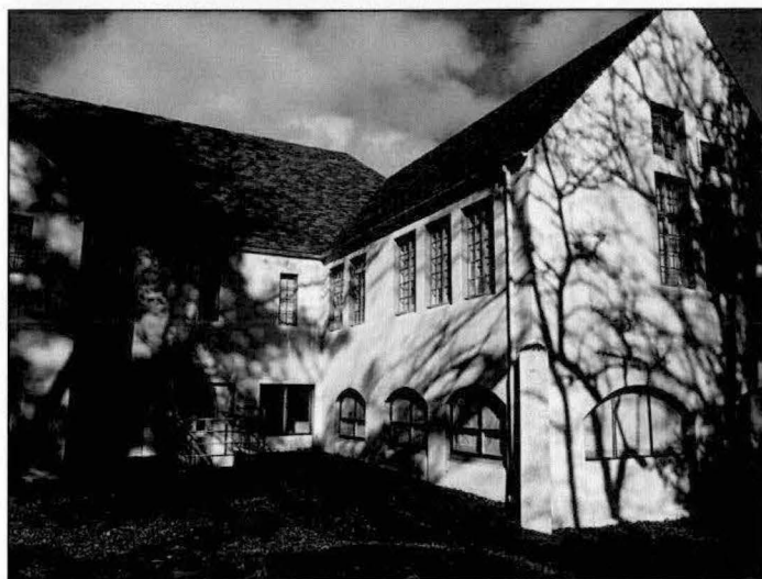
Photograph A.86. Looking west toward the southern end of the rear wing.
