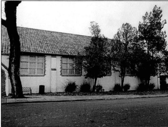
Photograph A.72. Looking north, showing the southeast elevation. The buttresses can be seen between the groupings of multi-light windows.
