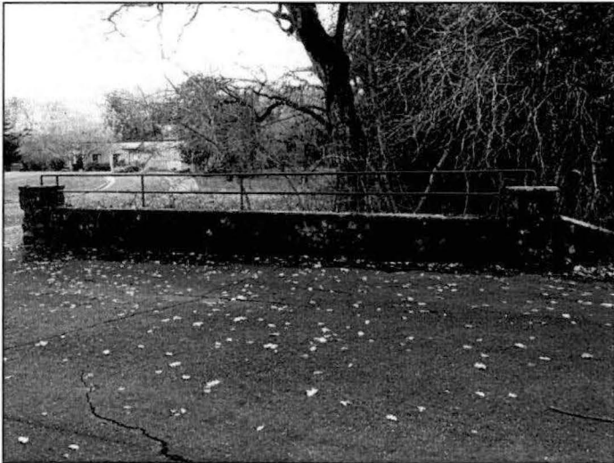
Photograph A.216. Looking west, showing the stone parapet and piers on the bridge's west elevation.
