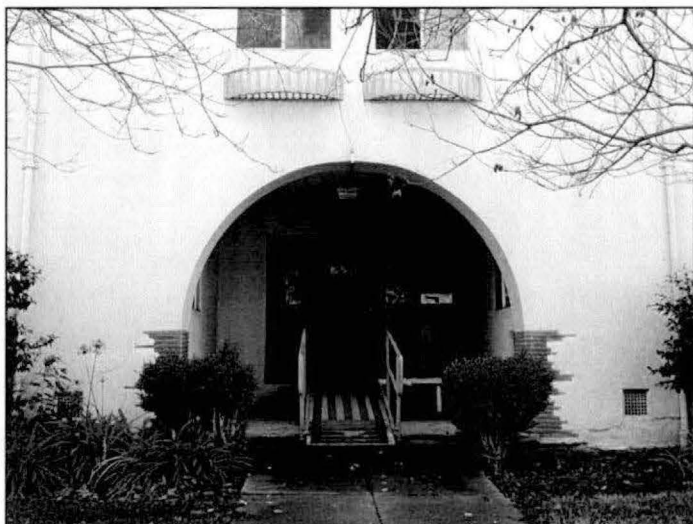
Photograph A.173. Looking southwest, showing the main entry arch with tabbed-brick, as well as the main entry door. Juliet balconies are visible above the entry.
