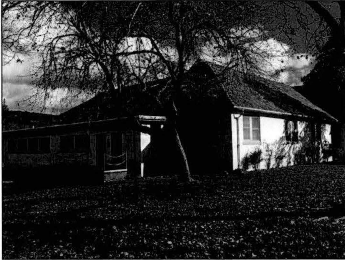
Photograph A.238. Looking east, showing one of the shed additions off the northwest elevation, and showing the southwest elevation to the right.
