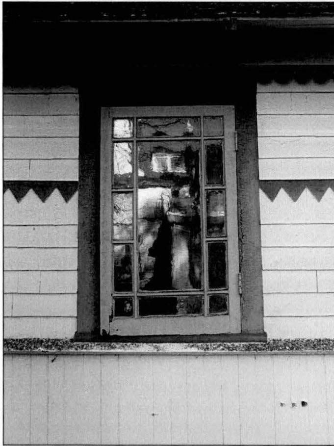
Photograph A.207. Detail of the wood window and shingle pattern on the 1891 building.
