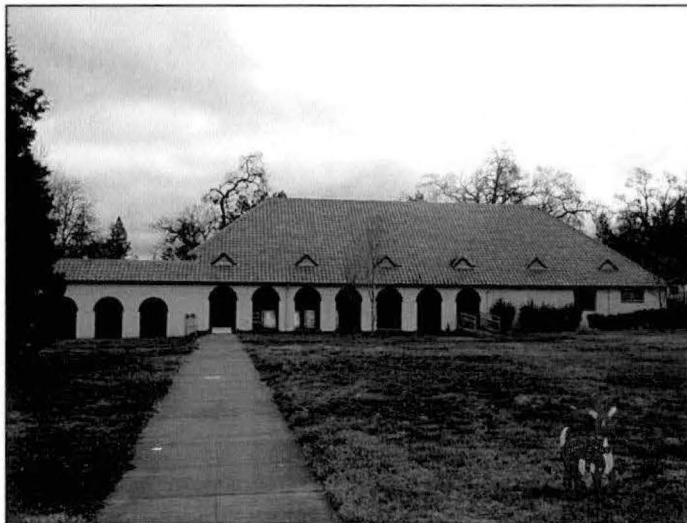
Photograph A.73. Looking southeast, showing the northwest elevation. The arcade that once faced the inner courtyard can be seen.
