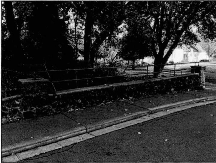
Photograph A.215. Looking east, showing the stone parapet and piers on the bridge's east elevation.
