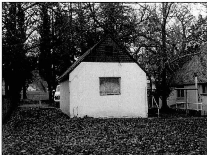
Photograph A.194. Looking southwest, showing the detached garage located to the south of the house.
