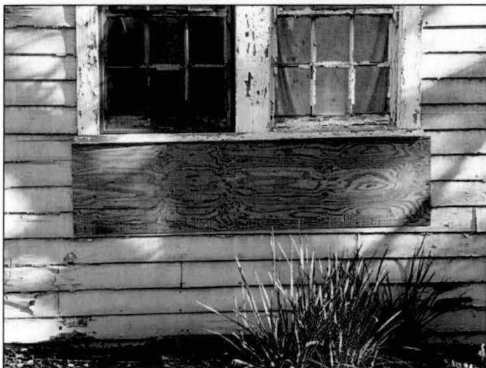
Photograph A.235. Wood board is affixed to the wood siding.
