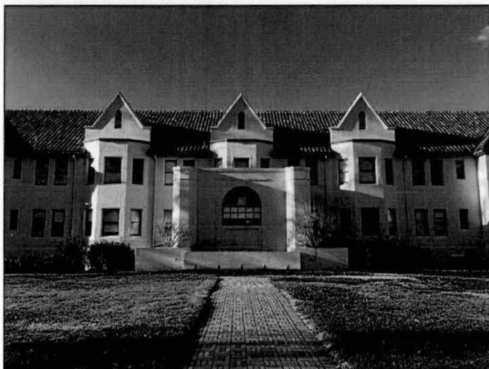
Photograph A.34. Looking northwest, showing the parapeted gables on the front, southeast elevation.
