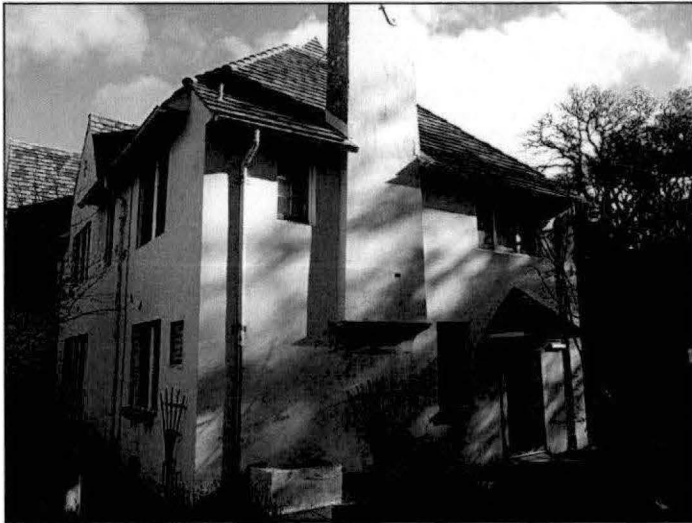
Photograph A.76. Looking east, showing the northwest and southwest elevations.
