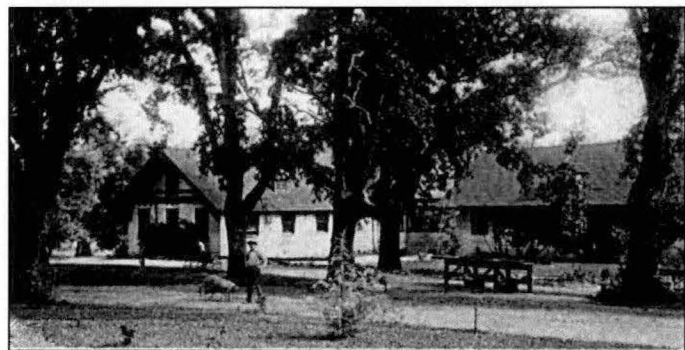
Photograph A.140. Ca.1915 historic photograph of Oak Lodge showing the gable of the west wing to the left, and the passthrough and rear wing to the right. 2
