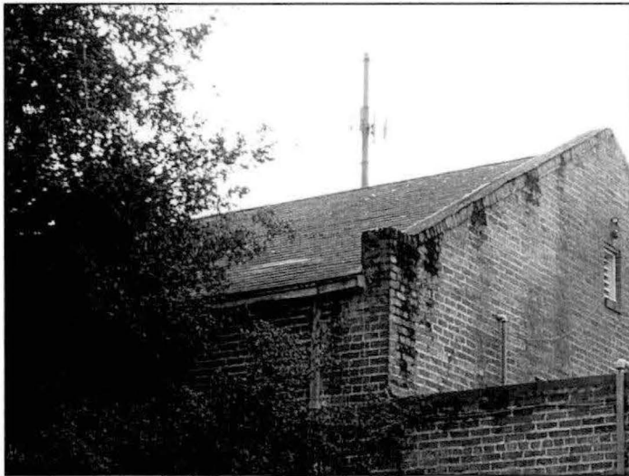
Photograph A.156. Minor biological growth on composition shingle roofing.
