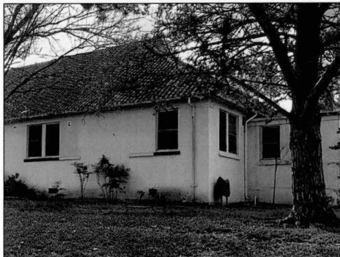
Photograph A.40. Looking south, showing the building's northern corner and the shed addition off the northwest elevation.
