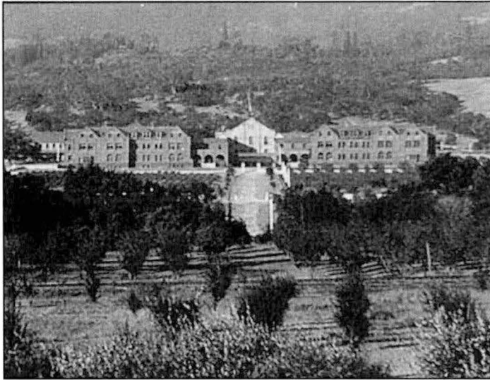
Photograph A.104. Ca.1900 historic photograph showing the Main Building and its two wings, Bentley and Judah Halls. The central core can be seen in this image, and shows this building form with its original two stories. 7
