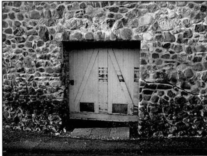
Photograph A.177. Looking southwest, showing the paneled wood batten double-doors on the ground level.
