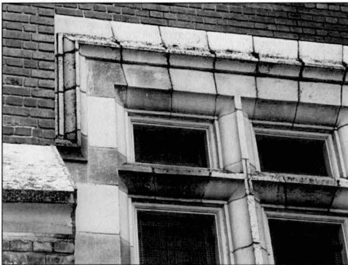
Photograph A.103. Detail of the terra cotta work that surrounds several of the building's windows.
