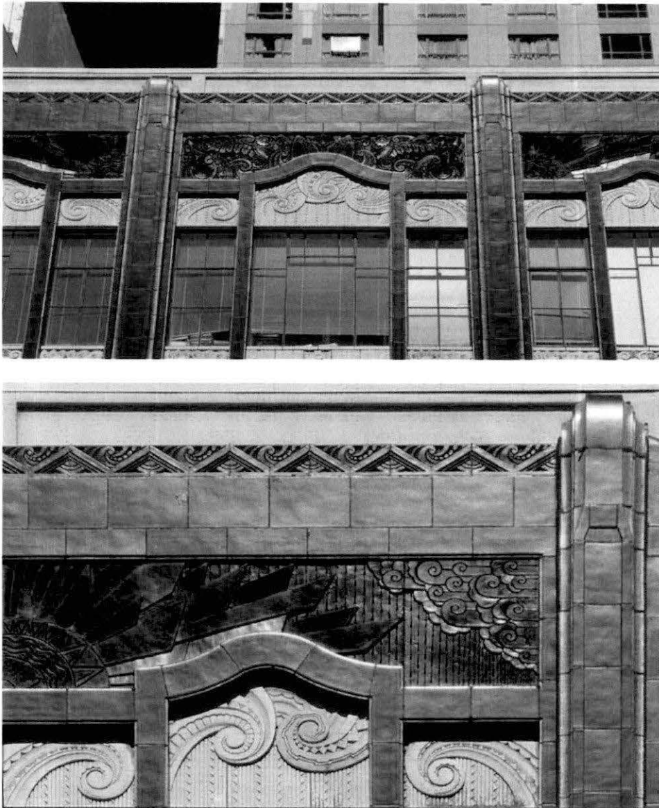
Fig. 13 Art Deco combined traditional spatial hierarchy and motifs with angularity of execution Top: Roof level spandrels and pilaster terminals From: "Building Oregon Collection, Digital Oregon," University of Oregon and Oregon State University Libraries, oregondigital.org/sets/building-or . Bottom: Jagged and swirling incised ornament From: "Building Oregon Collection, Digital Oregon," University of Oregon and Oregon State University Libraries, oregondigital.org/sets/building-or .
