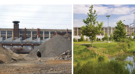
SALVATION ARMY KROC CORPS COMMUNITY CENTER, ANDROPOGON ASSOCIATES, 2010 Nearly all existing paving was reused on-site as crushed aggregate base and fill
