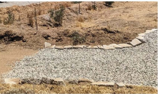
THE FOUNDATION WORKS, ACTON, CA
