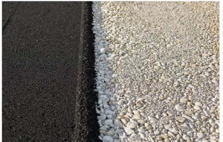
Crushed concrete aggregate as a base course for asphalt paving
