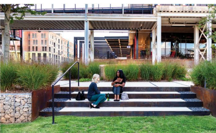
Former loading yard pavement is salvaged in rubble-filled gabions used at grade transitions and to define space throughout the site
