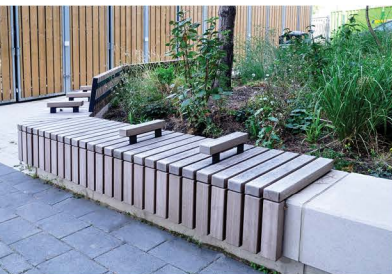
New wooden benchtops installed on concrete seat walls
