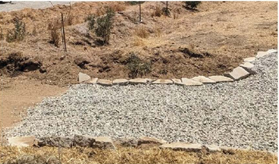
THE FOUNDATION WORKS, ACTON, CA
