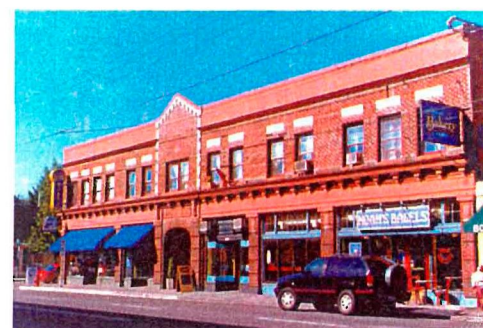
Ground floor retail with housing above.
