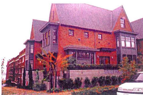
2-story corner unit.
