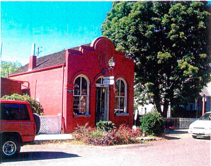
View of one-story commercial building
