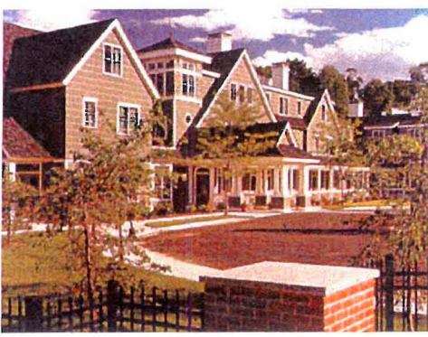
Primary entrance court.
