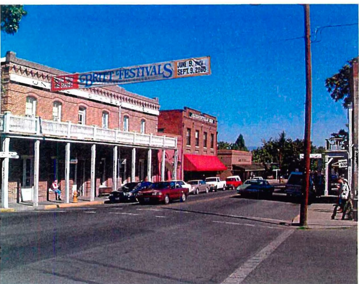
View of two-story building
