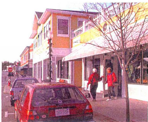
Ground floor retail with offices mixed with roof-deck above.
