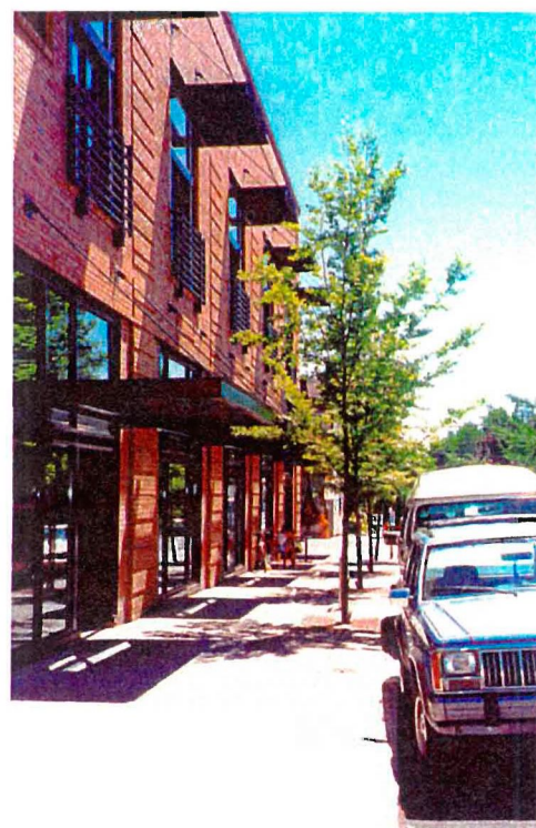
Awnings and shading devices help to articulate the building facade.
