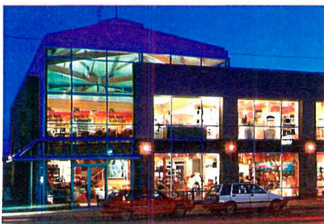
2-story with prominent entry corner.
