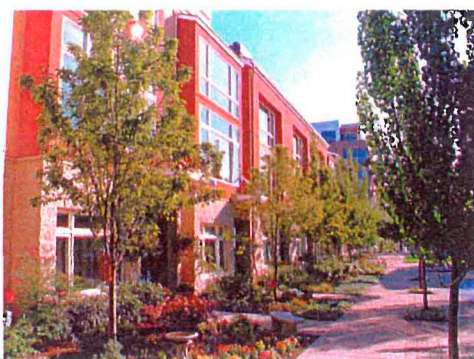
Ground floor entries are visible from the street and courtyard.
