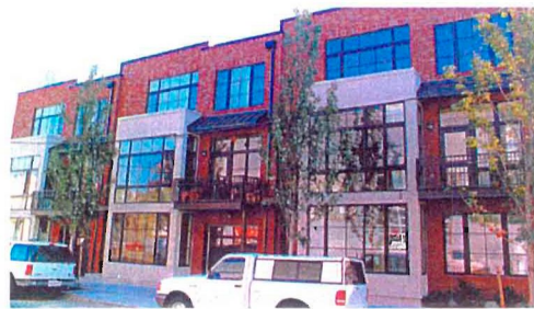
Varying building materials & elements create visual interest.
