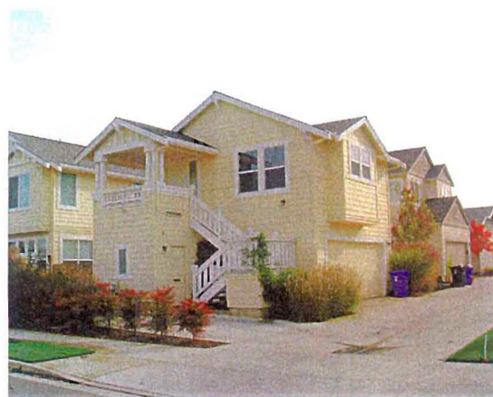
Accessory unit above alley loaded garage.
