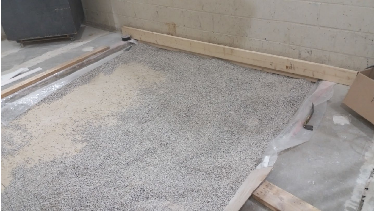
Figure 9 – Gravel partially installed over hemp board
