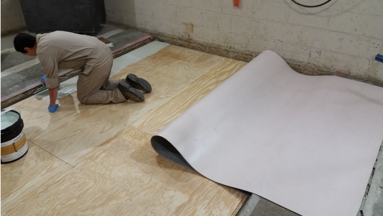
Figure 15 – Adhesive being troweled over plywood prior to installation of flooring
