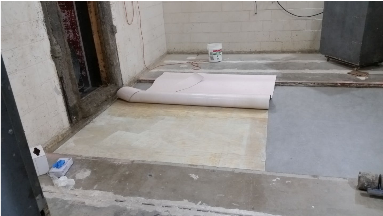
Figure 16 – Flooring partially installed
