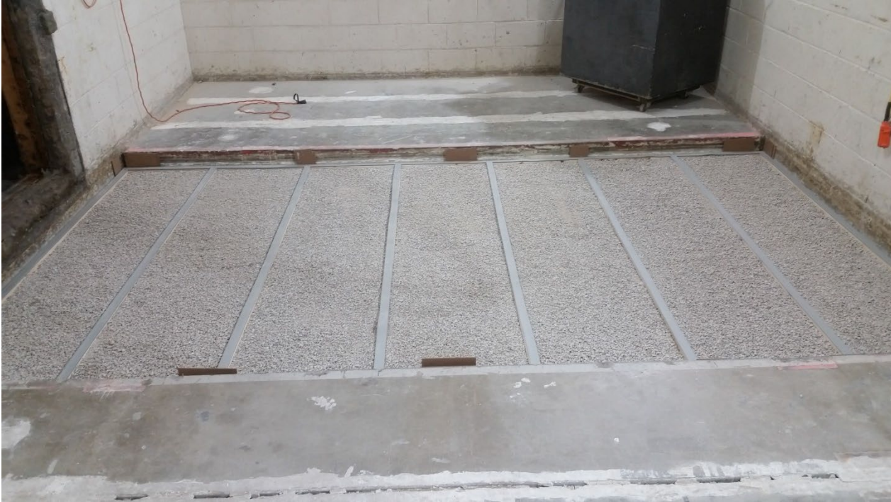
Figure 11 - Gravel and sleepers with Piano B 40/40 installed
