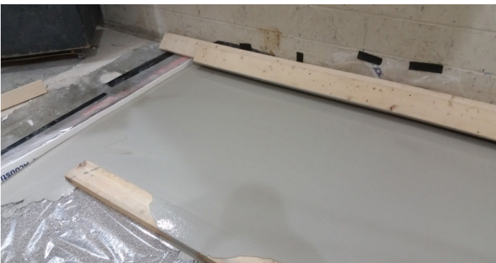
Figure 12 - Gypcrete partially installed over vapor barrier
