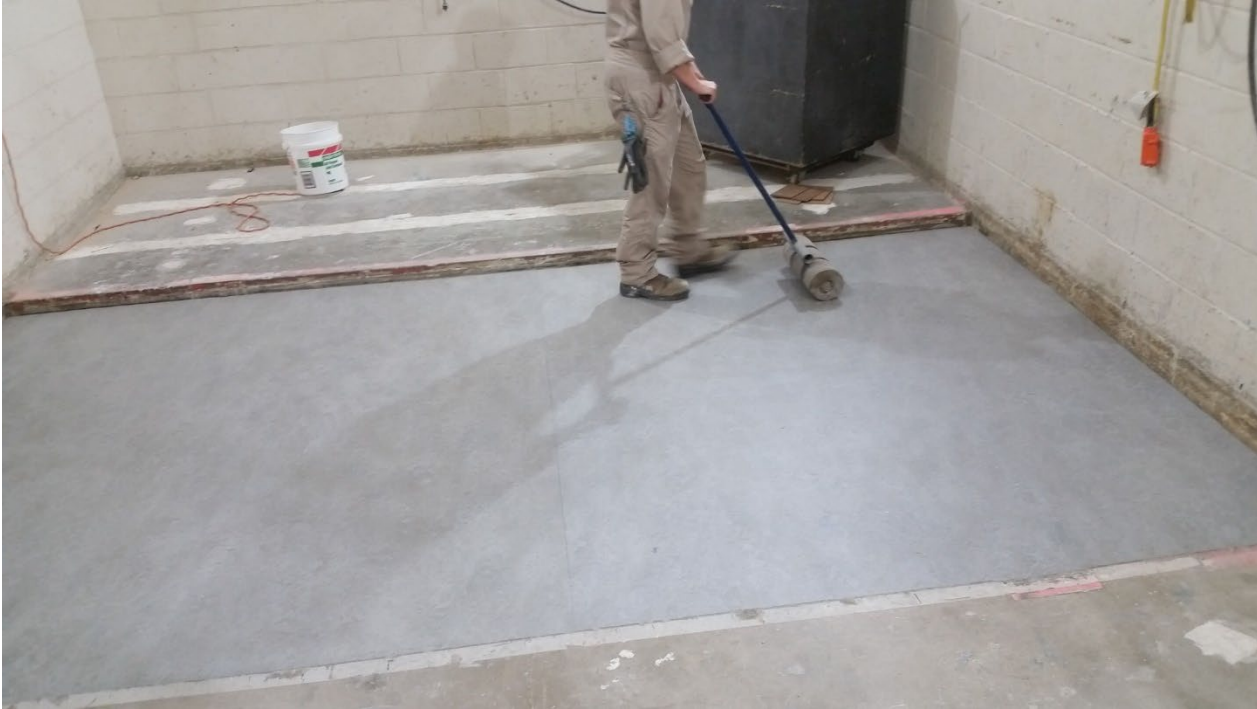
Figure 17 - Flooring partially installed
