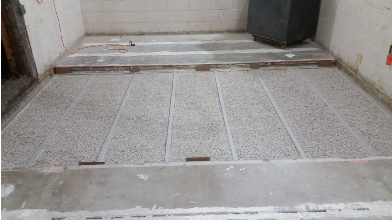
Figure 11 – Gravel and sleepers with Piano B 40/40 installed
