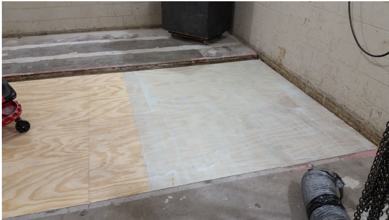
Figure 15 - Adhesive partially installed over plywood
