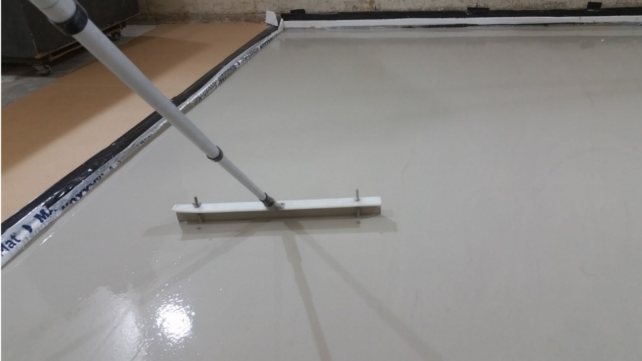
Figure 13 – Gypcrete installation
