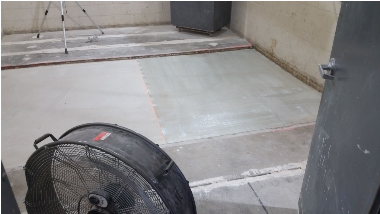
Figure 14 – Adhesive partially installed over gypcrete
