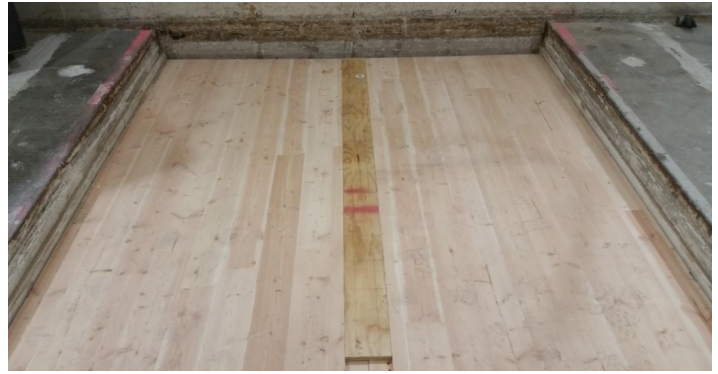
Figure 5 - 3/4" x 6" plywood spline partially installed over CLT rabbets
