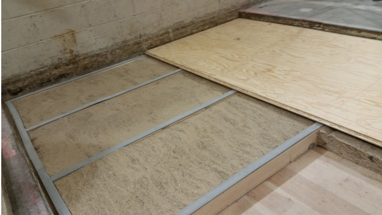
Figure 11 – Hemp boards partially installed between sleepers, plywood partially installed over sleepers
