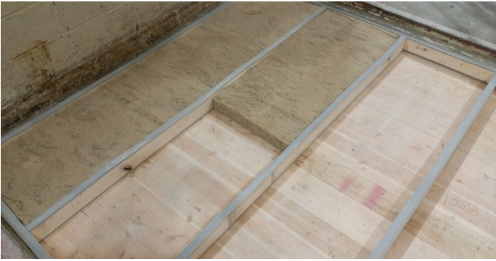
Figure 10 - Hemp boards partially installed between sleepers
