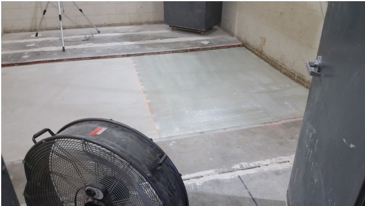
Figure 14 - Adhesive partially installed over gypcrete
