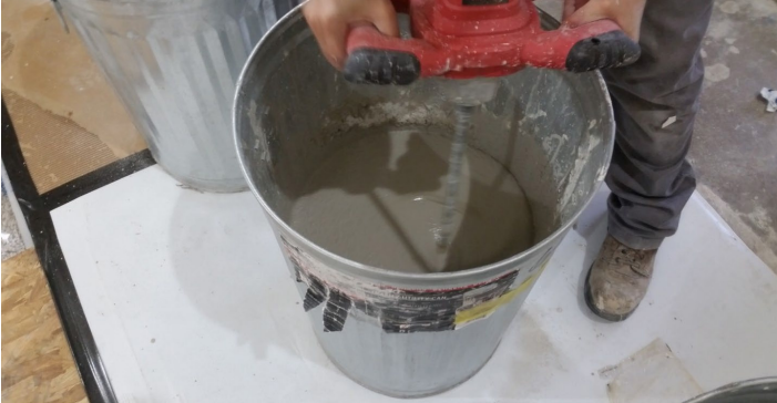
Figure 11 - Gypcrete mixing prior to pouring
