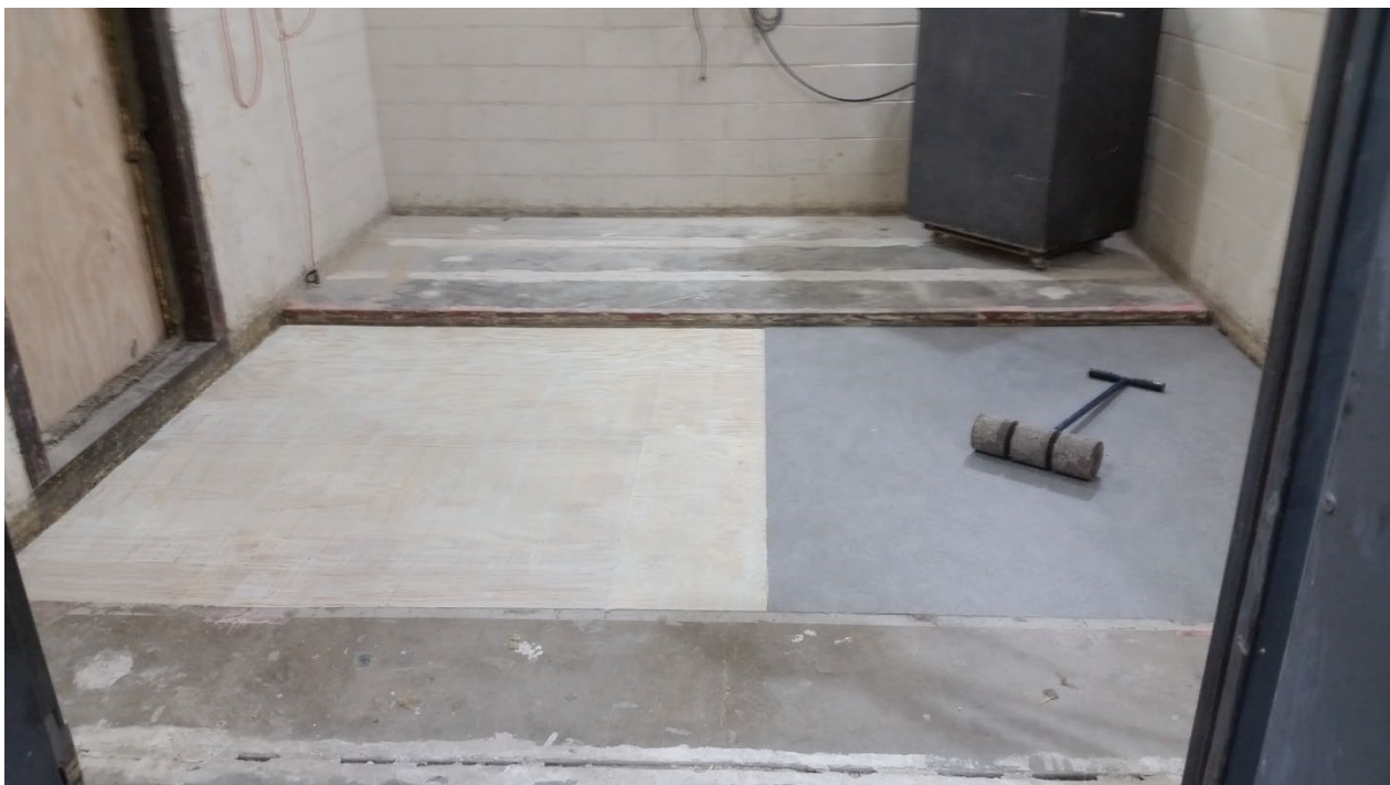
Figure 14 – Flooring partially installed over adhesive
