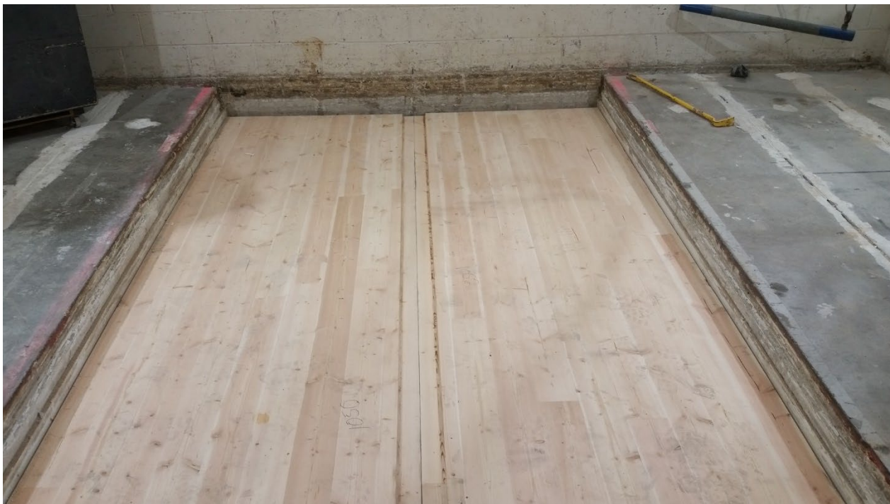
Figure 4 - CLT installed in test aperture
