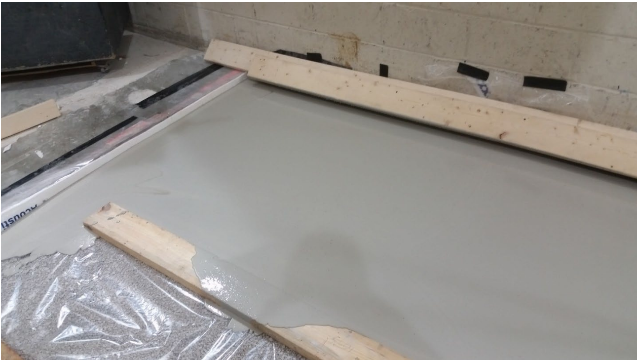
Figure 12 - Gypcrete partially installed over vapor barrier
