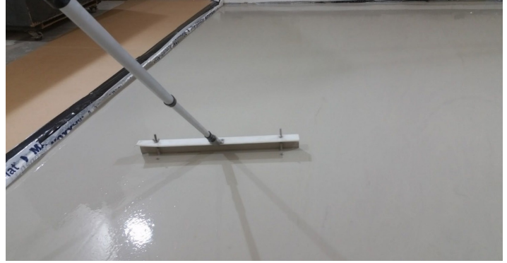
Figure 13 - Gypcrete installation
