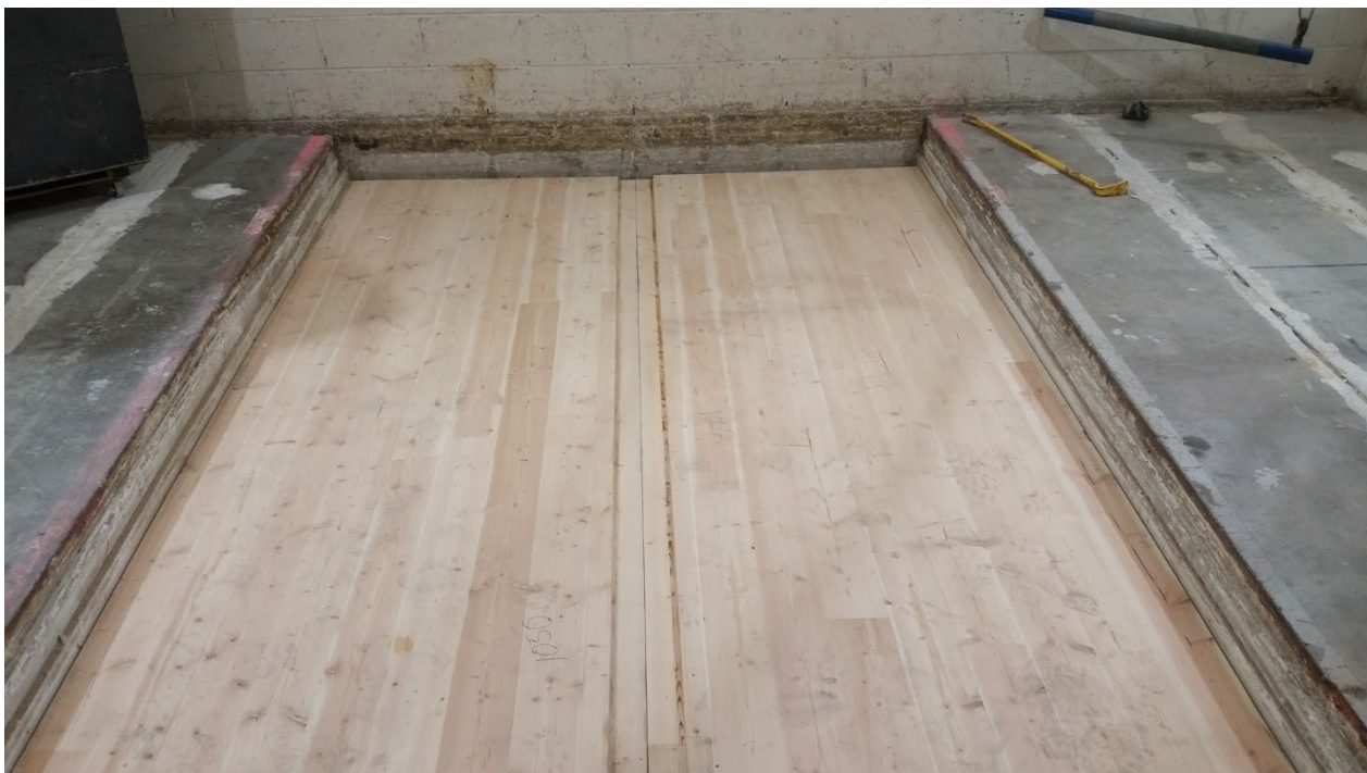
Figure 4 – CLT installed in test aperture
