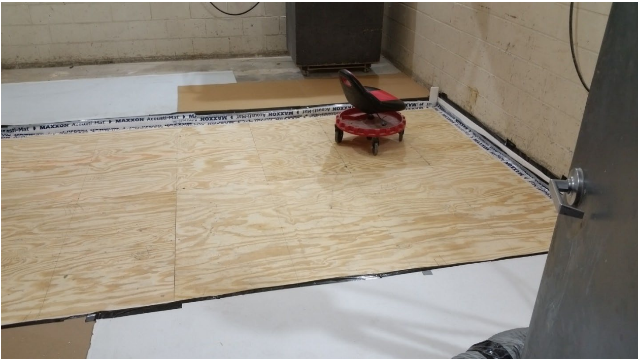
Figure 12 – Plywood subfloor installed
