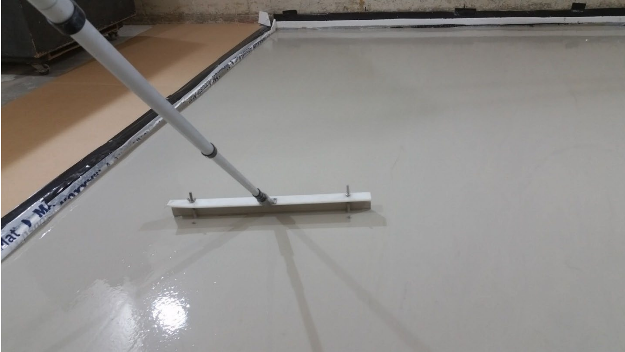
Figure 13 - Gycrete installation
