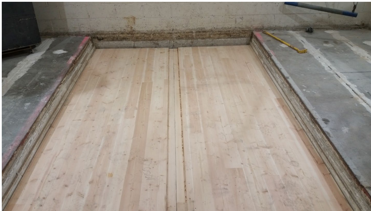
Figure 4 - CLT installed in test aperture
