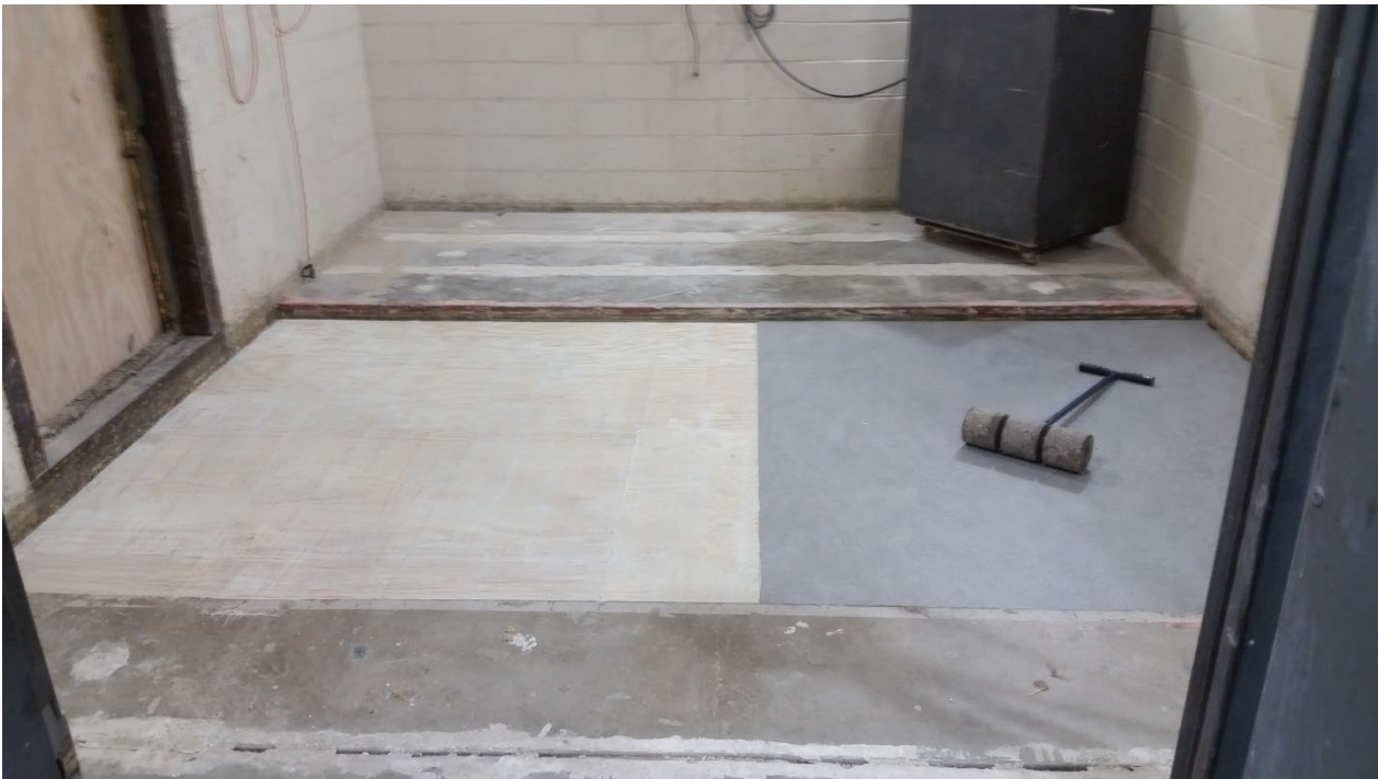
Figure 14 - Flooring partially installed over adhesive
