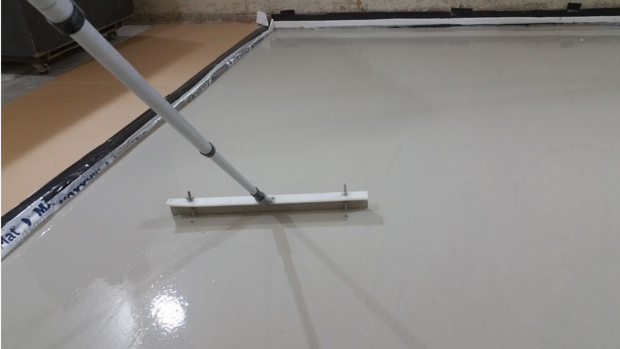
Figure 13 – Gypcrete installation
