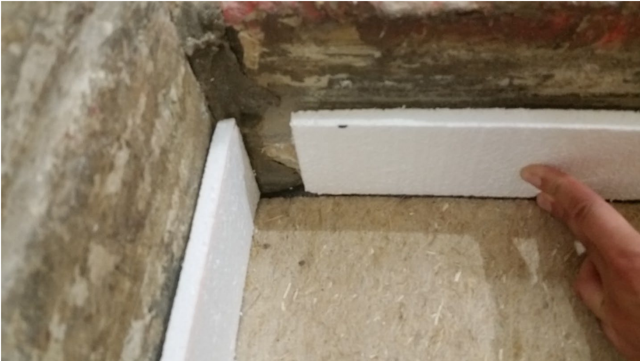
Figure 8 – Polystyrene used as an isolation around the perimeter prior to installation of gravel
