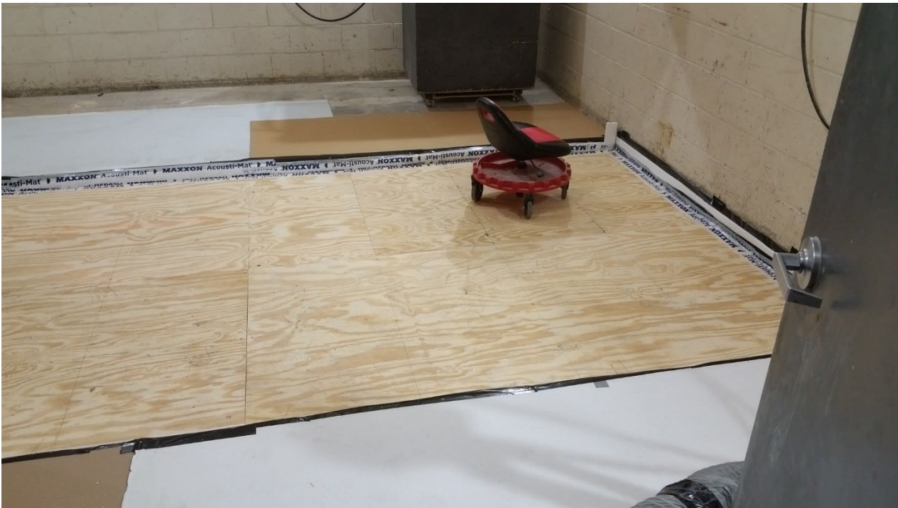
Figure 12 - Plywood subfloor installed
