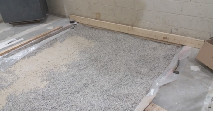
Figure 9 - Gravel partially installed over hemp board
