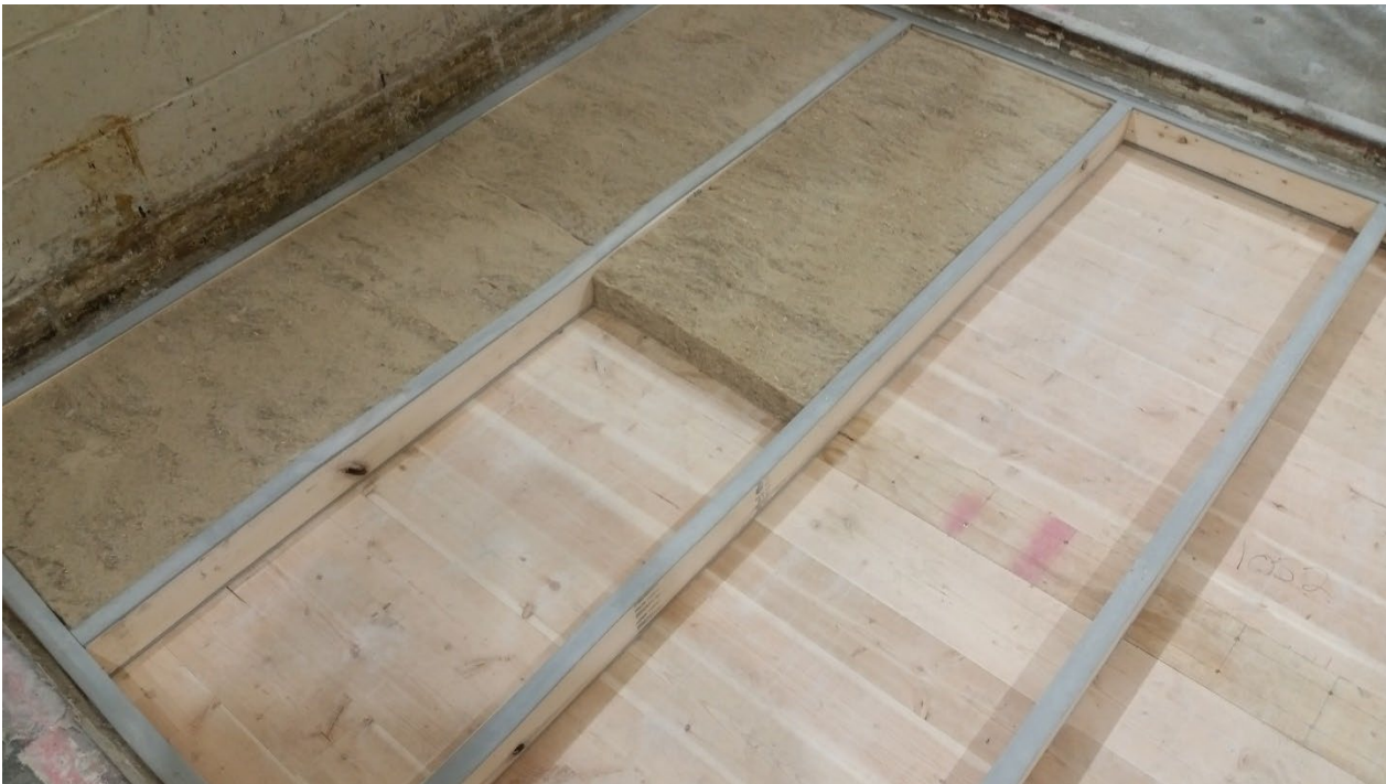
Figure 10 - Hemp boards partially installed between sleepers
