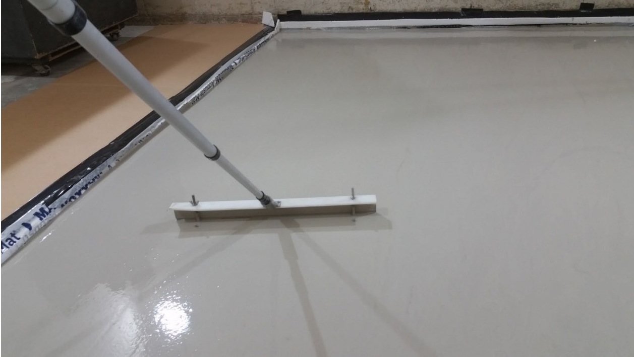
Figure 13 - Gypcrete installation
