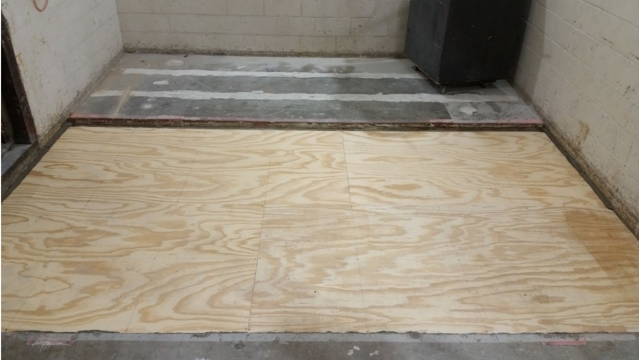
Figure 13 – Plywood subfloor installed
