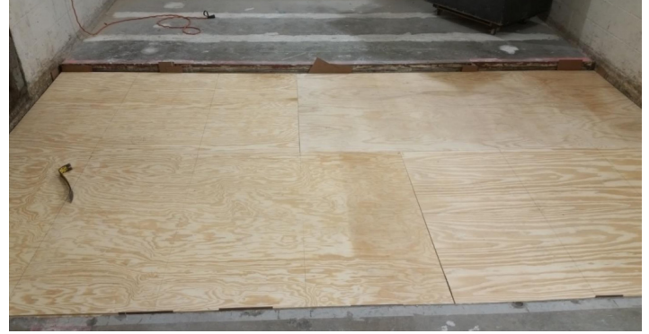
Figure 13 - Plywood subfloor installed
