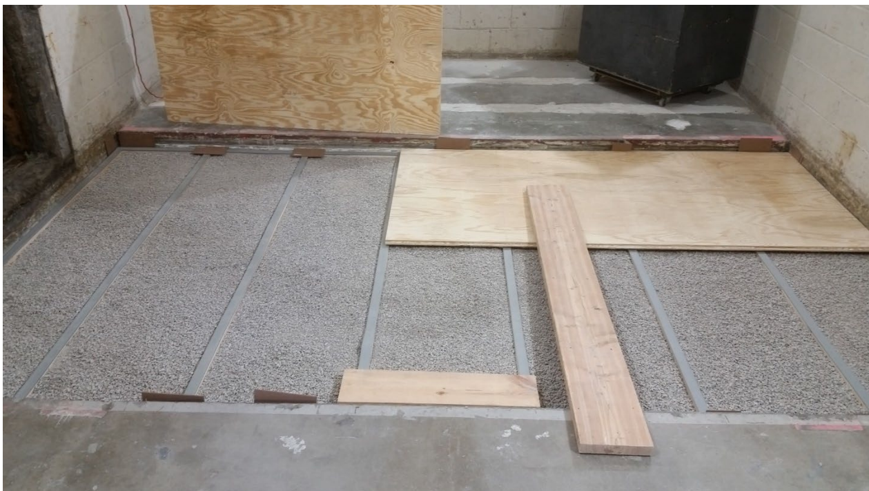
Figure 12 – Plywood subfloor partially installed
