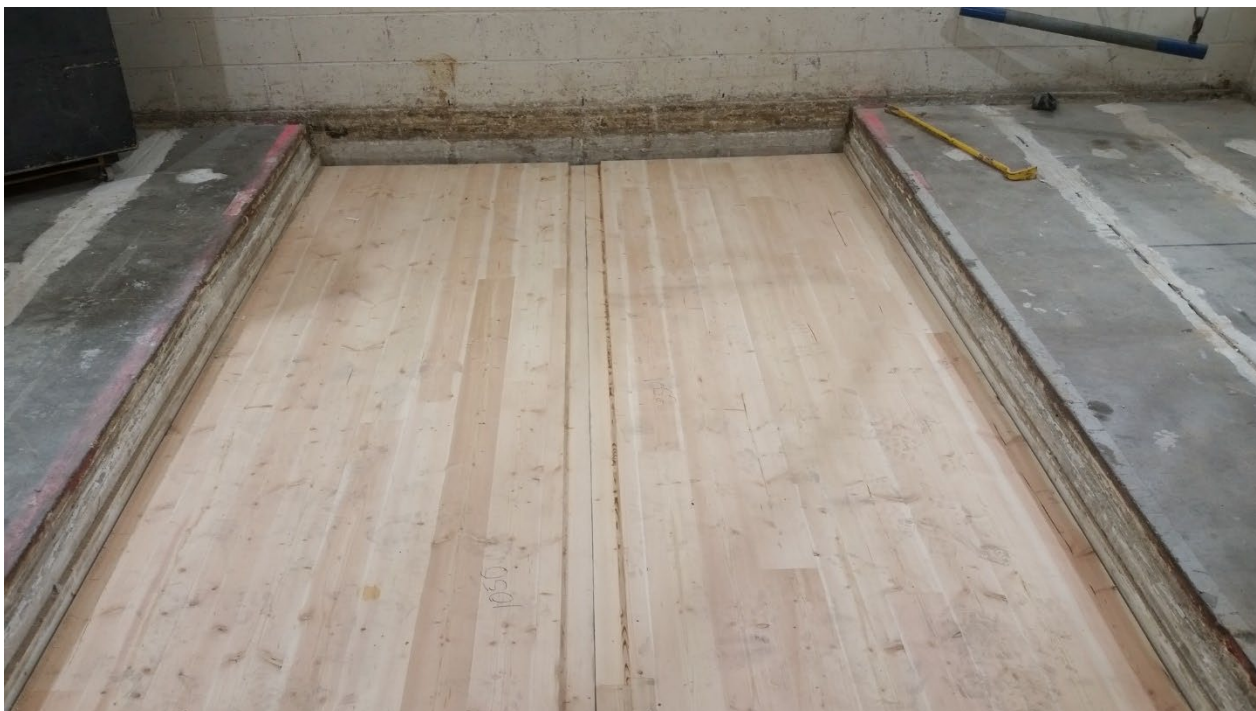
Figure 4 – CLT installed in test aperture
