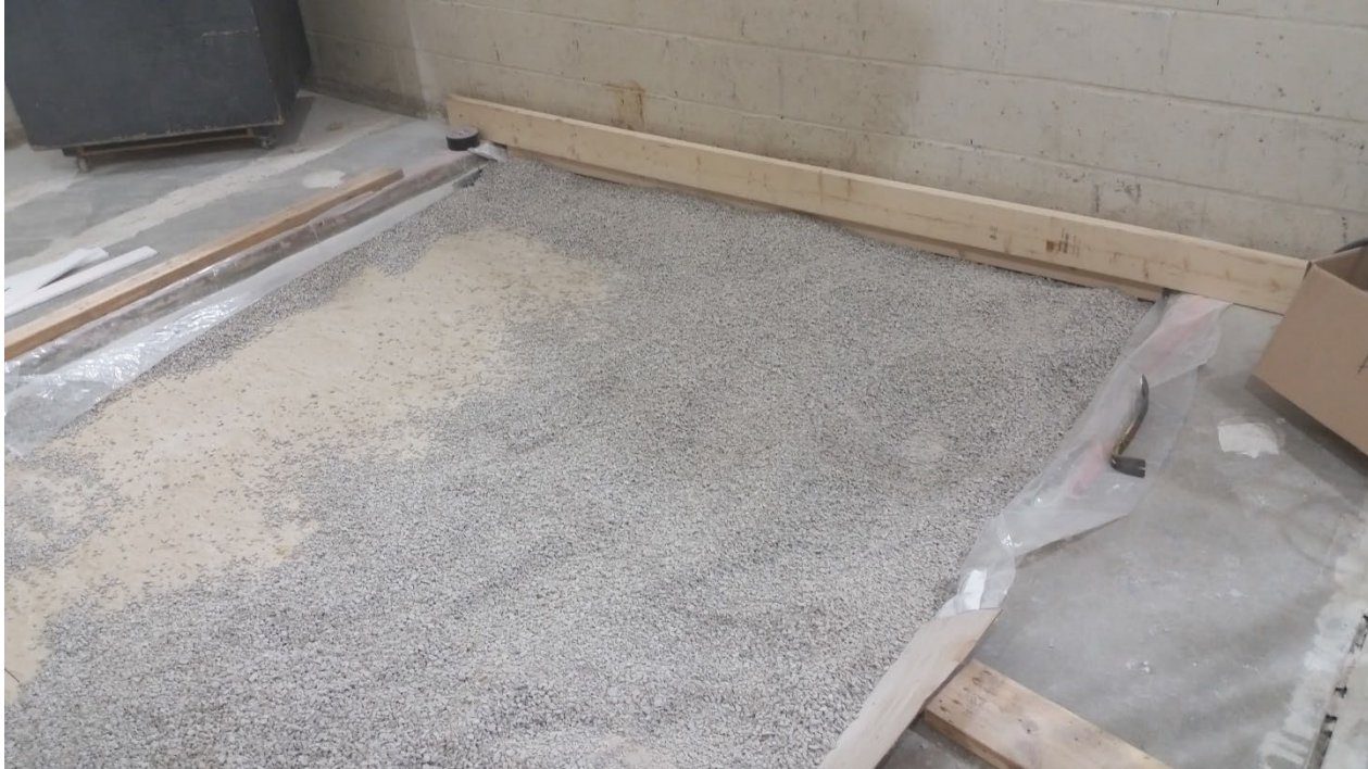
Figure 9 – Gravel partially installed over hemp board
