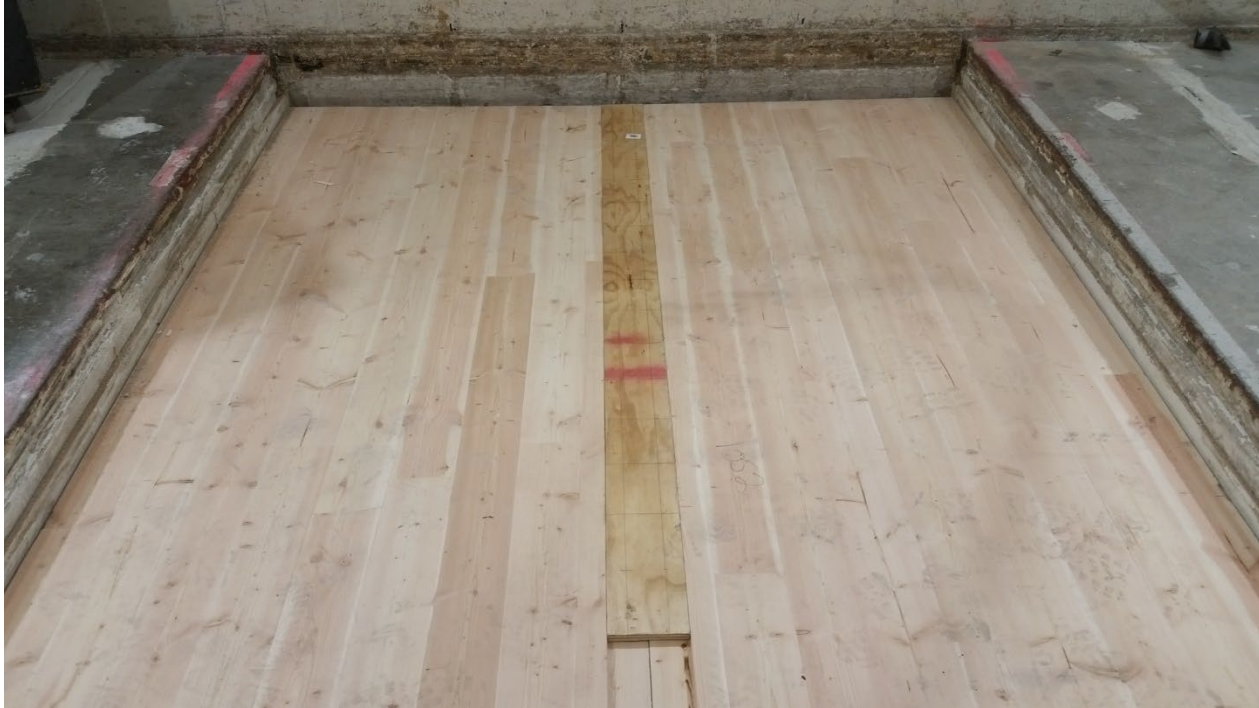
Figure 5 – 3/4” x 6” plywood spline partially installed over CLT rabbets
