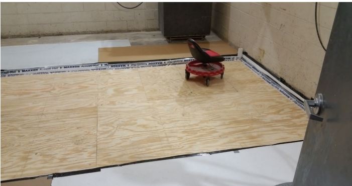
Figure 12 - Plywood subfloor partially installed
