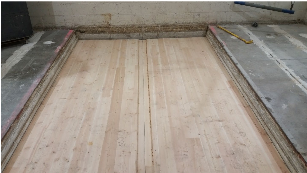
Figure 4 - CLT installed in test aperture
