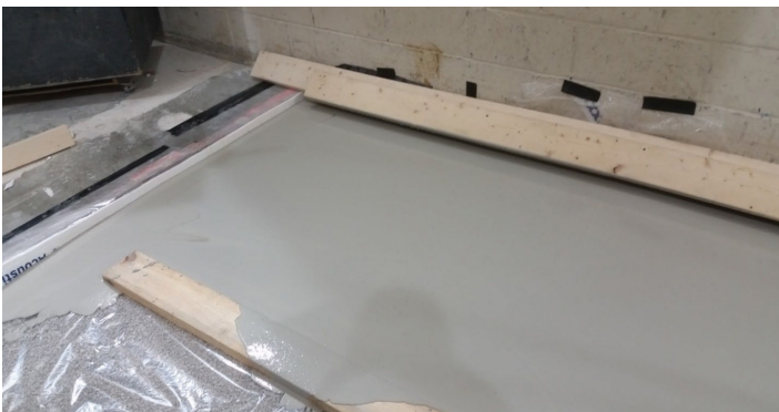
Figure 12 - Gypcrete partially installed over vapor barrier
