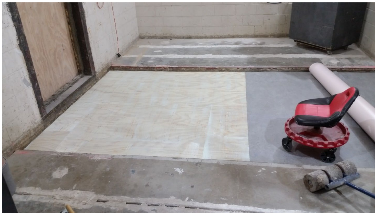
Figure 16 - Flooring partially installed over adhesive
