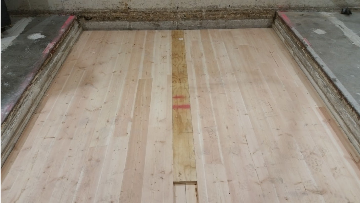
Figure 5 - 3/4" x 6" plywood spline partially installed over CLT rabbets
