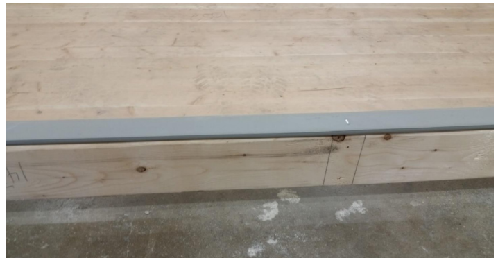
Figure 8 - Piano B 40/40 strip fastened to sleeper prior to installation of sleeper
