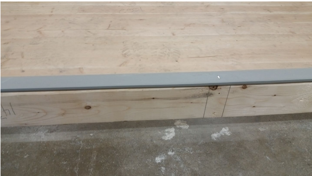
Figure 8 - Piano B 40/40 strip fastened to sleeper prior to installation of sleeper
