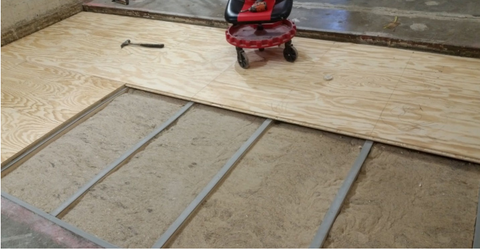
Figure 11 - Hemp boards installed between sleepers, plywood partially installed over sleepers
