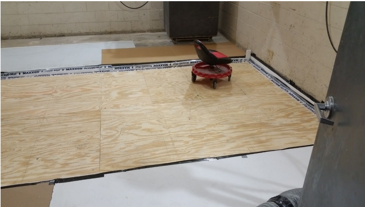
Figure 12 - Plywood subfloor installed
