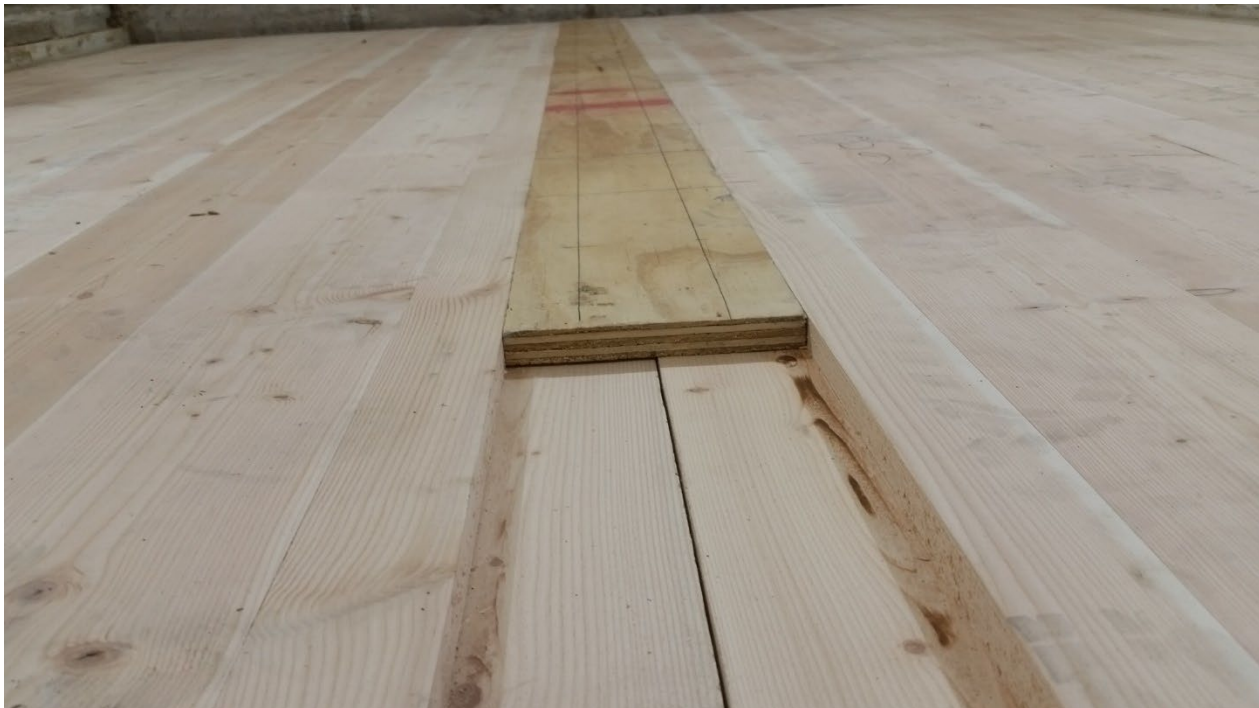
Figure 6 – Detail of 3/4” x 6” plywood spline partially installed over CLT rabbets
