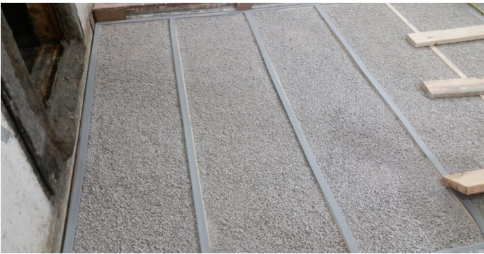
Figure 10 - Gravel installed; Piano B 40/40 partially installed to top of sleepers
