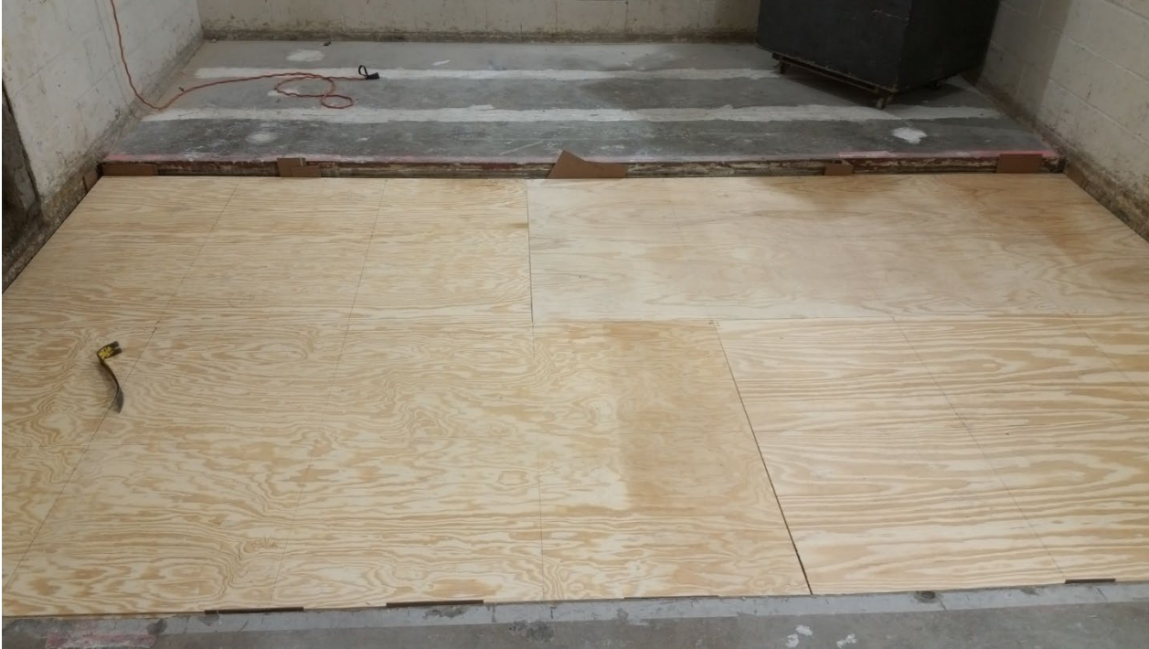
Figure 13 – Plywood subfloor installed
