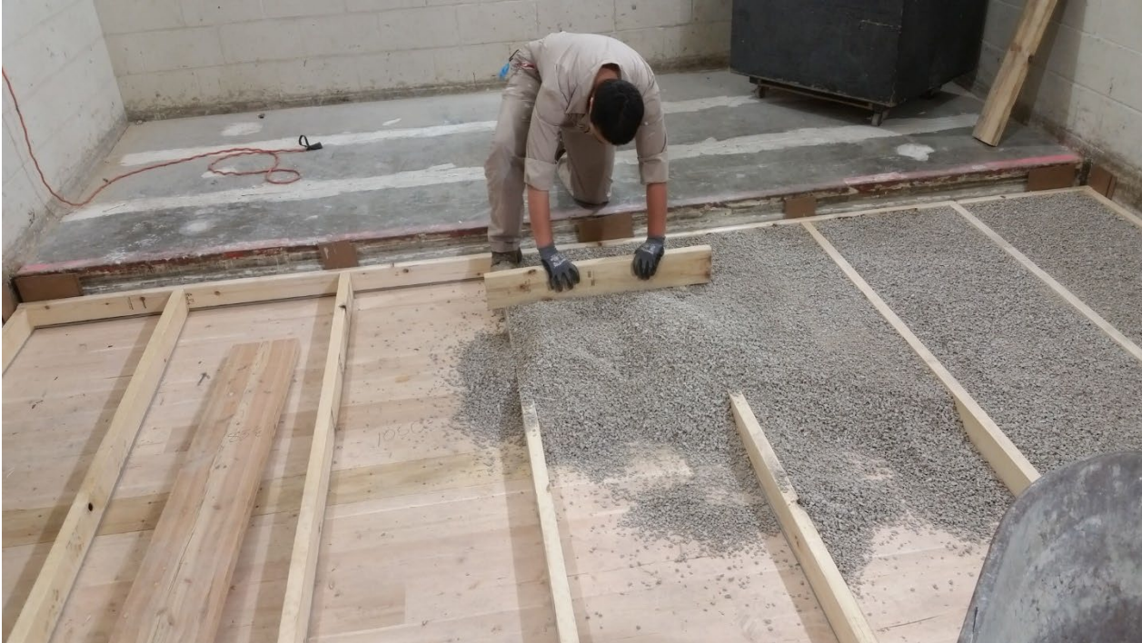
Figure 9 – Gravel partially installed in gaps between sleepers
