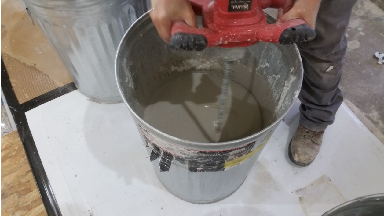
Figure 11 - Gypcrete mixing prior to pouring
