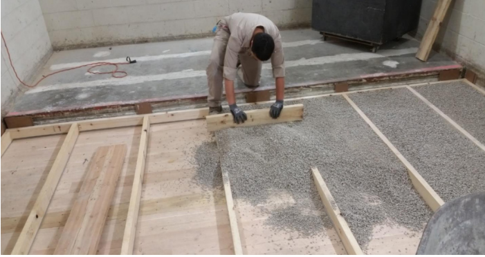
Figure 9 - Gravel partially installed in gaps between sleepers
