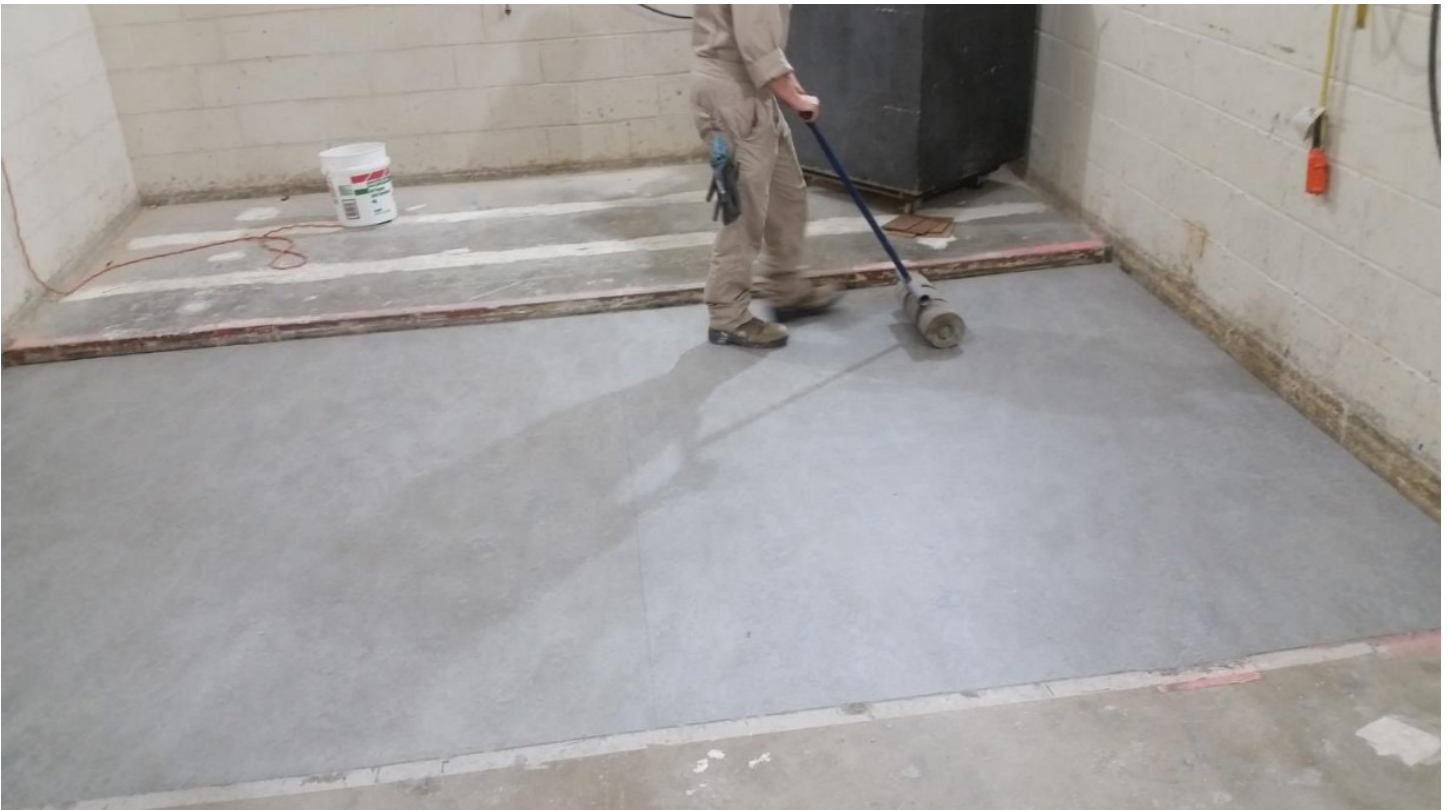
Figure 8 - F03 Assembly - Flooring partially installed (from above)
