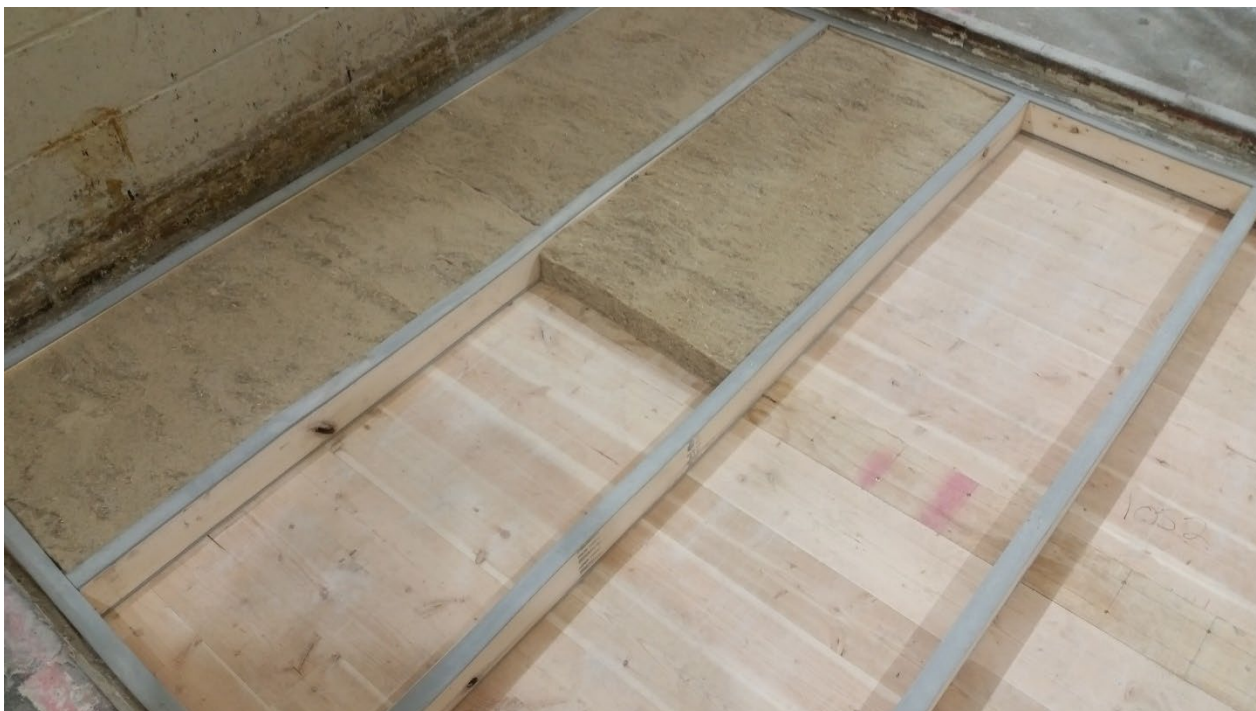
Figure 10 – Hemp boards partially installed between sleepers
