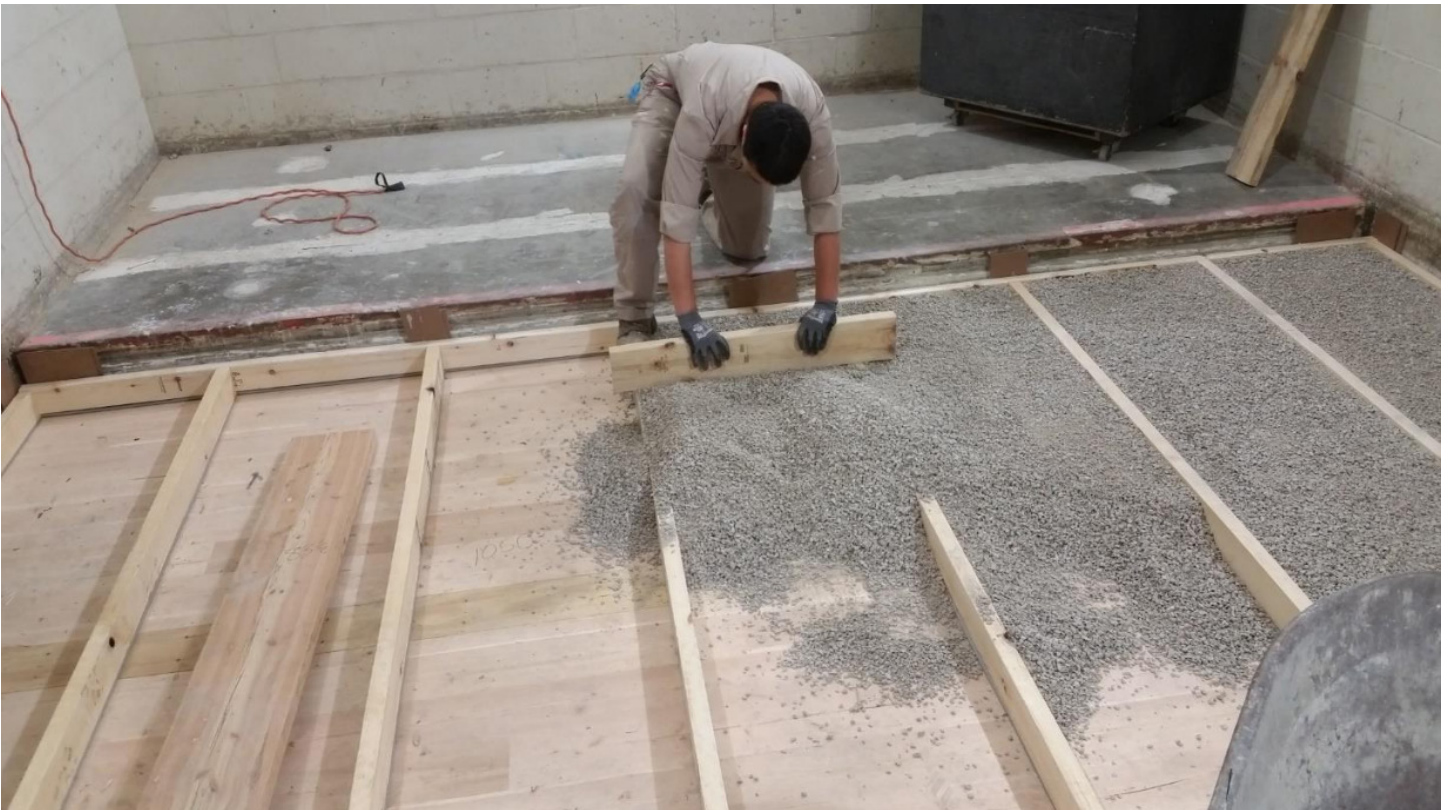
Figure 4 - F03 Assembly - Gravel partially installed in gaps between sleepers (from above)
