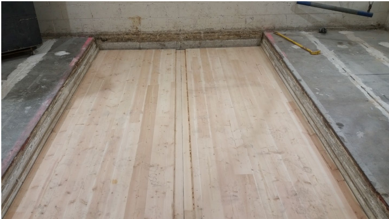
Figure 4 - CLT installed in test aperture
