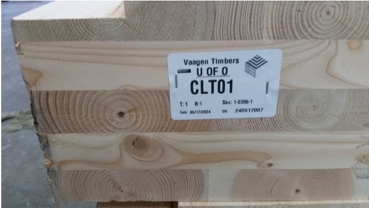
Figure 3 - CLT (1 of 2) prior to installation
