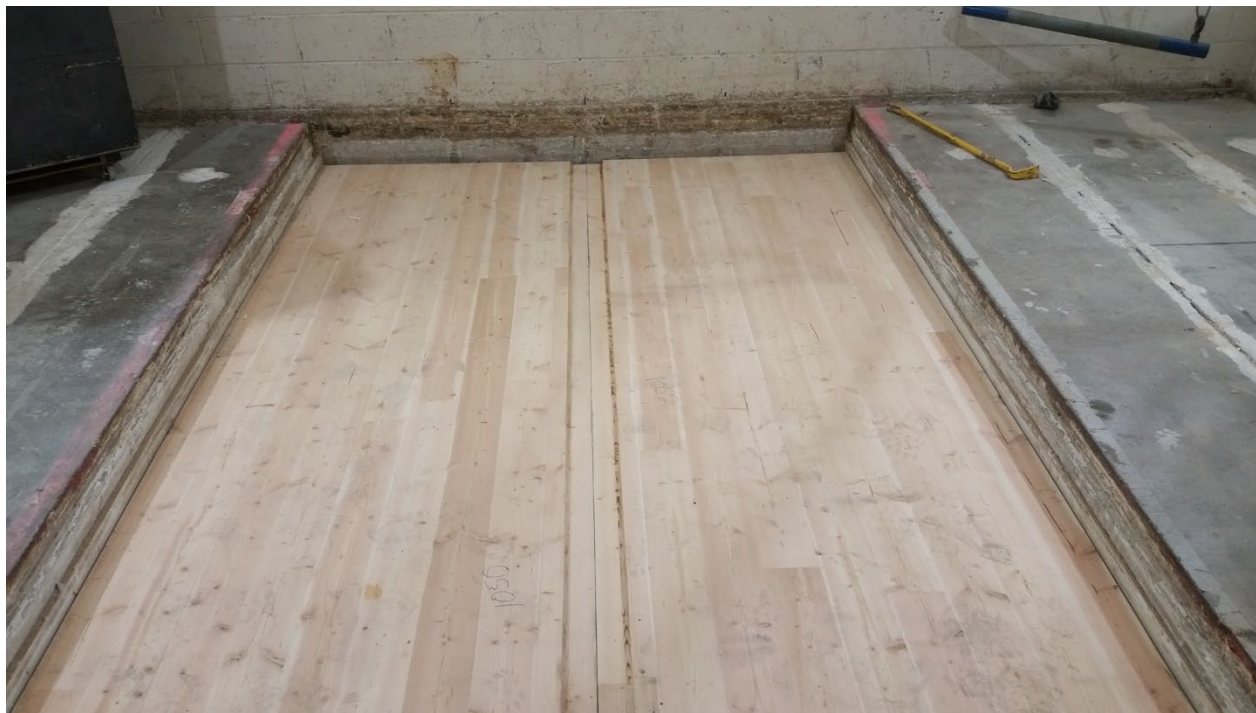
Figure 4 - CLT installed in test aperture
