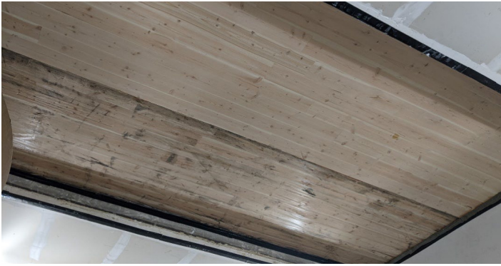
Figure 2 - Specimen mounted in test aperture, as viewed from receive room
