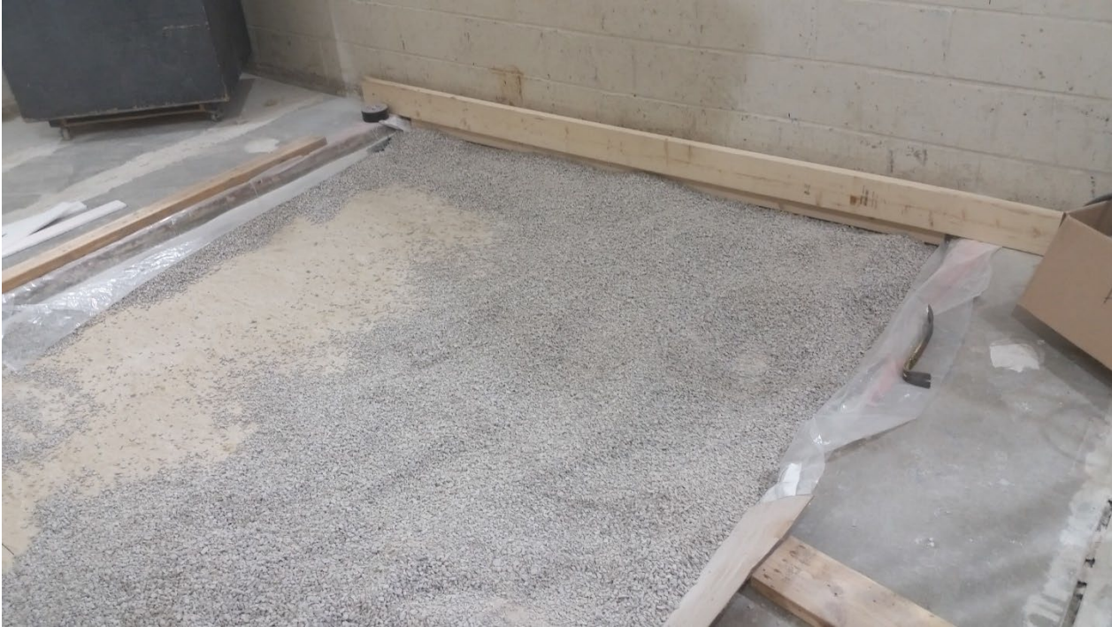
Figure 9 - Gravel partially installed over hemp board
