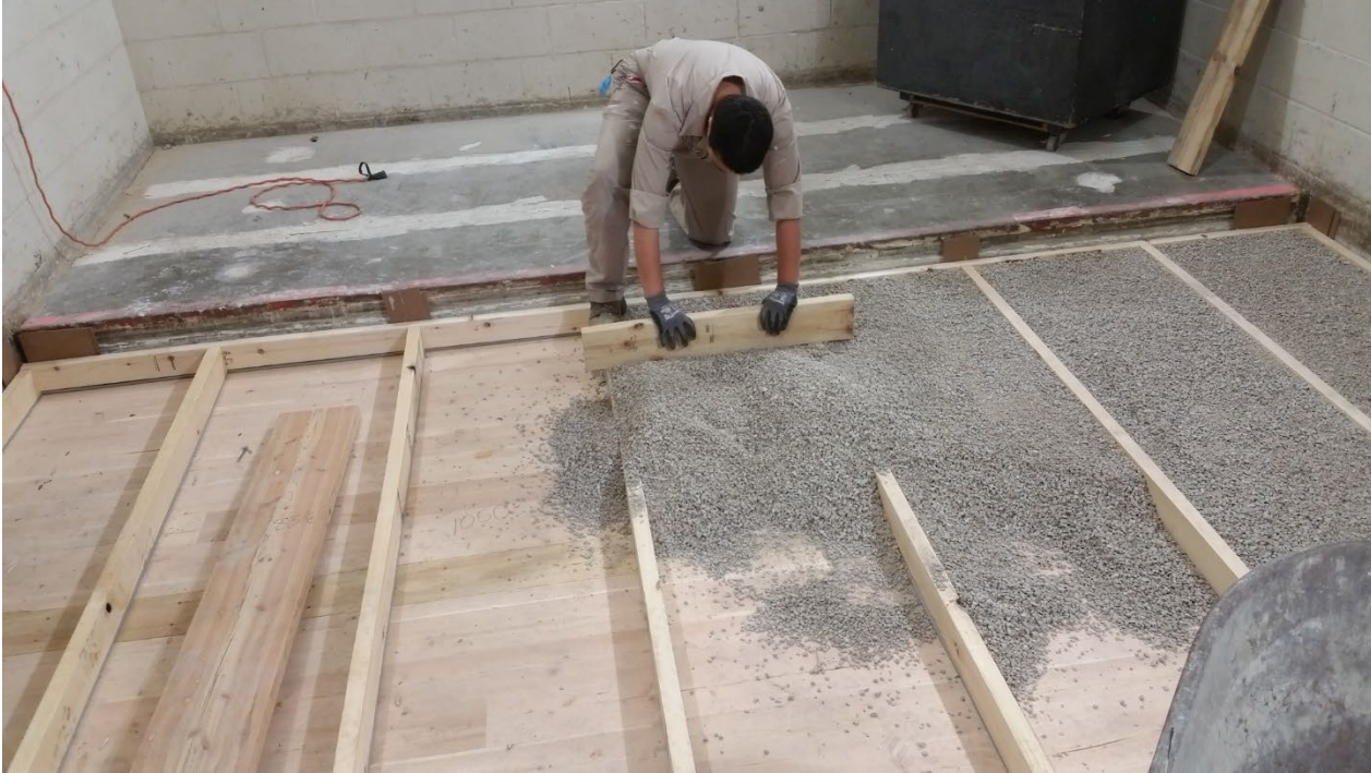
Figure 9 - Gravel partially installed in gaps between sleepers
