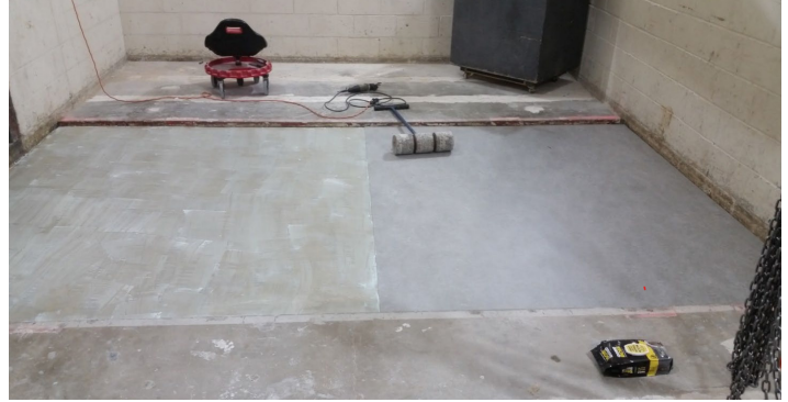
Figure 15 - Adhesive installed over gypcrete, flooring partially installed over adhesive
