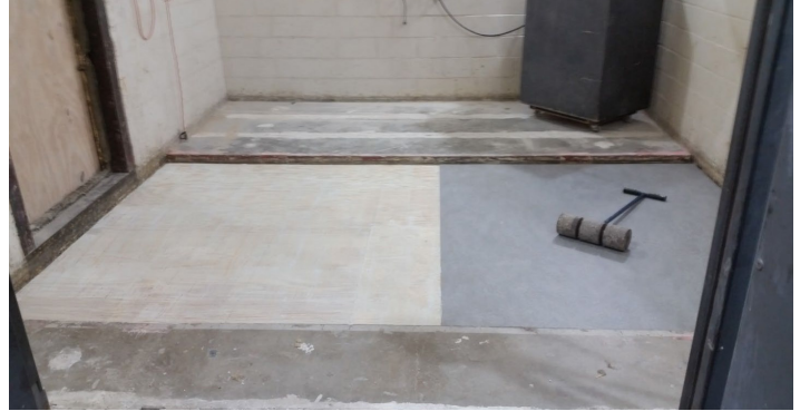
Figure 14 - Flooring partially installed over adhesive
