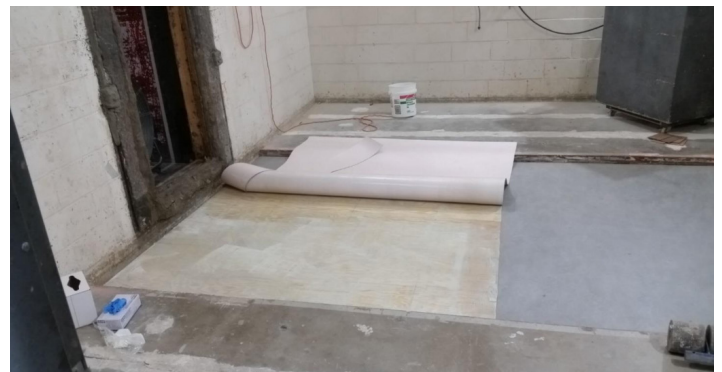
Figure 16 - Flooring partially installed
