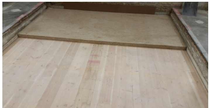
Figure 7 - Hemp board partially installed over CLT
