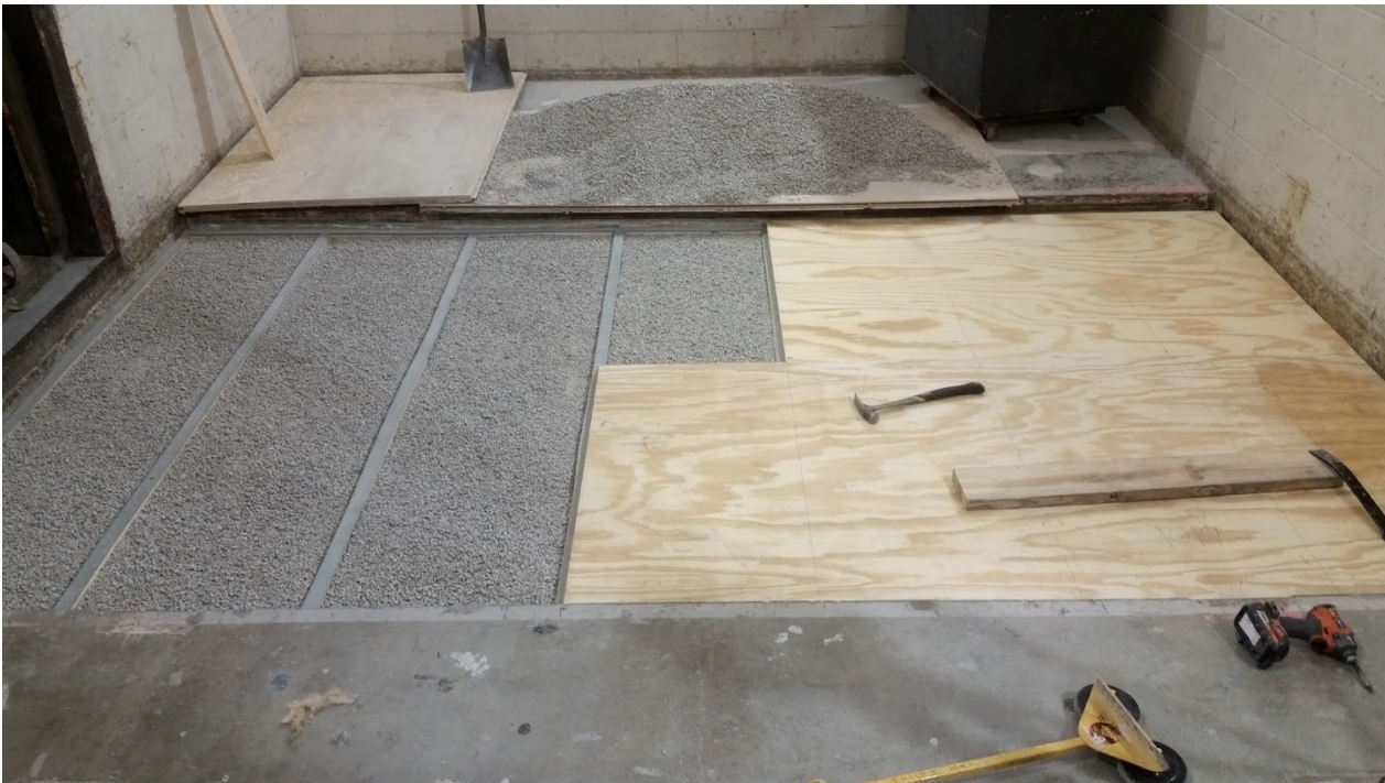
Figure 12 - Plywood subfloor partially installed
