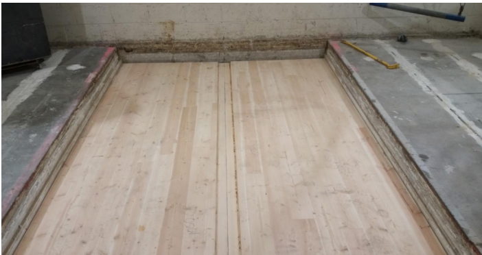
Figure 4 - CLT installed in test aperture
