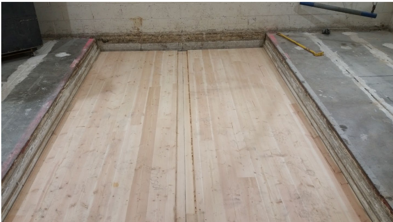
Figure 4 - CLT installed in test aperture
