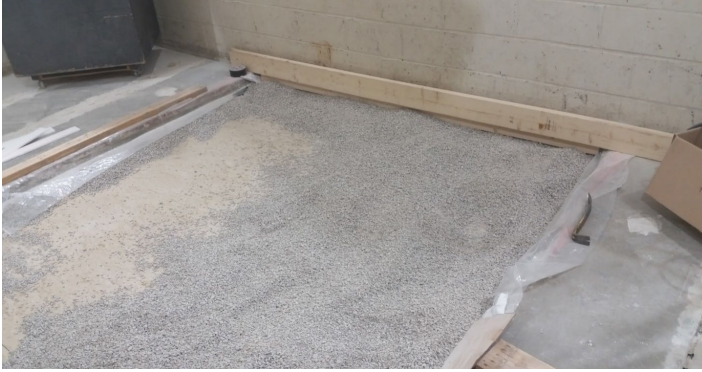
Figure 9 - Gravel partially installed over hemp board
