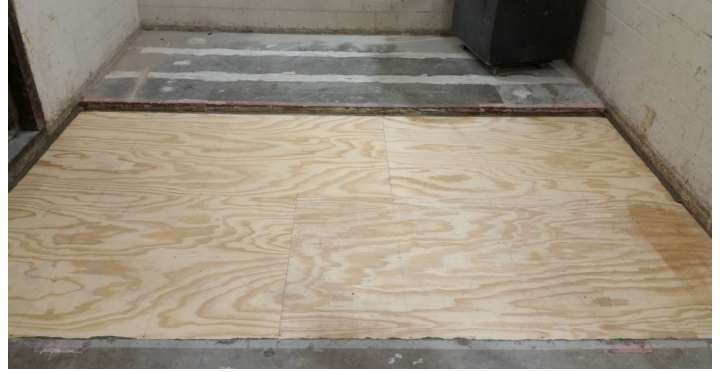
Figure 13 - Plywood subfloor installed
