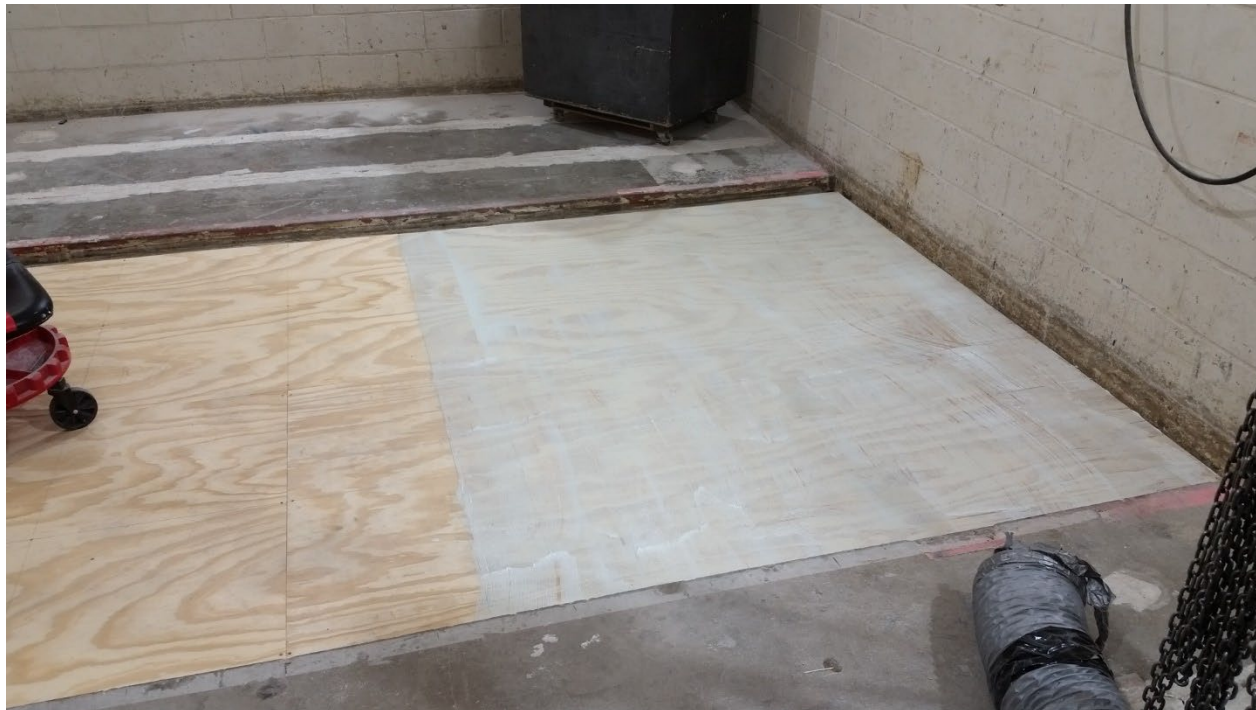
Figure 15 – Adhesive partially installed over plywood
