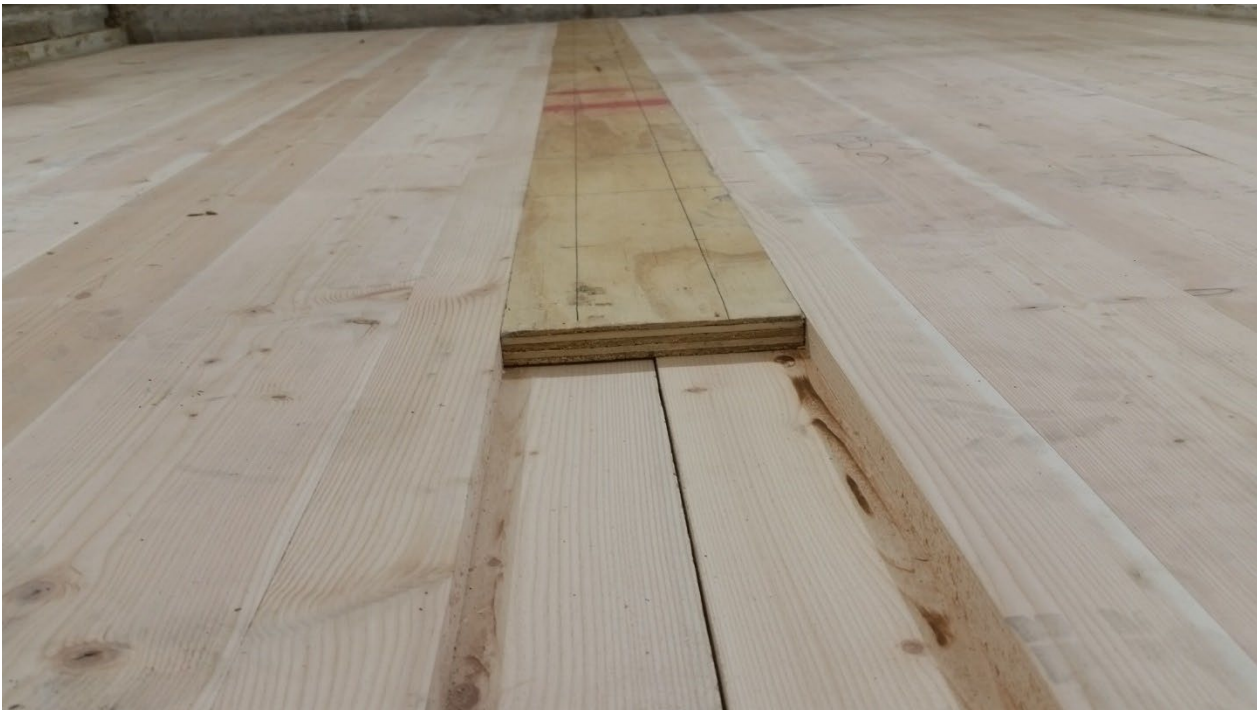
Figure 6 – Detail of 3/4” x 6” plywood spline partially installed over CLT rabbets
