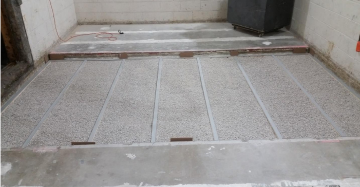
Figure 11 - Gravel and sleepers with Piano B 40/40 installed
