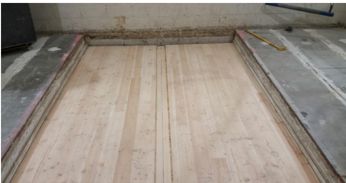
Figure 4 - CLT installed in test aperture
