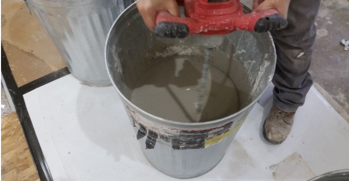
Figure 11 - Gypcrete mixing prior to pouring
