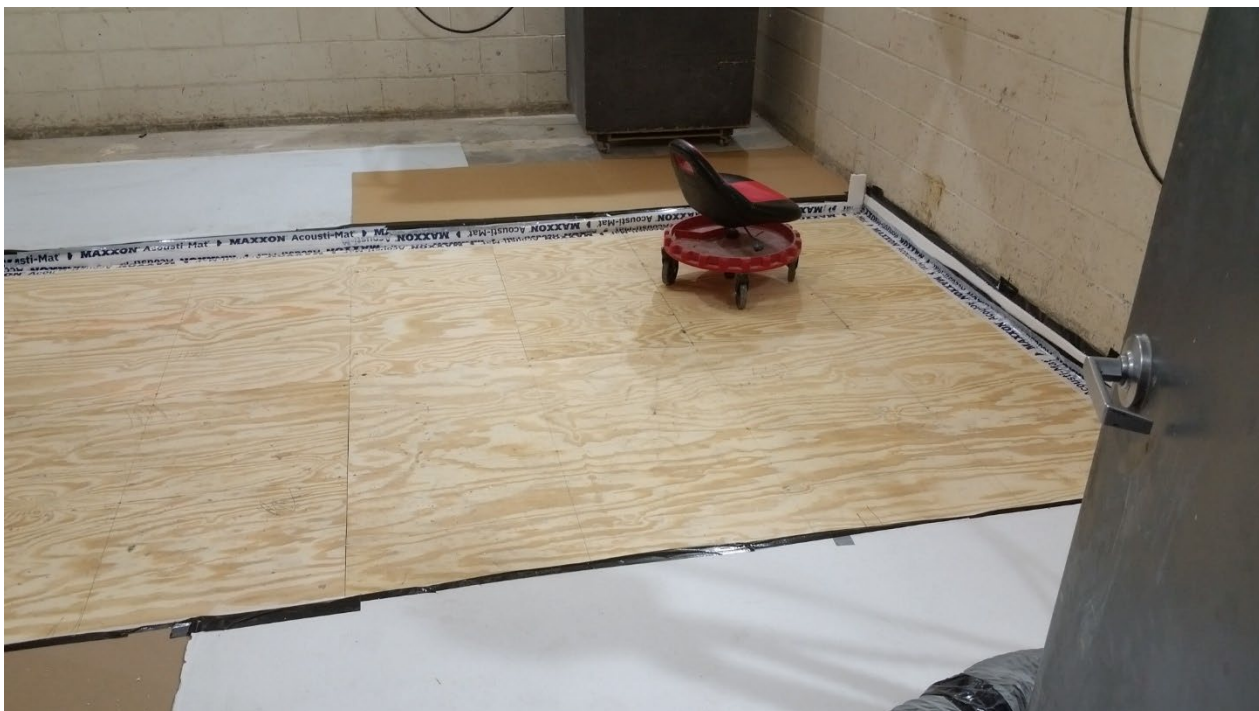
Figure 12 – Plywood subfloor installed
