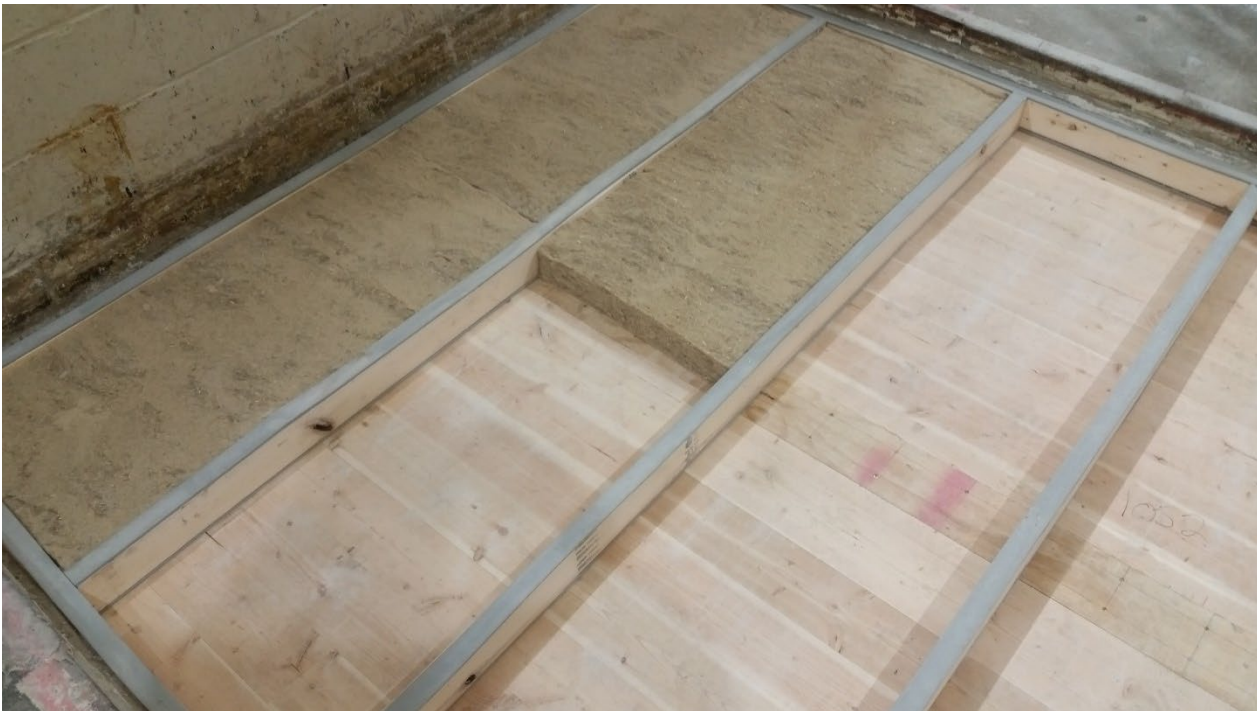
Figure 10 - Hemp boards partially installed between sleepers
