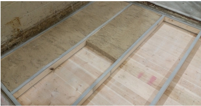
Figure 10 - Hemp boards partially installed between sleepers
