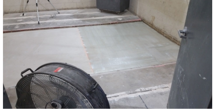
Figure 14 - Adhesive partially installed over gypcrete
