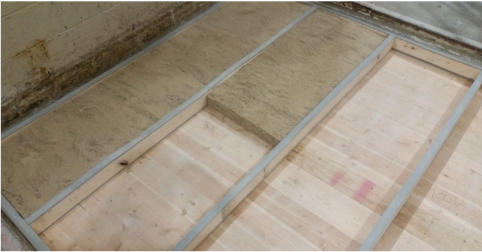
Figure 10 - Hemp boards partially installed between sleepers
