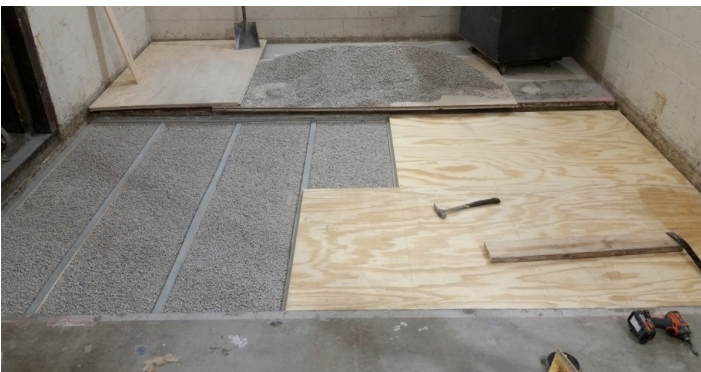
Figure 12 - Plywood subfloor partially installed
