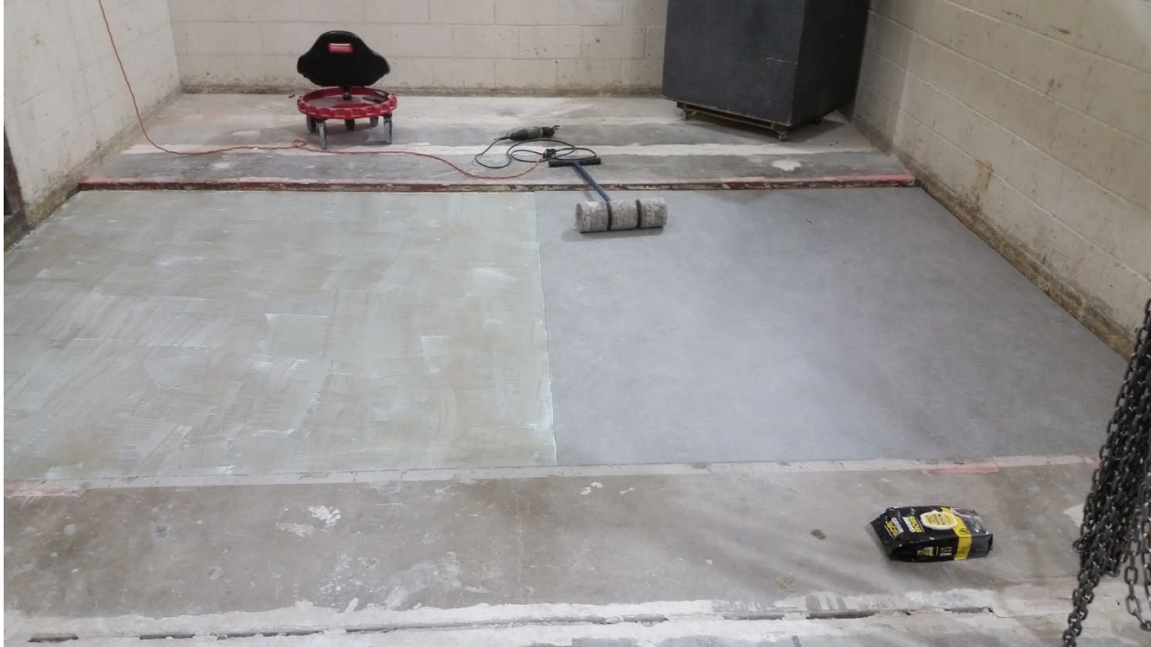
Figure 15 – Adhesive installed over gypcrete, flooring partially installed over adhesive
