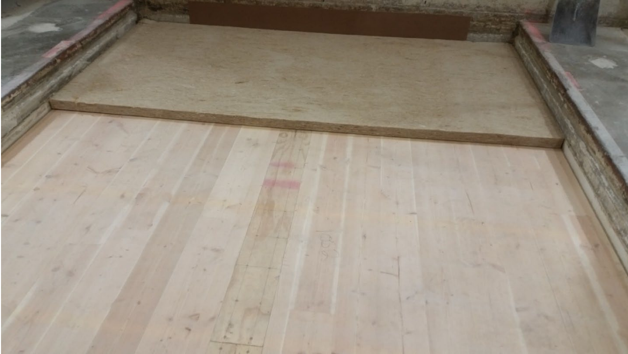
Figure 7 - Hemp board partially installed over CLT
