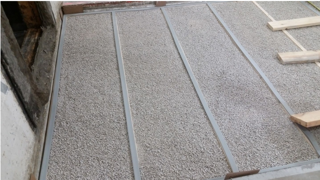
Figure 10 – Gravel installed; Piano B 40/40 partially installed to top of sleepers
