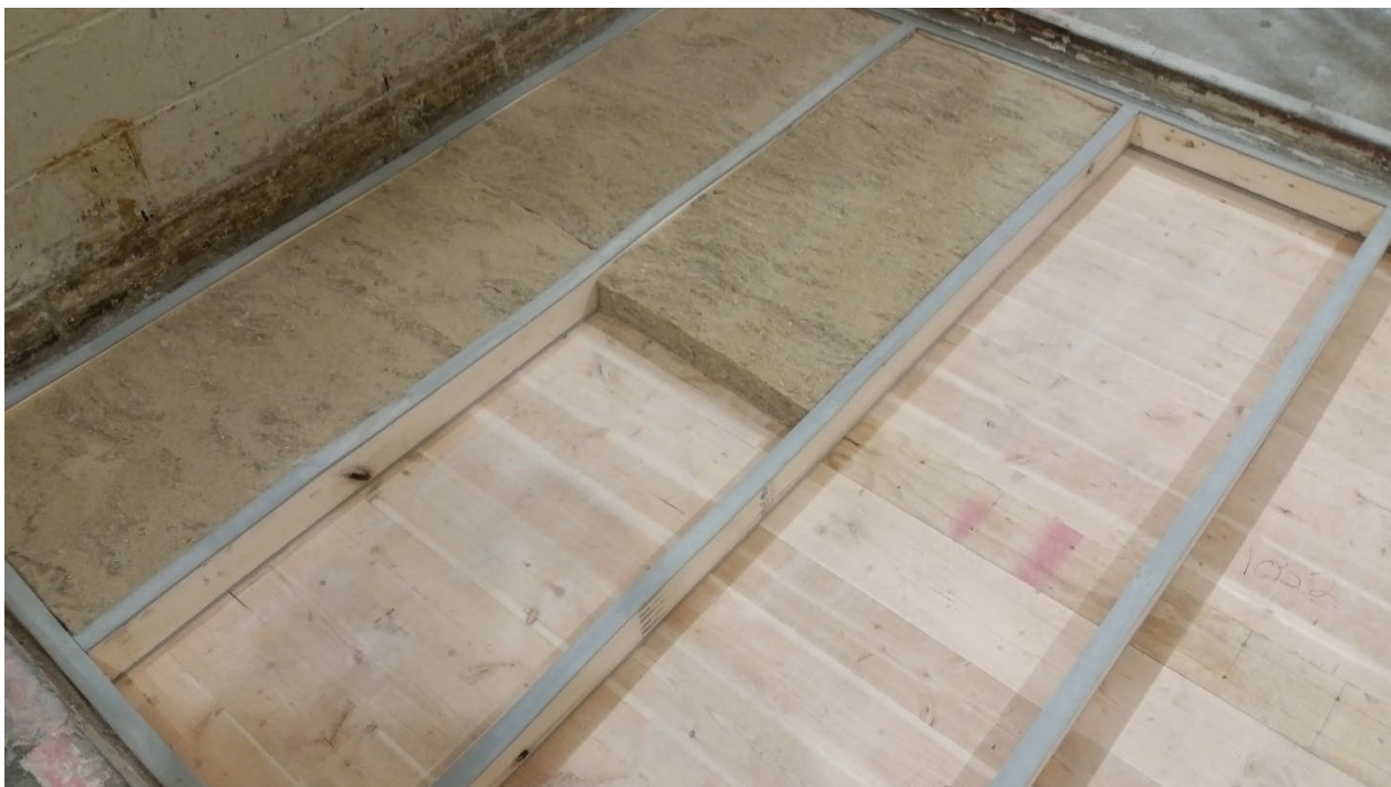
Figure 10 – Hemp boards partially installed between sleepers
