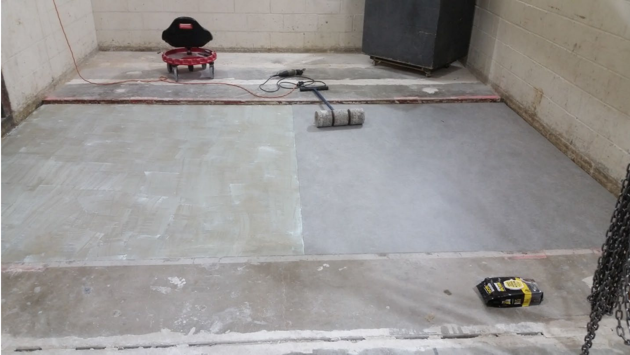
Figure 15 - Adhesive installed over gypcrete, flooring partially installed over adhesive
