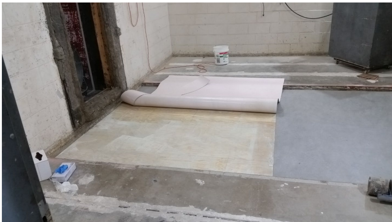
Figure 16 - Flooring partially installed
