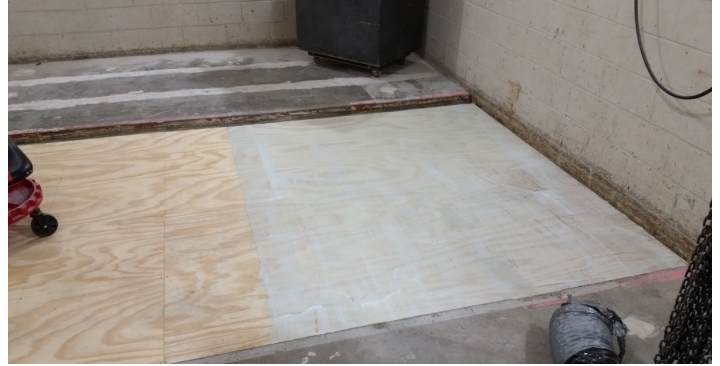
Figure 15 - Adhesive partially installed over plywood
