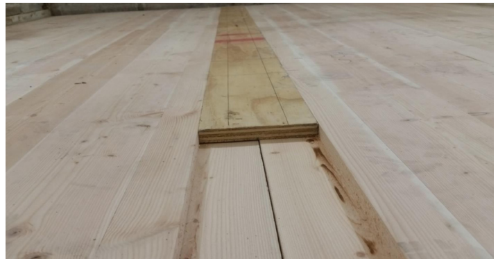
Figure 6 - Detail of 3/4" x 6" plywood spline partially installed over CLT rabbets
