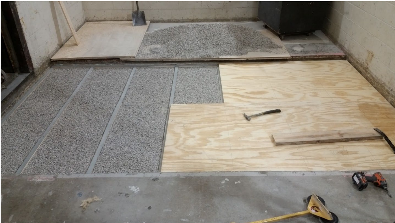
Figure 12 – Plywood subfloor partially installed
