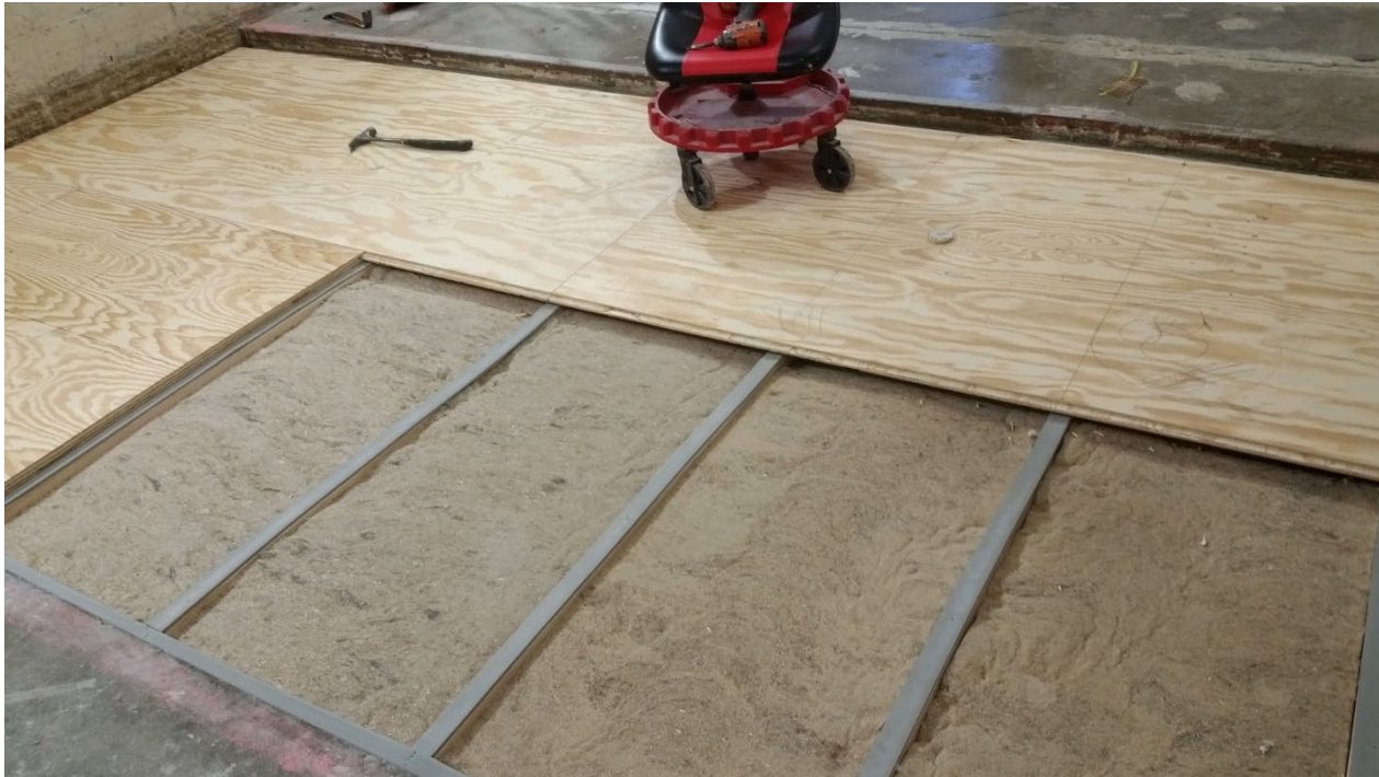
Figure 11 – Hemp boards installed between sleepers, plywood partially installed over sleepers
