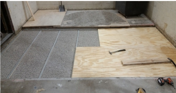
Figure 12 - Plywood subfloor partially installed
