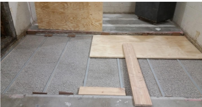
Figure 12 - Plywood subfloor partially installed
