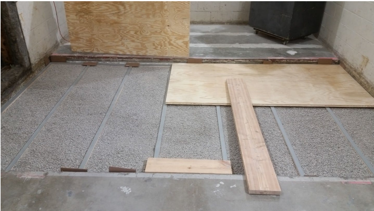
Figure 12 - Plywood subfloor partially installed
