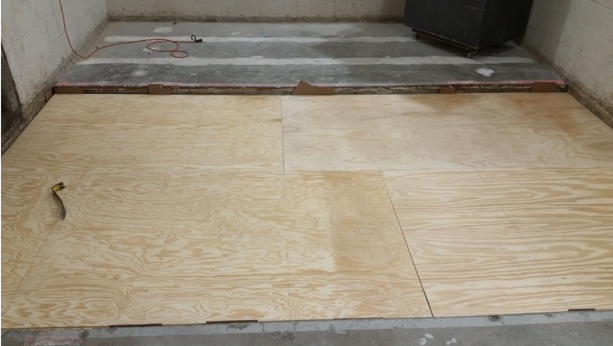
Figure 13 - Plywood subfloor installed
