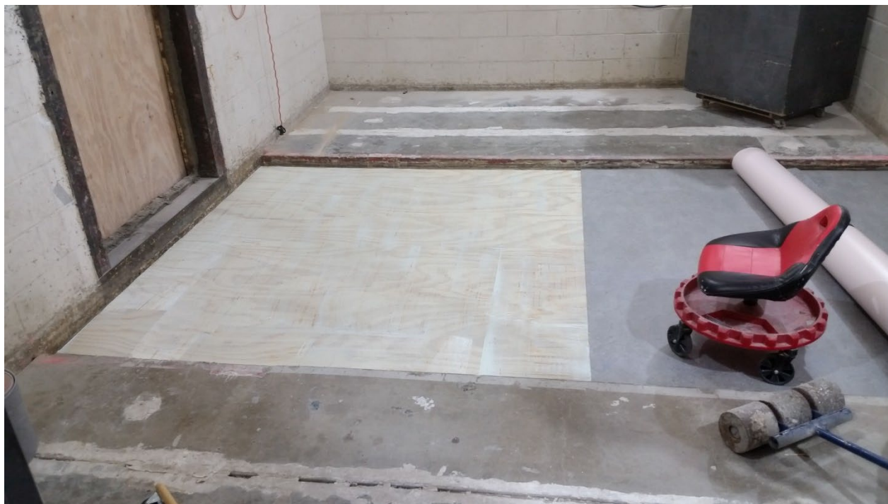
Figure 16 – Flooring partially installed over adhesive
