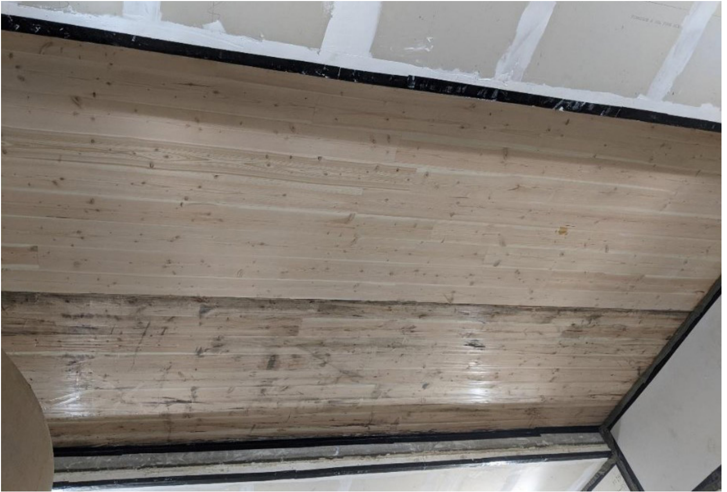
Figure 9 - F03 Assembly - CLT panels (from below)
