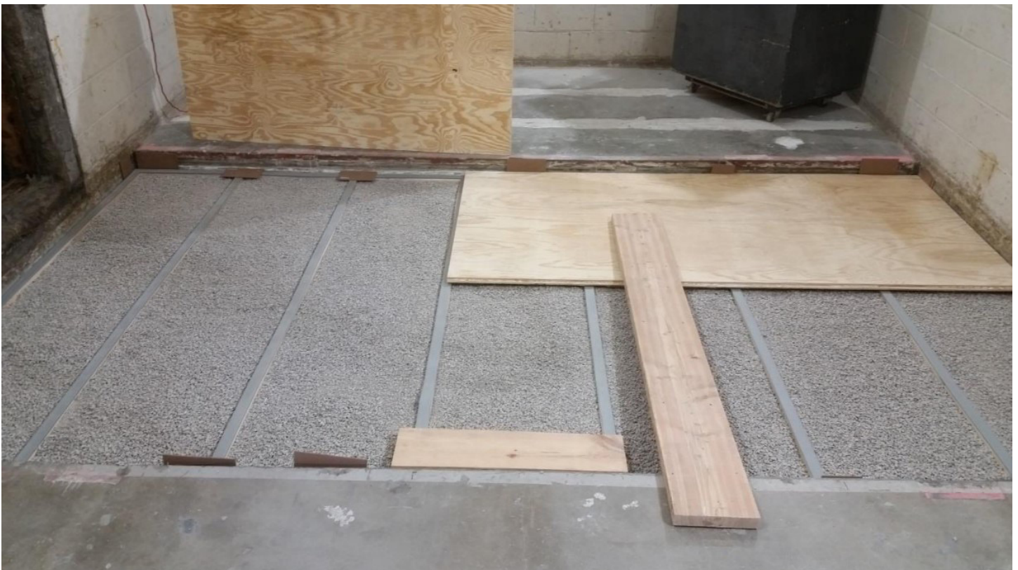
Figure 6 - F03 Assembly - Plywood subfloor partially installed (from above)
