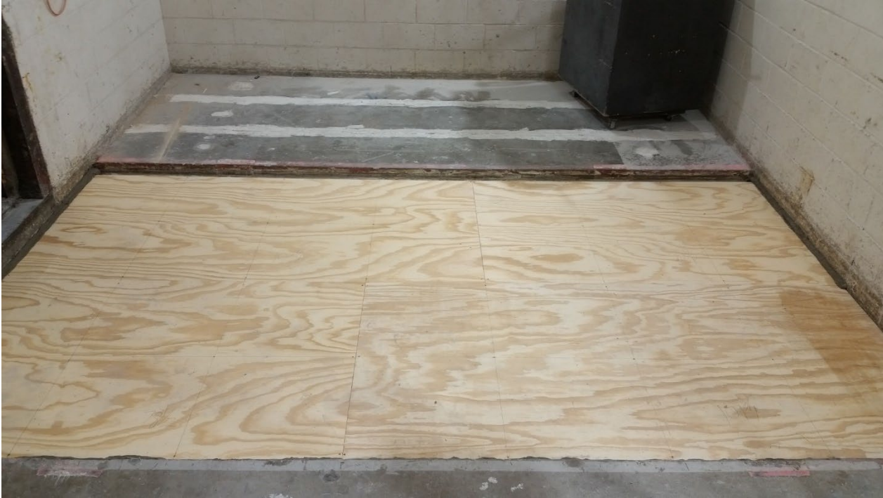
Figure 13 - Plywood subfloor installed
