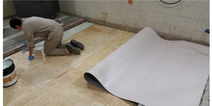
Figure 15 - Adhesive being troweled over plywood prior to installation of flooring
