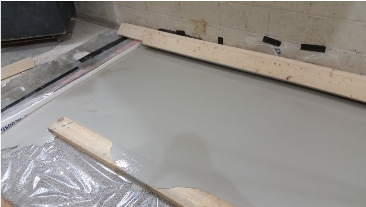
Figure 12 – Gypcrete partially installed over vapor barrier
