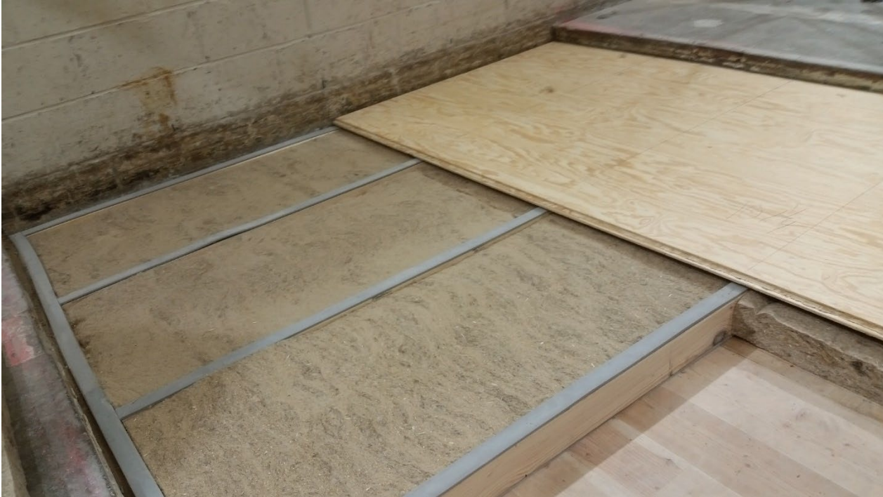
Figure 11 – Hemp boards partially installed between sleepers, plywood partially installed over sleepers
