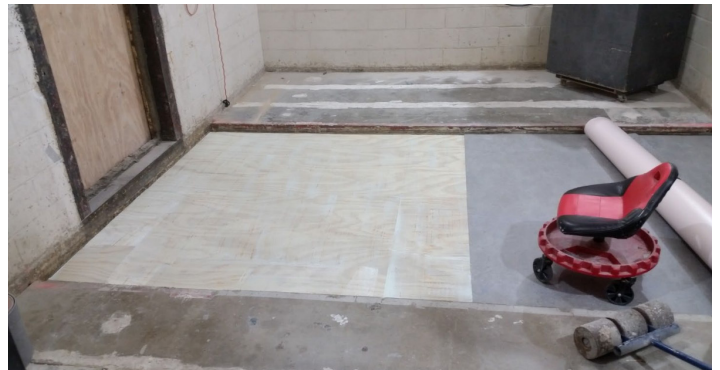
Figure 16 - Flooring partially installed over adhesive
