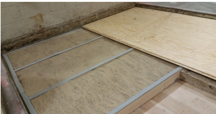
Figure 11 - Hemp boards partially installed between sleepers, plywood partially installed over sleepers
