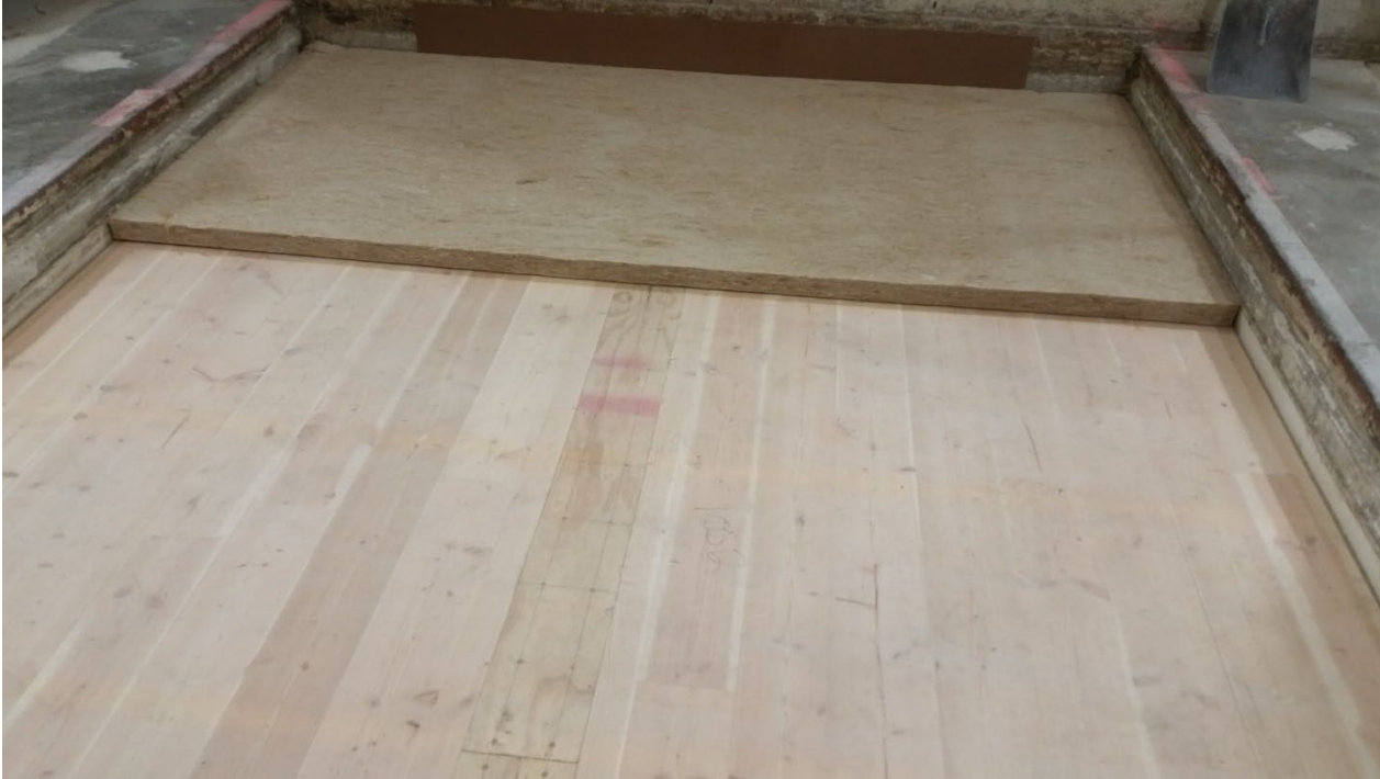
Figure 7 – Hemp board partially installed over CLT
