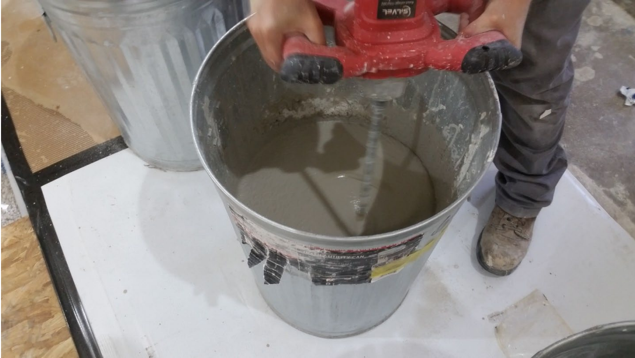
Figure 11 – Gypcrete mixing prior to pouring
