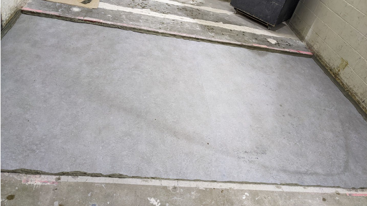
Figure 1 – Specimen mounted in test aperture, as viewed from source room
