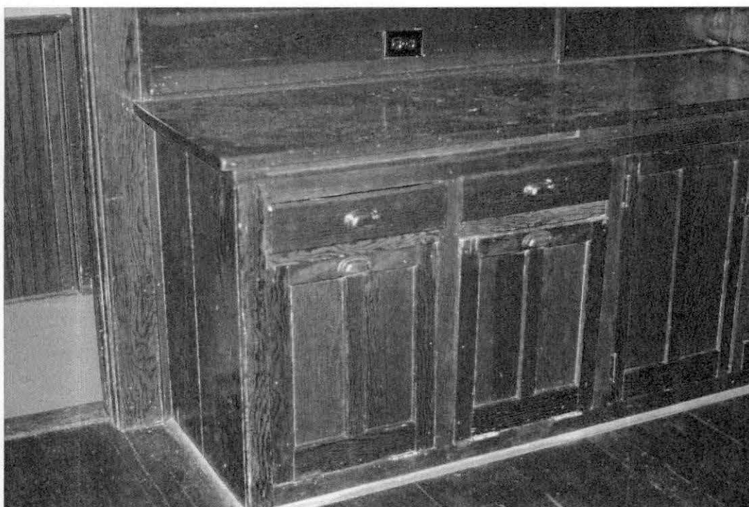
FIGURE 64. Soultz-Westfall Duplex, Base Cabinets. Photo by Author.
