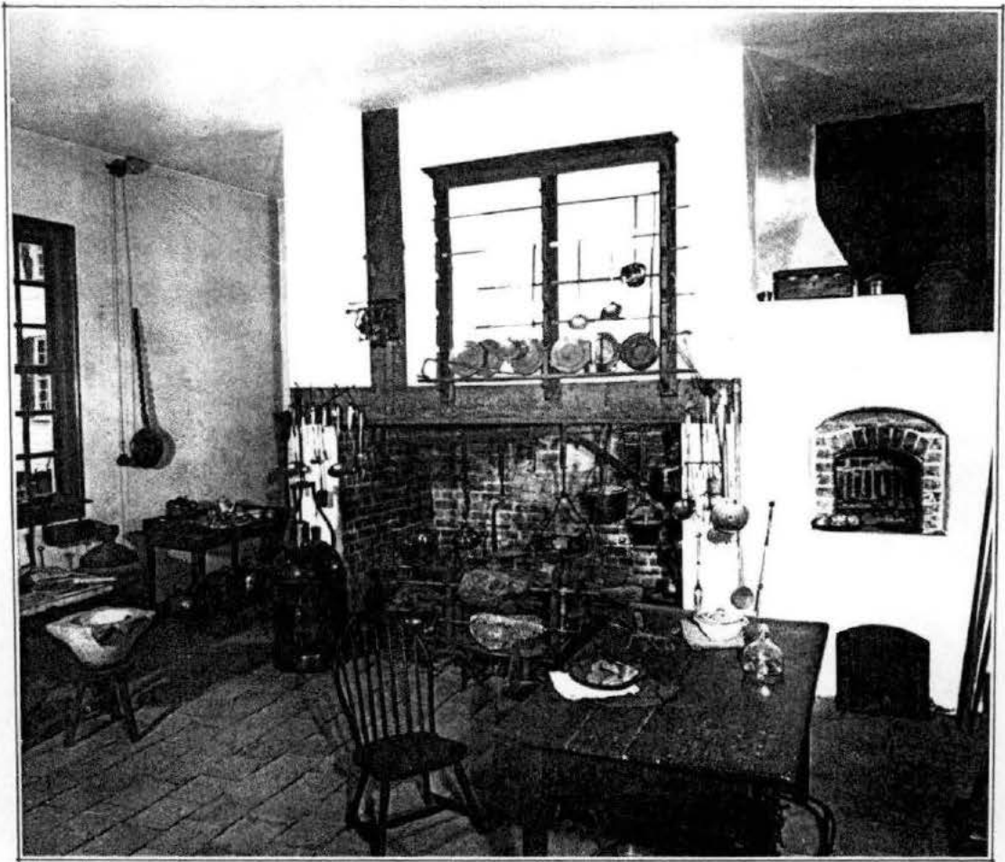
FIGURE 3. Eighteenth Century Fireplace with Side Oven. Source: Ladd, Early American Fireplaces , (New York: Hastings House Publishers, 1977), 126.
