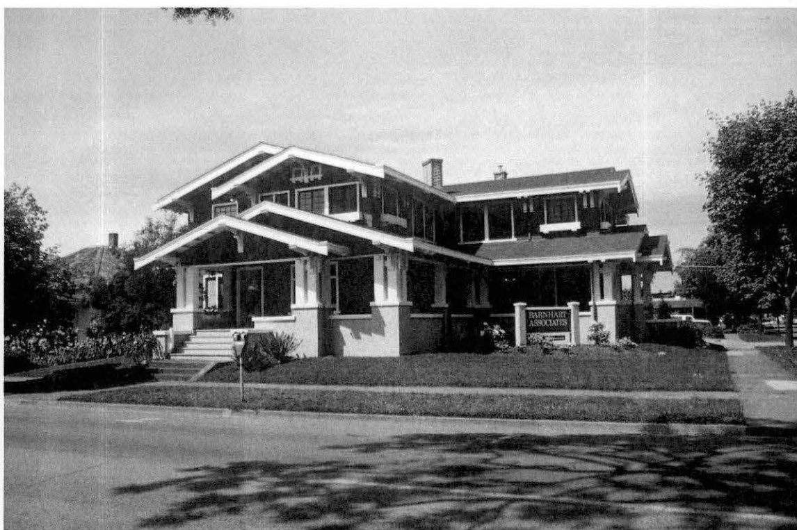
FIGURE 56. Soultz-Westfall Duplex, Exterior. Photo by Author.
