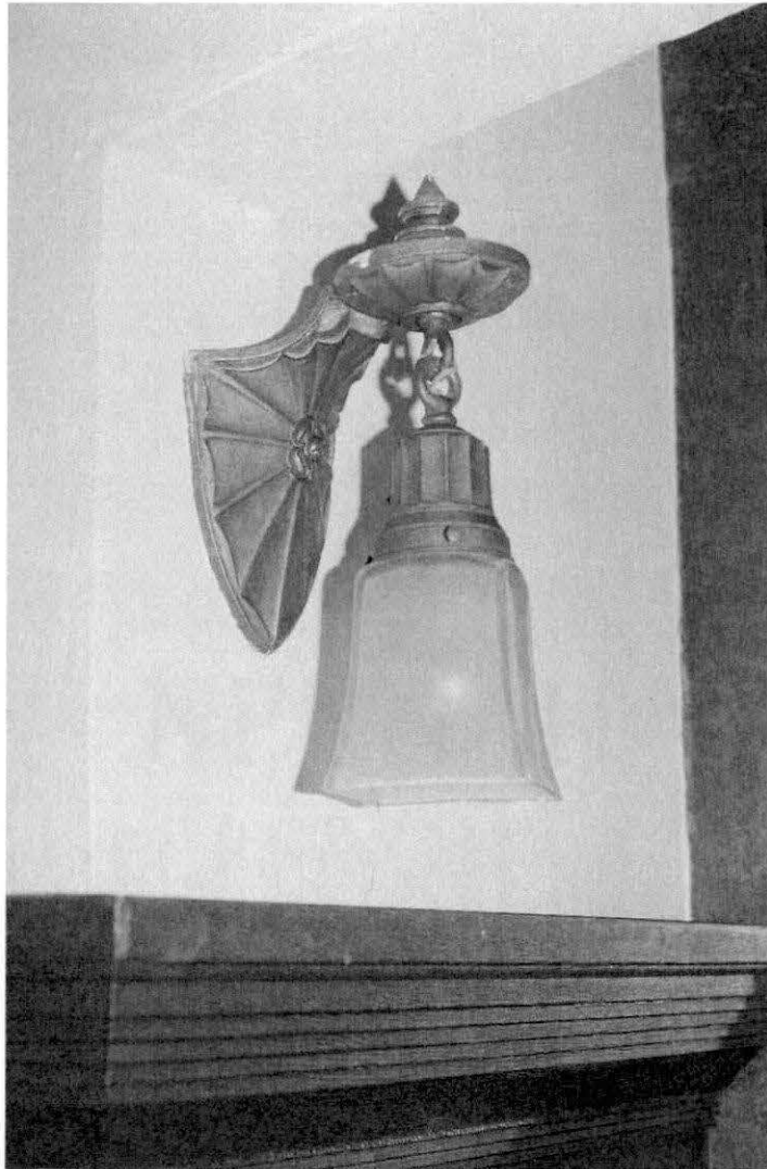
FIGURE 50. Soultz-Westfall Duplex, Craftsman Lighting Fixture. Photo by Author.
