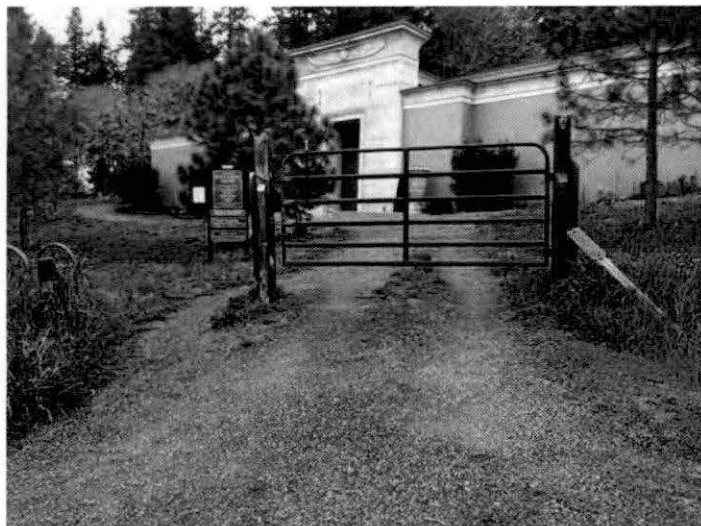
SW entrance looking NE
