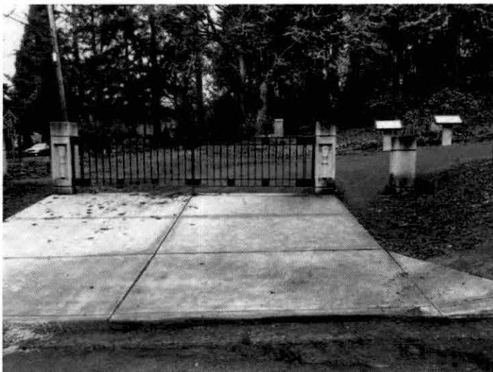
NW entrance looking E
