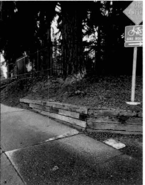
NE corner showing fence looking SW
