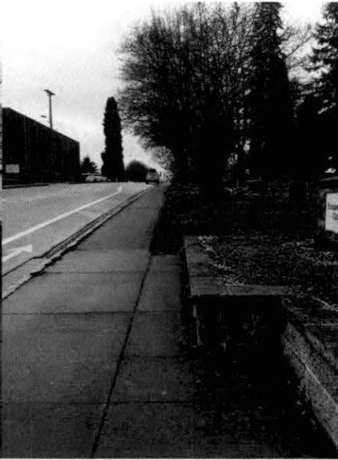
S perimeter looking W
