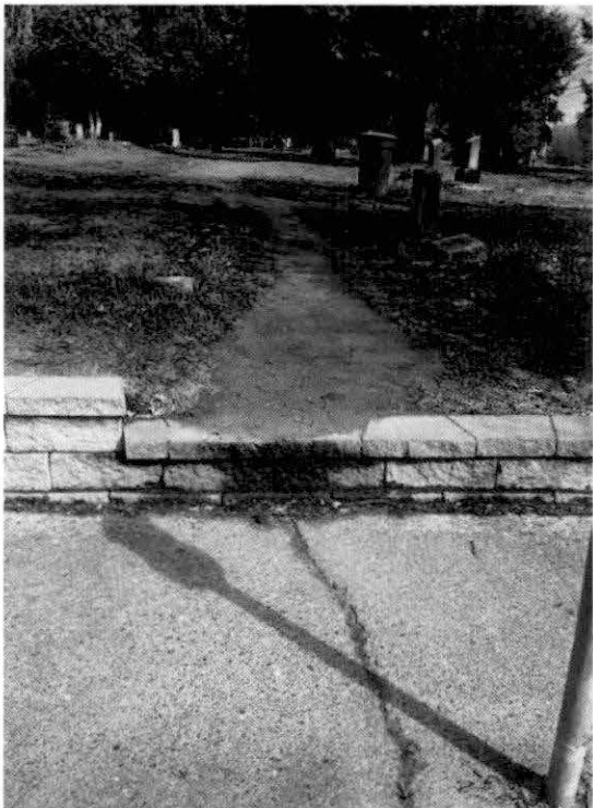
Social trail on S perimeter, looking N
