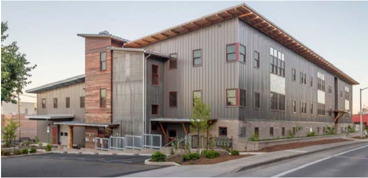
Source: Essex General Construction – Mahonia Building (2019)
