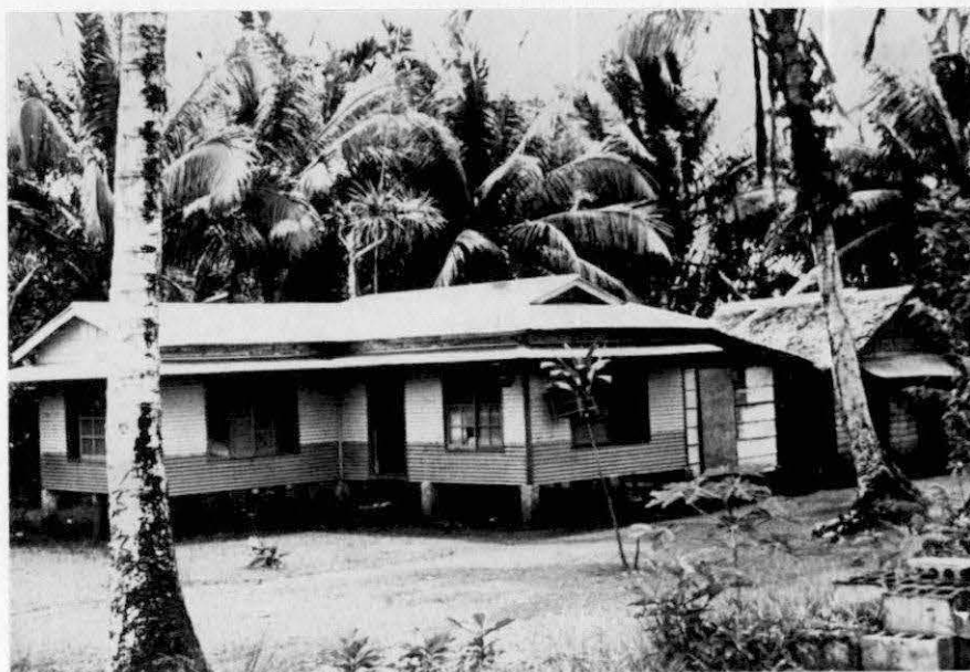
FIGURE 25. Maidesil's house (Letter 'k' on Figure 18) illustrates the larger house built of milled lumber, brick pilings, corrugated iron, and embellished with sliding glass windows.
