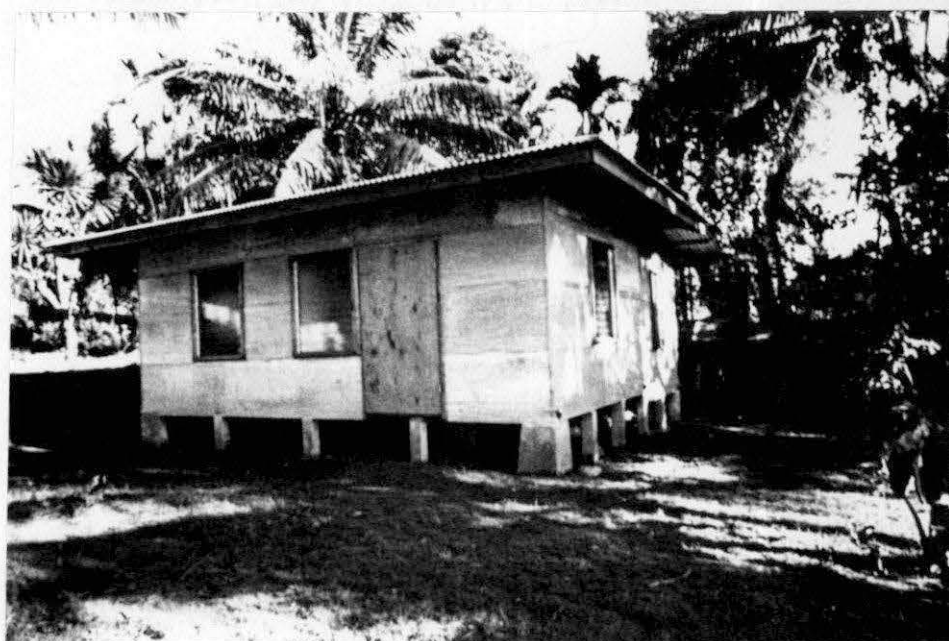
FIGURE 26. Mellemat's house (Letter 'D' on Figure 18) illustrates the larger house built of concrete pilings, milled lumber, and corrugated iron. This house has such luxuries as louvered windows, linoleum floors and fabricated wood panel interior walls.
