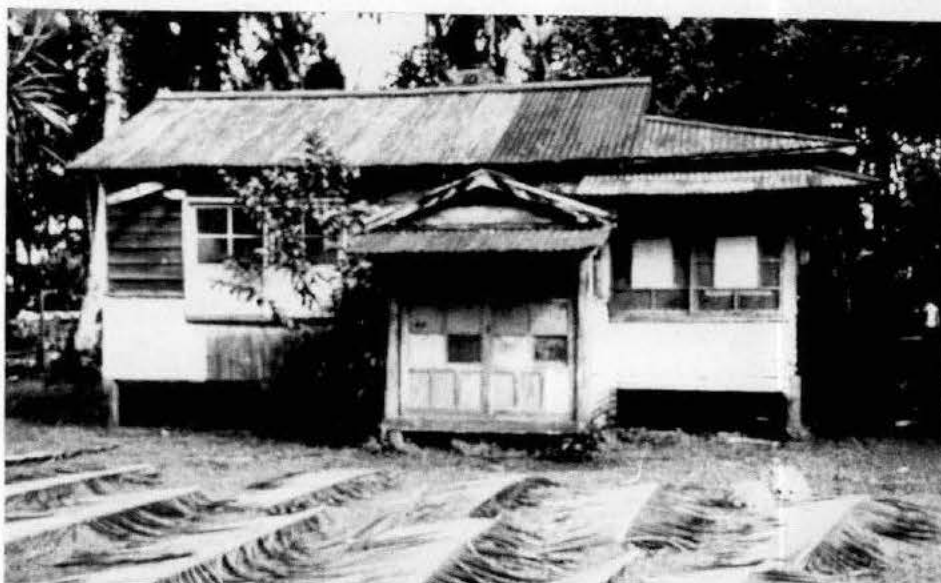
FIGURE 24. Renguul's house (Letter 'j' on Figure 18) illustrates the smaller house built on milled lumber, bamboo, and corrugated iron.
