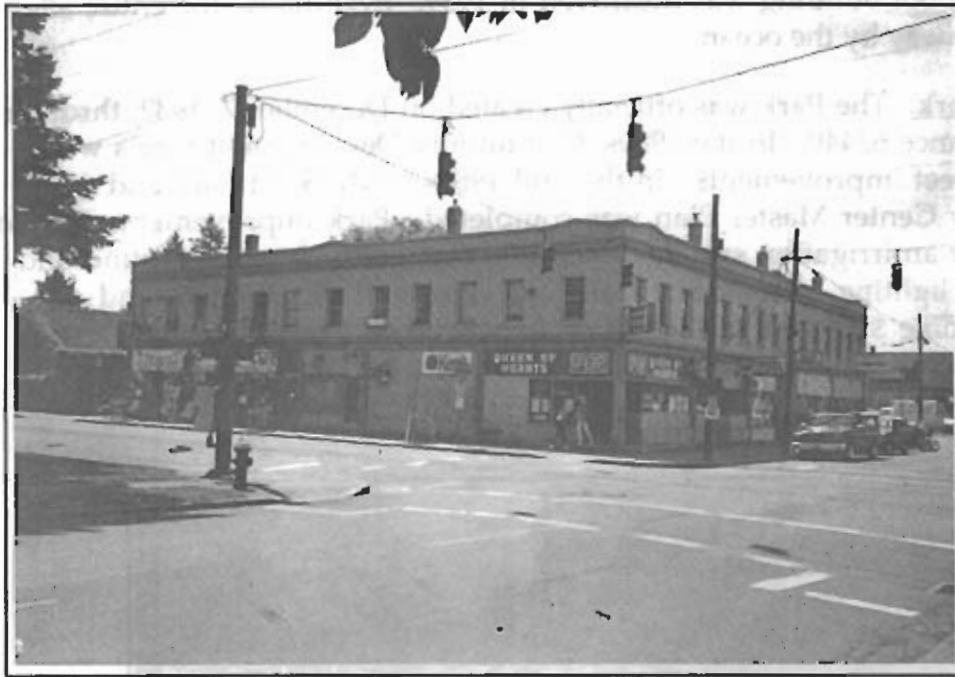
This Street Car Era Building at SE 72nd Avenue and Harold Street is an important landmark for neighborhood residents.
