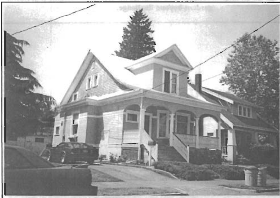
The graceful form of this stately porch graces the street.
