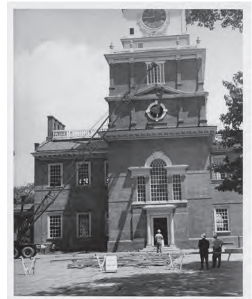
Efforts by Nelson during the restoration of Independence Hall ensured the restored building appeared as it did when the Declaration of Independence and U.S. Constitution were written there in the 1700s. Photograph courtesy of UO Libraries Special Collections.
