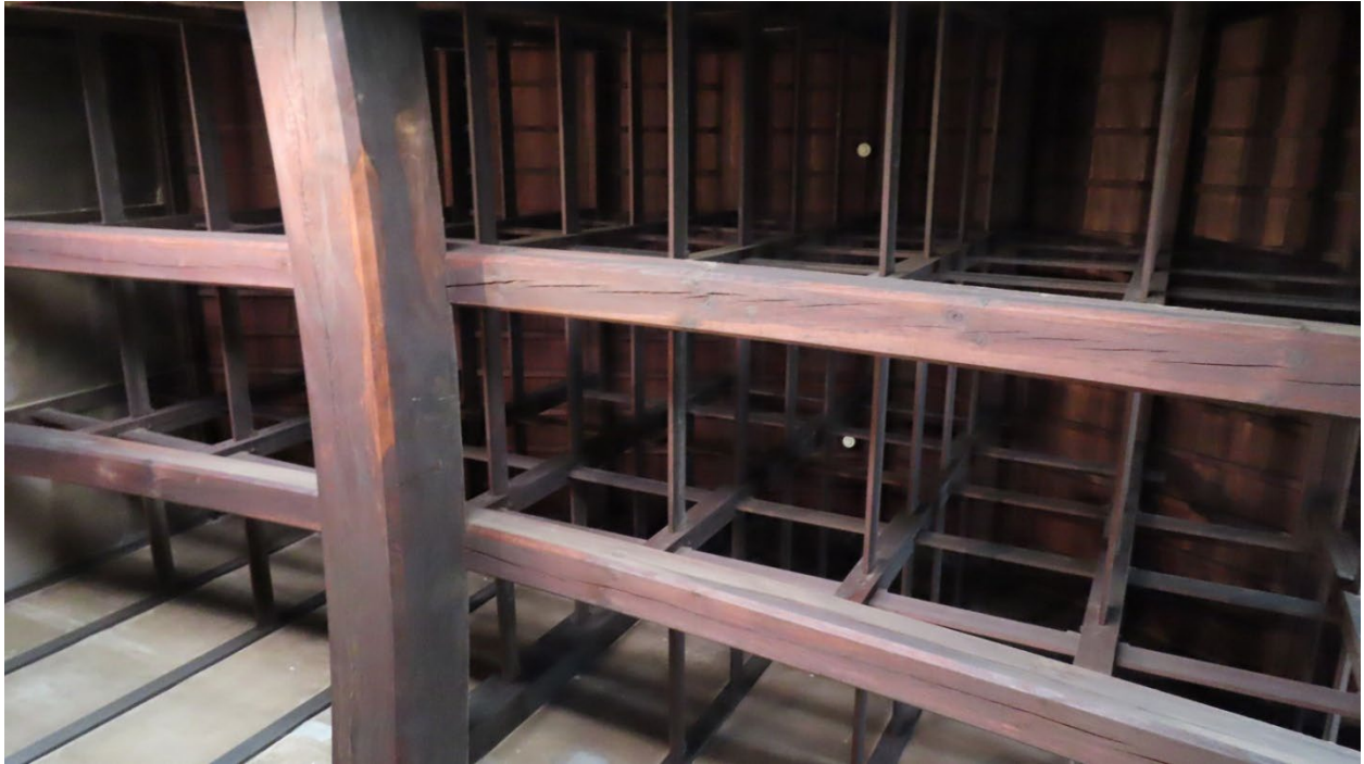
Fig. 2.1 – Internal Machiya Roof Structure , Meiji Period, Completed 1903, omoteya-zukuri, Former Konishi Residence, Chuo (this area was Doshomachi, the medicine town), Osaka
