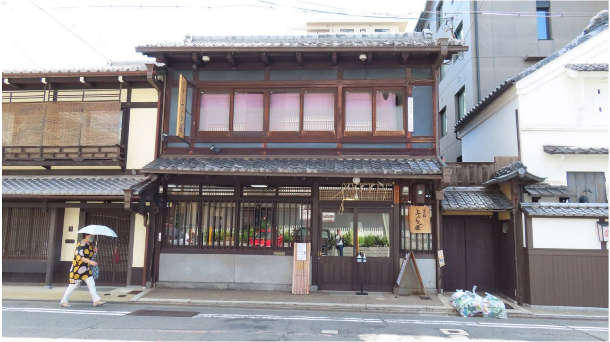
Fig. 4.10 – Exaggerated-Shinkabe Style with stone base and metal bars on first story windows, Kamanza Street, Nakagyō, Kyoto
