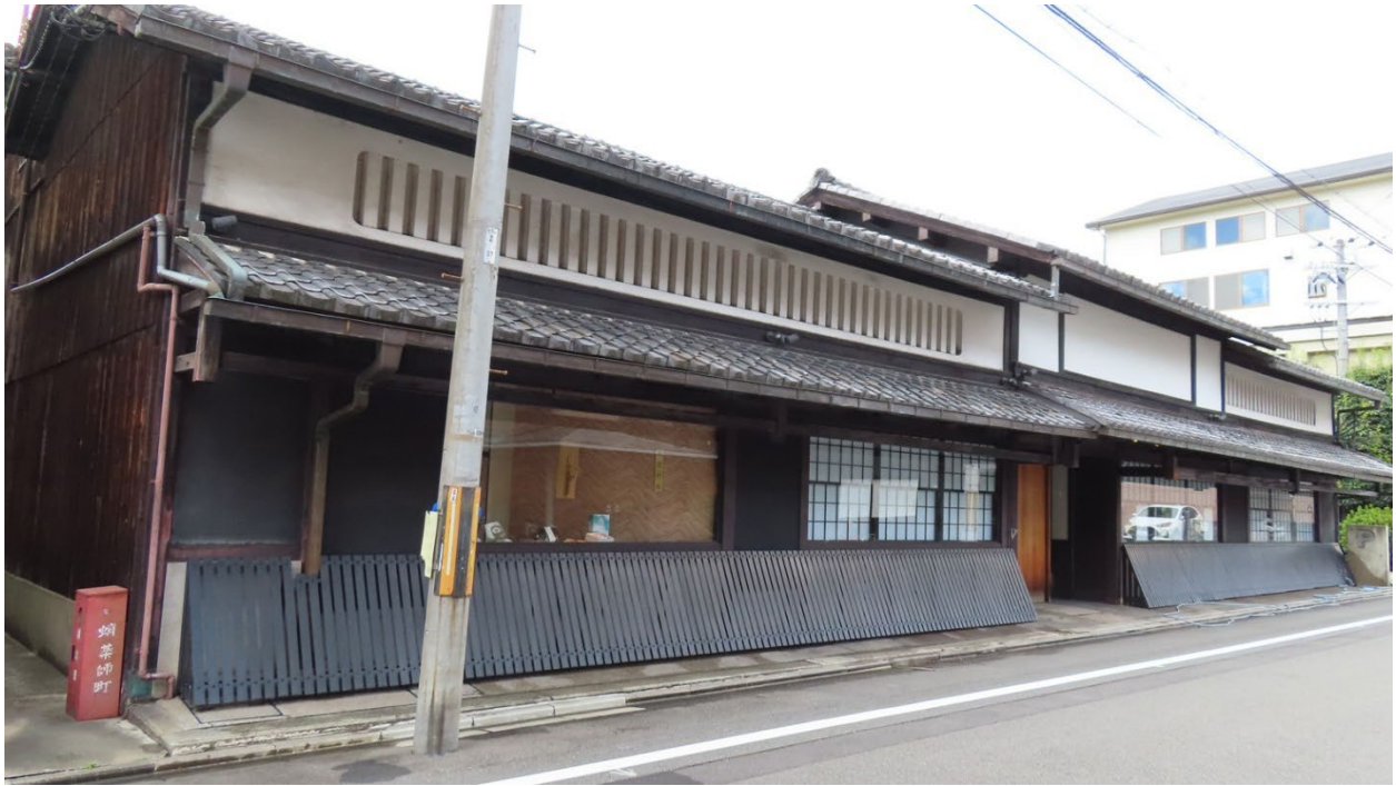
Fig. 2.21 – Inuyarai , Muromachi Street, Nakagyo, Kyoto
