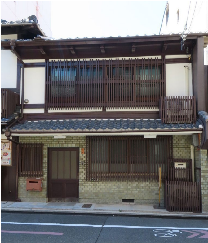
Fig. 4.11 – Exaggerated-Shinkabe Style with brick first story, Kamanza Street, Nakagyō, Kyoto
