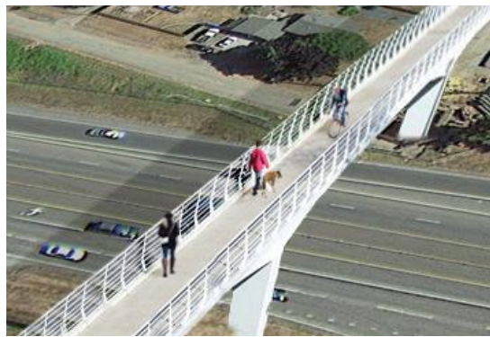
Figure 13: A bicycle/pedestrian bridge across Highway 126 provides a safe crossing.
