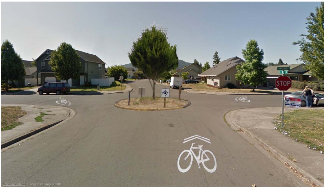
Figure 24: A traffic circle at 41st Street and Virginia Street makes the neighborhood safer for all users.
