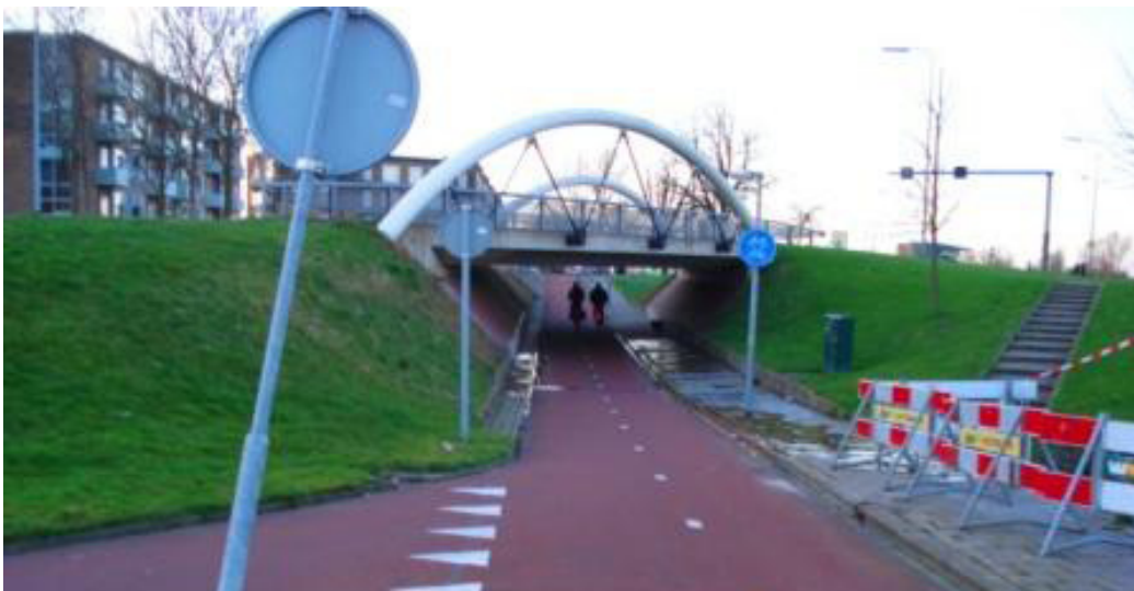
Figure 4: A tunnel carries bicyclists under a busy roadway (Shahan 2011).
