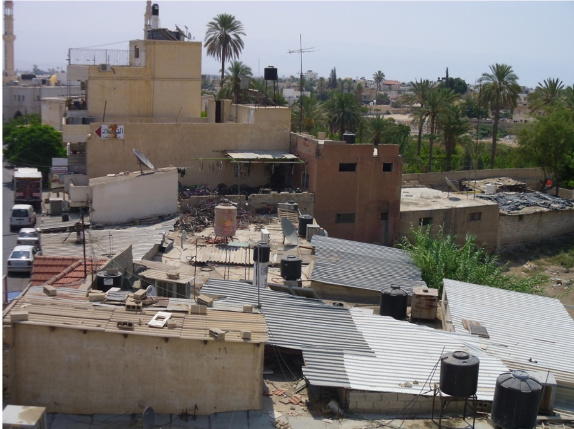
Figure 7: Rooftop tanks in Jericho city, photo by author.
