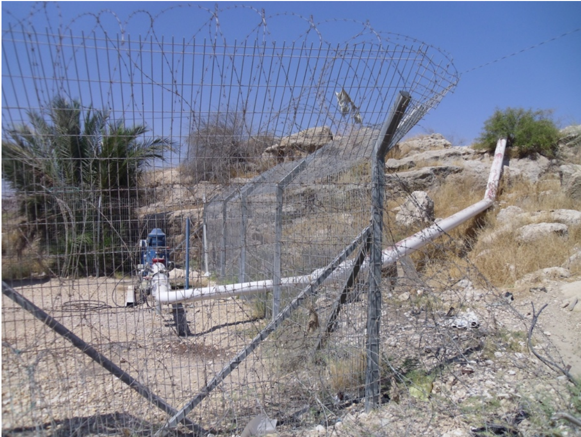
Figure 9: Pipe to Argaman, Israeli settlement, photo by author.
