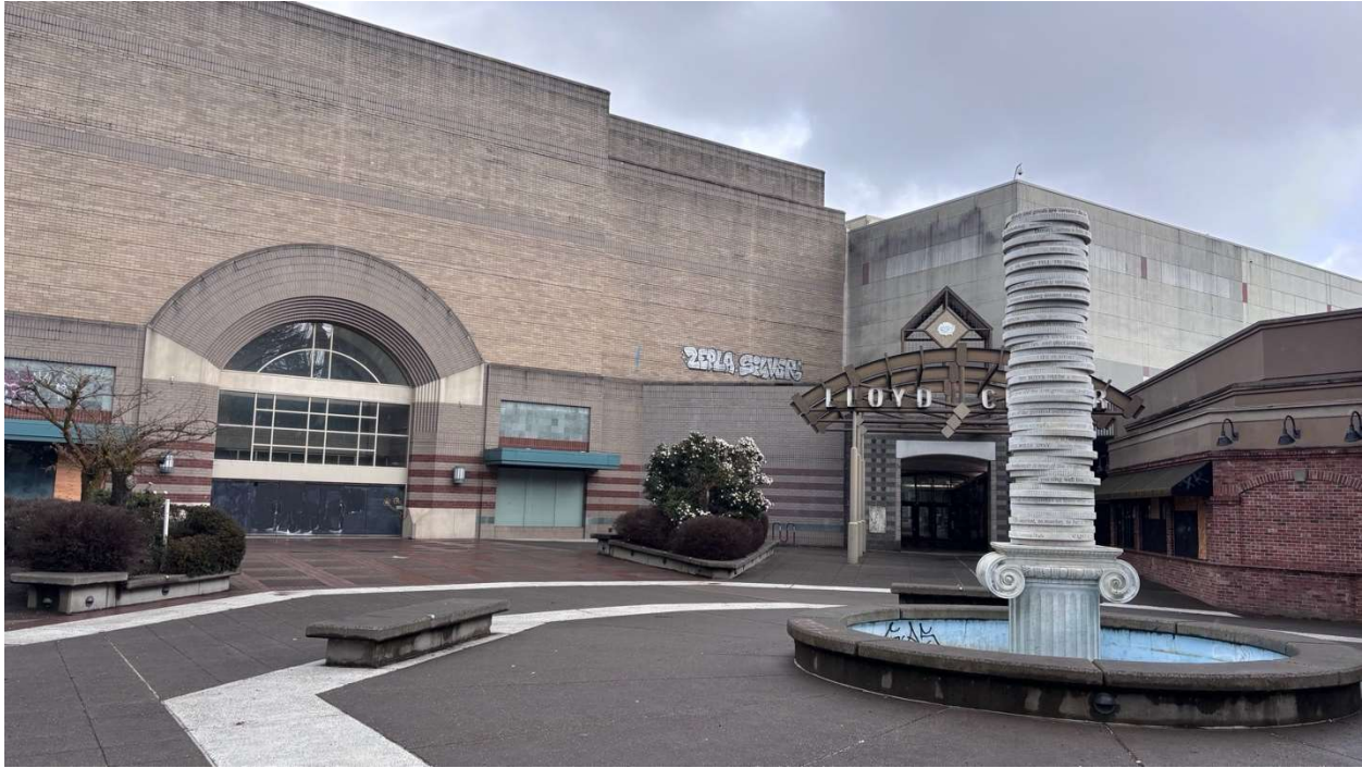
Figure 13: Southwest Lloyd Center Entrance Plaza — Close Up View
