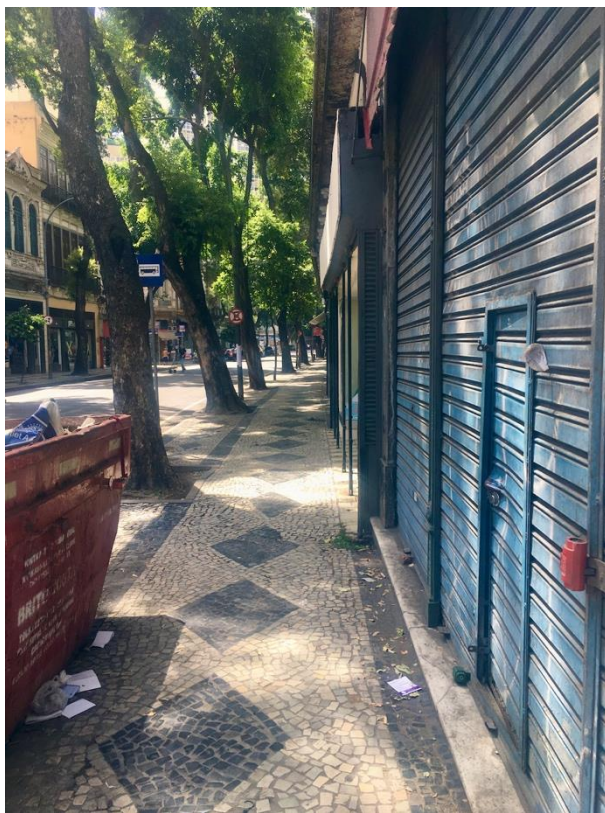
Figure 31 The little blue door through which the MMOB entered to occupy the building. Note the indentation near the lock where they pried open the door.
