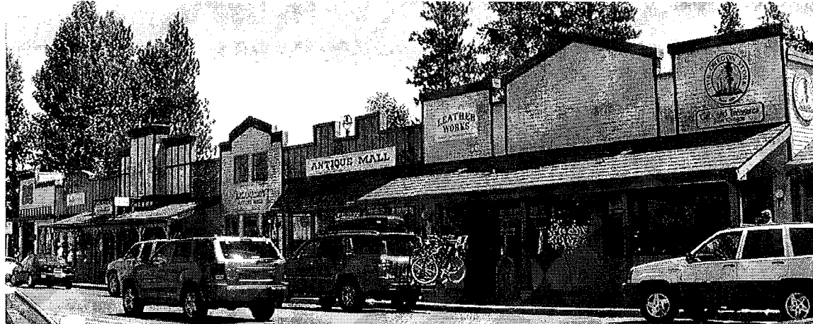
Antique Mall Building – 261 W. Cascade Avenue
