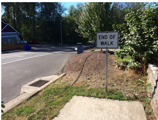
Figure 3B: Disconnected sidewalks prevent safe and directed pedestrian flow
