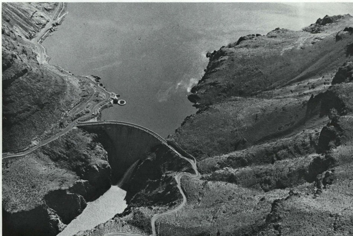
Figure 21. Owyhee Dam from the air. The abutments are against a body of rhyolite which has caused narrowing of the canyon here, creating an ideal place for a dam. The ring-like object is the gloryhole spillway.
