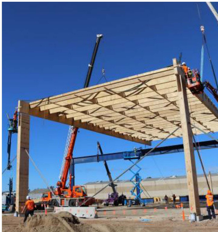
Above : Middle Box Beam that spans 104'-10" getting craned into place made up of 3'-10" box beam and purlins.
