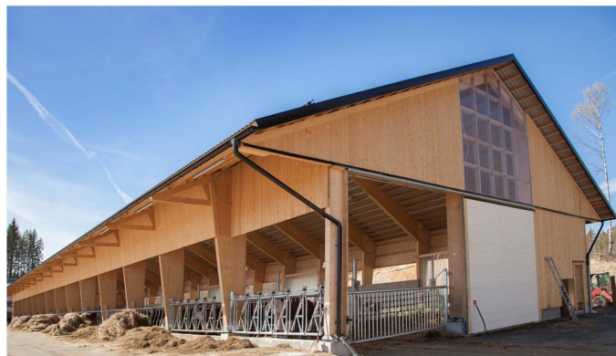
Above : Roof line extend out beyond edge of LVL frame to allow for large overhang.
