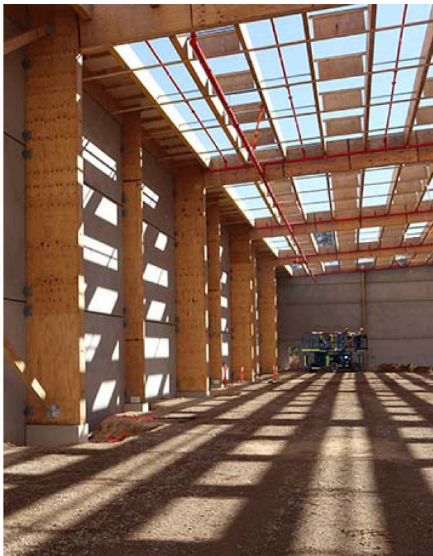
Above : End Wall Bracing is dealt with through precast concrete panels laid out horizontally.
