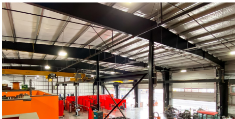
I&E Construction Woodburn, Oregon | 30,000 sf
