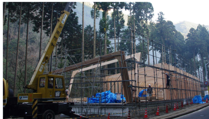
Above : Glulam frames were constructed on the ground by hand, and then raised by crane into place.
