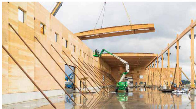
Above : Sections of the roof were constructed on the ground and craned into place to speed up the construction process.
