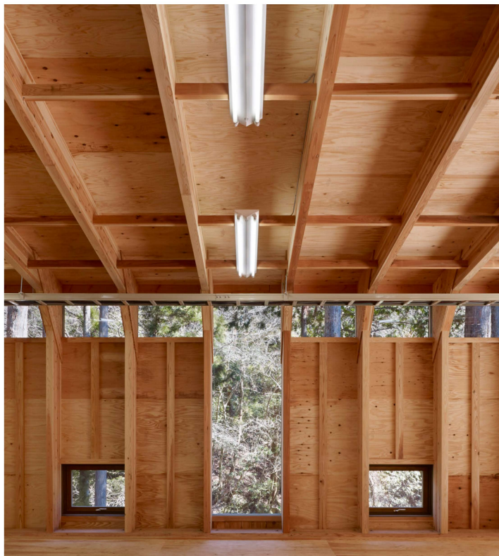
Above : As the walls are not bearing, clerestory windows wrap around the entire facade like ribbon.
