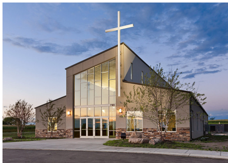
Riverwood Covenant Church Rockford, Minnesota | 12,655 sf
