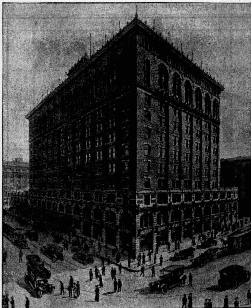
Fig. 1 Main Portion of the Davenport Hotel Built in 1913. (Source: Cheney Cowles Museum, Spokane.)
