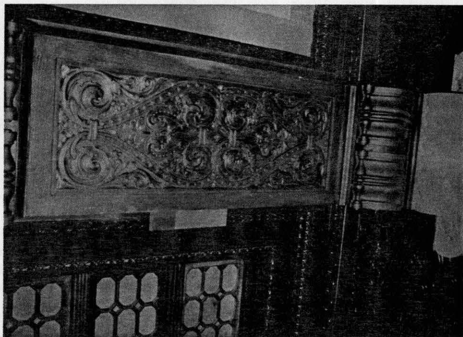
Fig. 7 Davenport Hotel, Underside of Beam, Present. (Source: author's photograph.)
