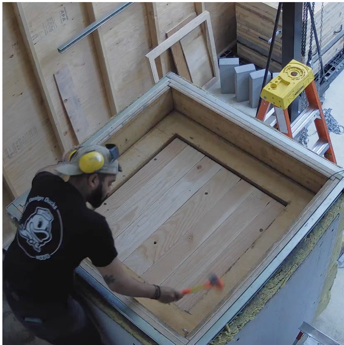
place on the 'donut' sealing ring, allowing for a small gap (1/8 ") around the edge of the panel
