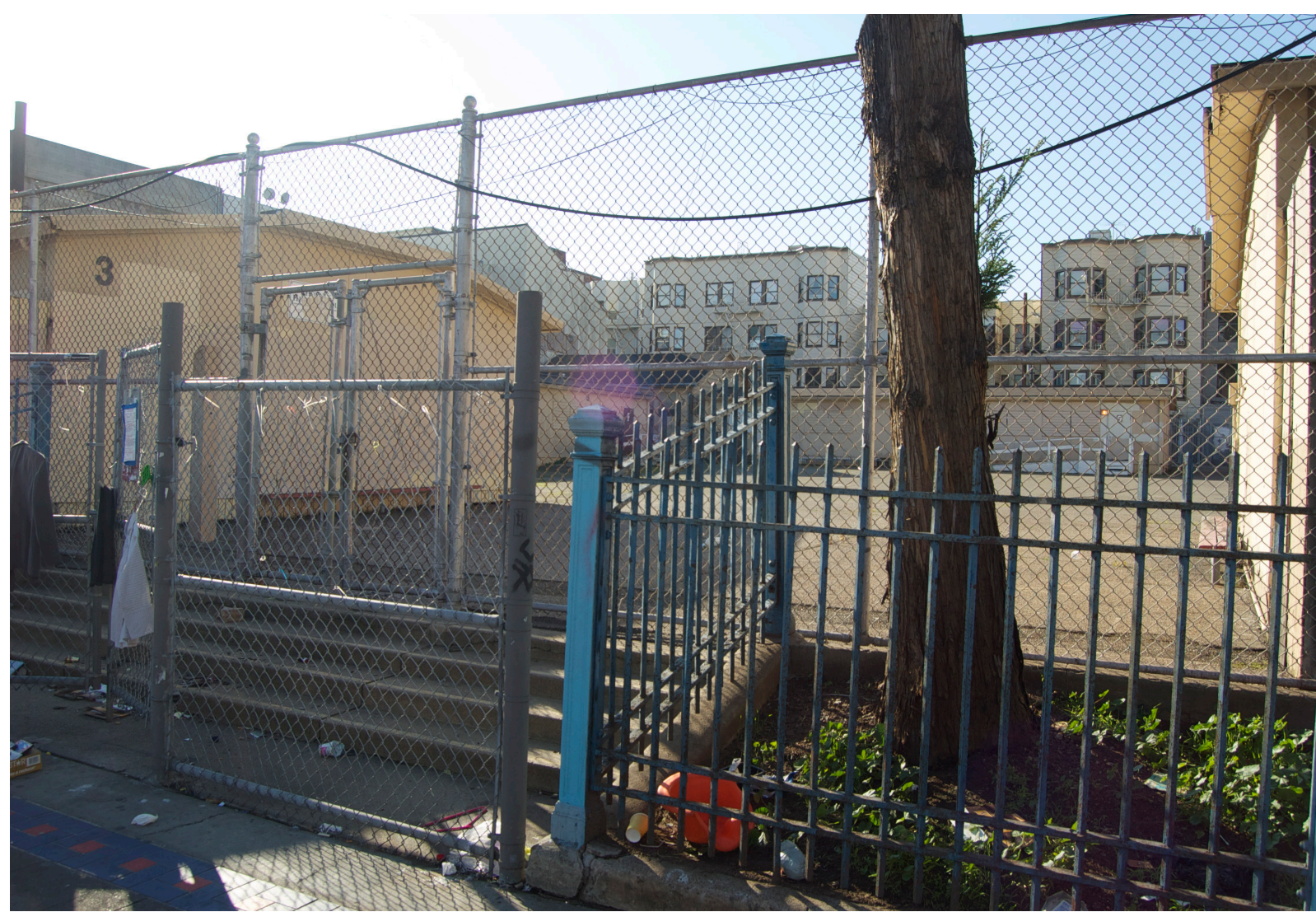
PRE-EXISTING STRUCTURE FROM EAST
