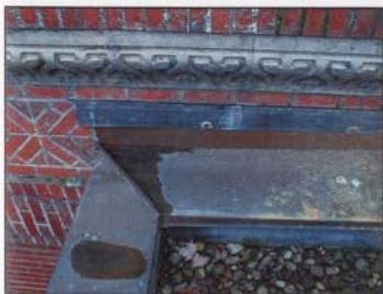
FIGURE 57: FLASHED CONNECTION AT THE TOP OF THE 1951 ADDITION.
