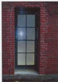
FIGURE 17: WINDOW OPENING ADDED TO THE NORTH ELEVATION ON THE FIRST FLOOR
