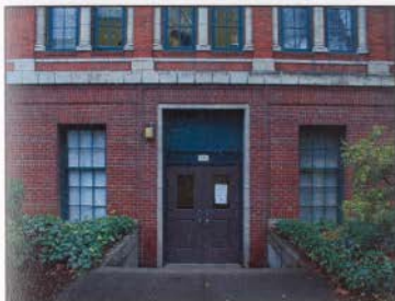
FIGURE 16: SOUTH ENTRY WITH ALTERED TRANSOM
