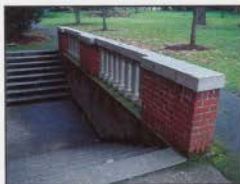
FIGURE 61: WALL AND STAIR AT EAST ENTRY
