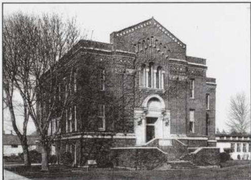
FIGURE 1: 1916 EDUCATION BUILDING SOUTHEAST ELEVATION – CIRCA. 1935 Lawrence Collection, Courtesy of Special Collections, Knight Library, University of Oregon.
