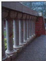
FIGURE 63: MECHANICAL ABRASION OF GLAZE FROM BICYCLE CHAINS
