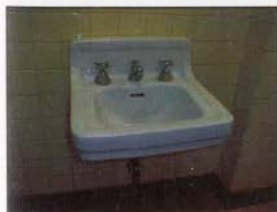
FIGURE 49: ORIGINAL SINK FIXTURE
