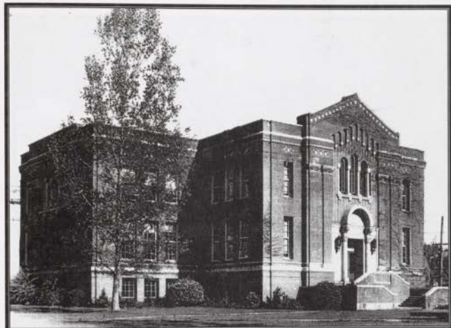
FIGURE 121: COMMERCE HALL NORTHWEST ELEVATION – CIRCA. 1945
