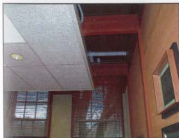
FIGURE 19: SUSPENDED CEILING, RM 201
