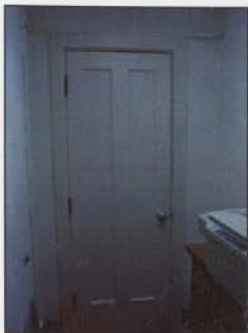
FIGURE 87: TYPICAL HISTORIC SECONDARY DOOR
