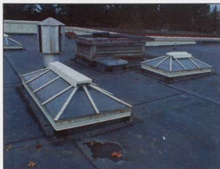
FIGURE 35: GABLED SKYLIGHTS WITH OPERABLE VENT CAPS
