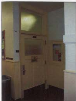
FIGURE 86: ROOM 364. ALL ORIGINAL MILLWORK
