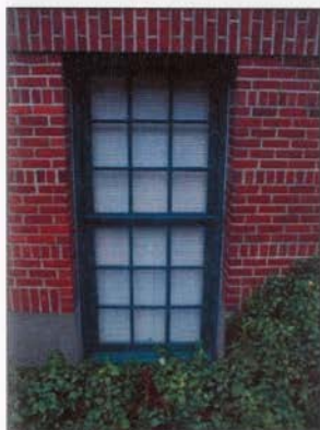
FIGURE 77: TYPICAL 9 OVER 9 WOODEN SASH
