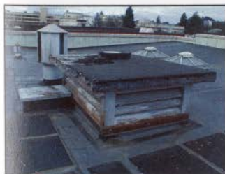
FIGURE 32: HISTORIC ROOF VENT "PENTHOUSE"
