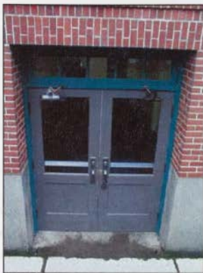
FIGURE 76: FIRST FLOOR ENTRY DOORS AT SOUTH ELEVATION
