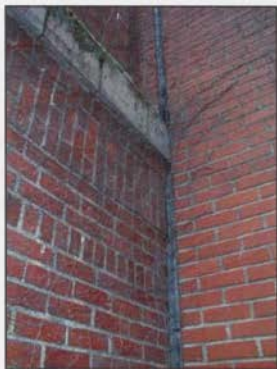
FIGURE 58: DETAIL OF THE EXPANSION JOINT SEAM BETWEEN COMMERCE HALL AND THE 1951 ADDITION
