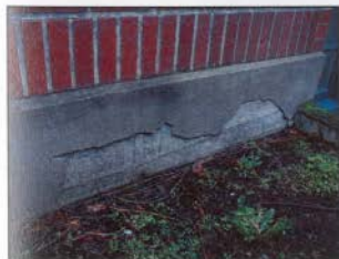
FIGURE 21: STUCCO DETERIORATION
