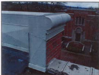
FIGURE 56: BACK OF CAVITY WALL WITH COPPER COPING INSTALLED
