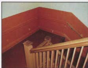
FIGURE 89: STAIRWELL WITH MOLDINGS, RAILS, BALUSTERS AND NEWELS
