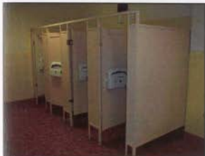
FIGURE 88: ORIGINAL BATHROOM STALLS
