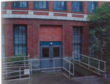
FIGURE 14: HANDICAP RAMP AT EAST ENTRY, 1975 NOTE THAT THE TRANSOM WAS BRICKED-IN
