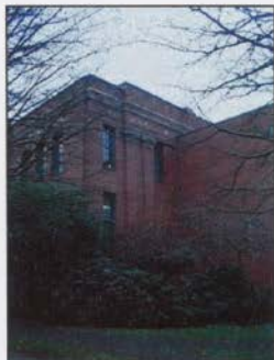
FIGURE 52: EAST SIDE OF THE NORTH ELEV.
