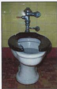
FIGURE 48: ORIGINAL TOILET FIXTURE
