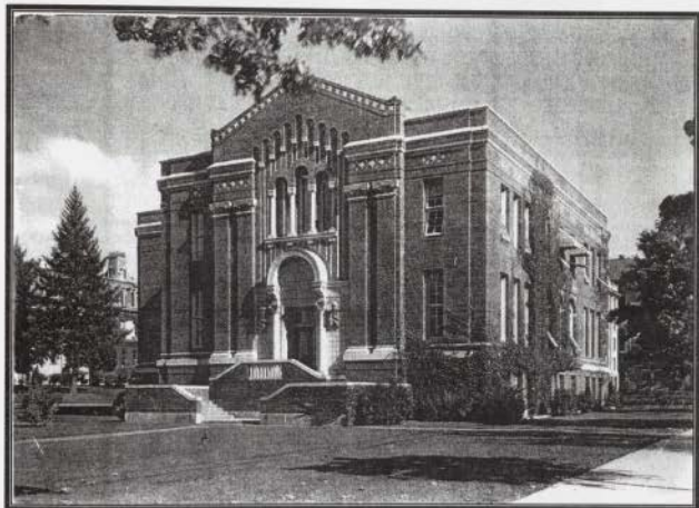
FIGURE 122: COMMERCE HALL SOUTHWEST ELEVATION – CIRCA. 1930 Lawrence Collection, Courtesy of Special Collections, Knight Library, University of Oregon.
