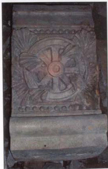
FIGURE 103: PILASTER CAPITAL Type: Pilaster capital Number: 1 each Glazing: Glazed buff clay body Size: 27"x15 1/2" x 14" Condition: Good condition Original Location: Extra piece
