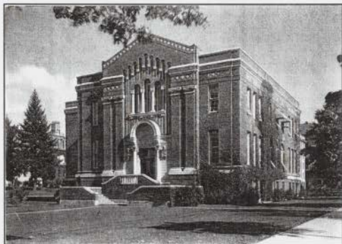
FIGURE 2: 1921 COMMERCE HALL NORTHWEST ELEVATION – CIRCA. 1930 Lawrence Collection, Courtesy of Special Collections, Knight Library, University of Oregon
