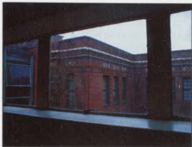
FIGURE 54: VIEW FROM THE COMMONWEALTH ADDITION
