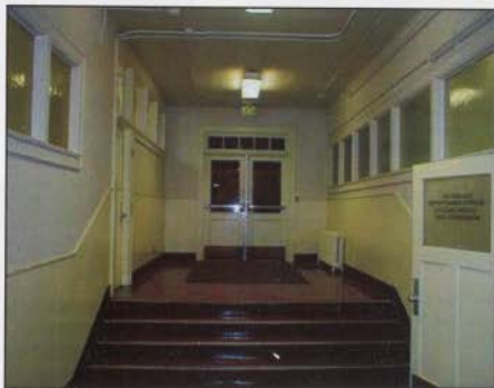
FIGURE 85: EAST ENTRY AT FIRST FLOOR. NOTE THE CONCENTRATION OF HISTORIC FABRIC.
