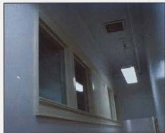
FIGURE 91: WINDOW BANK IN PARTITION WALL ON 3 RD FLOOR
