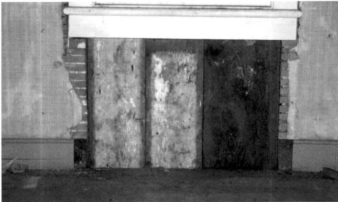
Fig. V-5. Opening in the east wall of Room 1 (E2) beneath the window showing evidence of modern reuse of what appears to be Military era whitewashed planks exhibiting the ghosts of former battens and perhaps molding. This was a former (c. 1925) doorway to Room E1, before restoration by the NPS. The planks were installed during the c. 1978 restoration. Photograph by Aaron Lemchen October 2005.
