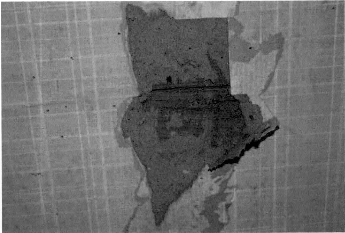
Fig. V-4. Opening in the south wall of Room 1 (E2) showing layers of heavy paperboard and wallpaper over horizontal wood planks. Photograph by Aaron Lemchen October 2005.
