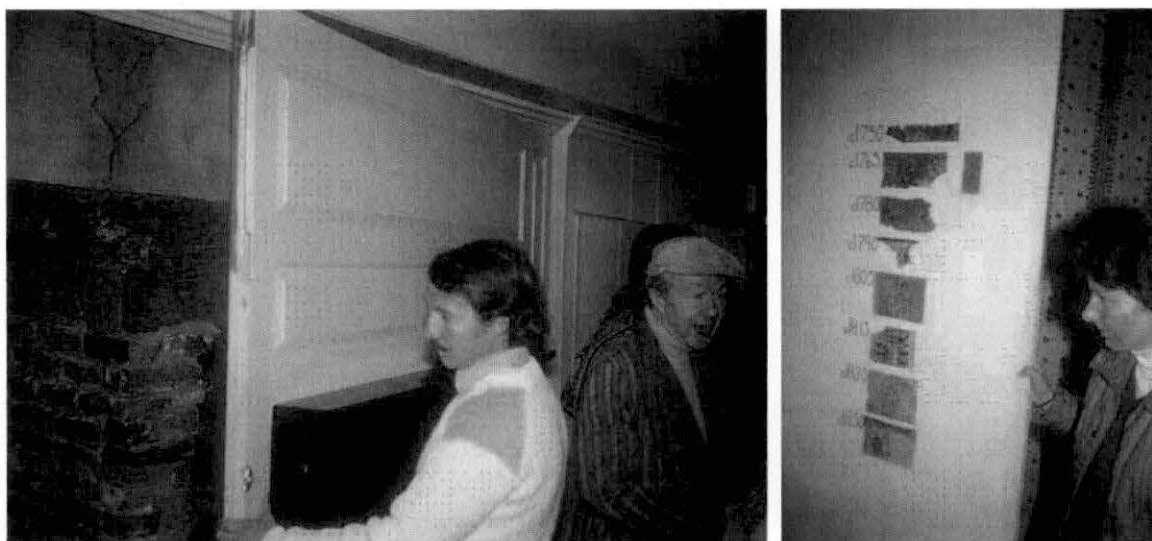
Fig. VII-1. Left: The late eighteenth century raised paneling is mounted on piano hinges and operated here by Professor Patrick Malone of Brown University, revealing the early eighteenth century historic hearth in the Parson Barnard House, North Andover, Massachusetts (c.1715). Abbott Lowell Cummings of Yale University is to his right interpreting the site's preservation approach to members of the Vernacular Architectural Forum. Right: another door in the same room is opened by an unnamed person in the "study house" and reveals a chronology of the wallpaper patterns within the house. Photographs courtesy of Dr. Kingston W. Heath, 1981.
