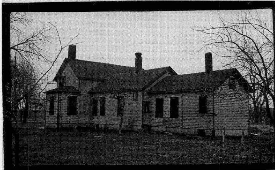
Fig. II-8. 1937 HABS photograph of "General Grant's Headquarters" (c.1849), Vancouver Barracks, Fort Vancouver, Vancouver, Washington. Quarter view of the rear.
