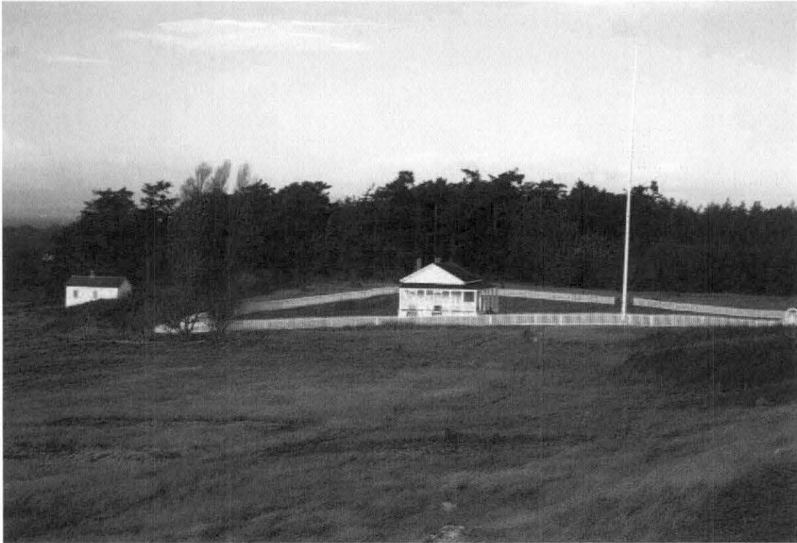
Fig. VI-2. View of HS-11 after its exterior restoration. Photo by Aaron Lemchen, October, 2005.
