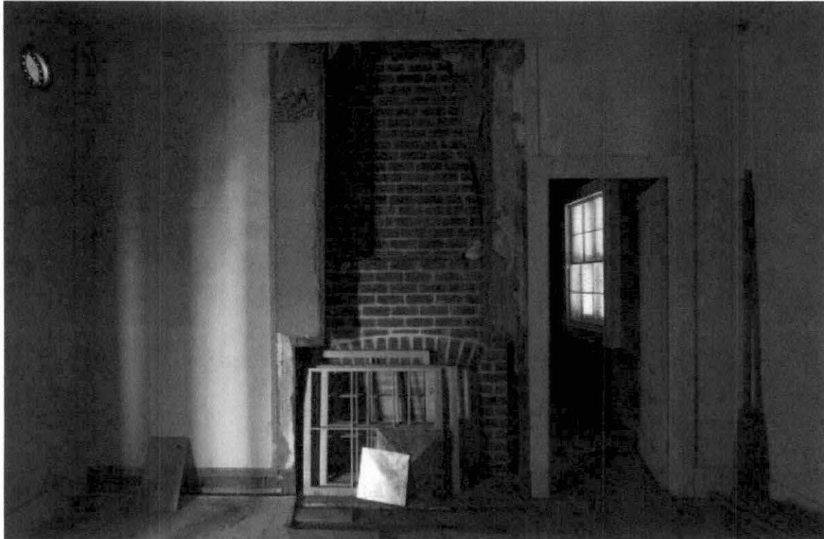
Fig. V-10. Room 3 (E7), south wall showing restored fireplace as well as the various layers of finishes. Photograph by Aaron Lemchen March 2005.
