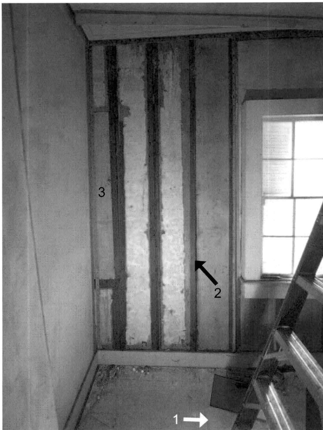
Fig. V-7. East wall of Room 2 (E5). Note the aligned butt joint and paint shadow in the floor boards at the bottom of the picture (1). Also note its alignment with the paint shadow on the vertical structural planks, which also appear to have shadows in the paint and wallpaper from previous battens (2). This suggests the presence of an earlier wall division that ran on either side of the hearth. A patch where a window once was can be seen in the board at the leftmost section of the east wall in this picture. It was butted against by the north wall (3). This patch was likely an original window during the military or agricultural era. Photograph and image enhancement by Aaron Lemchen March and June 2005.
