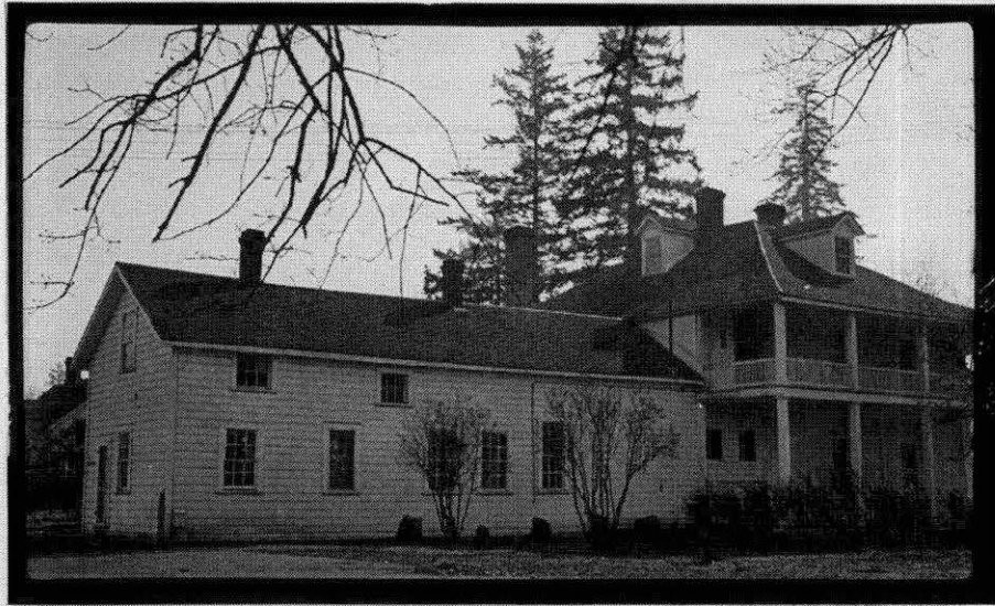
Fig. II-4. 1937 HABS photograph of Ulysses S. Grant House (c. 1849, Former Post Library & Officers' Club), Fort Vancouver Barracks, Washington. Quarterview of rear.
