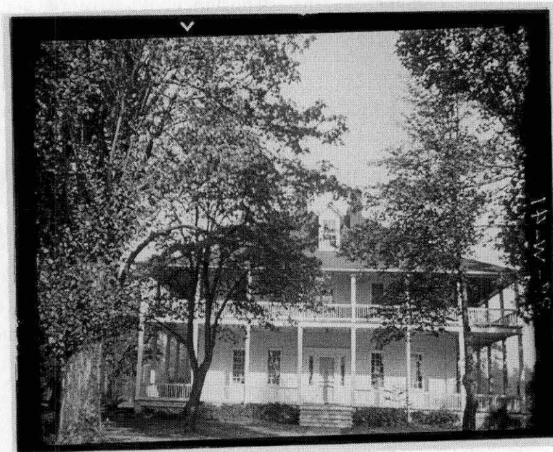
Fig. II-3. 1937 HABS photograph of Ulysses S. Grant House (c. 1849, former Post Library & Officers' Club), Fort Vancouver Barracks, Washington, Front.
