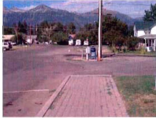
Figure 3-2: Existing utility poles and mailboxes could complicate sidewalk construction on W McCully Avenue near Main Street.
