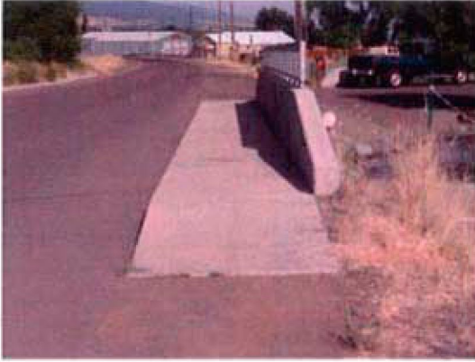
Figure 3-1: The W McCully Avenue bridge over Wrenn Dobbin Ditch includes a sidewalk on the north side.
