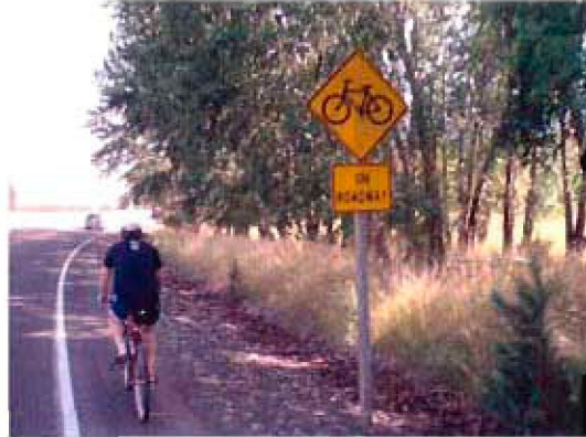
Figure 2-10: Warning signs on Wallowa Lake Highway alert motorists of bicyclists on the roadway.
