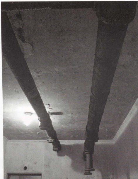
Historic Structure Report — Photographic Documentation
