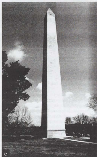
Figure 20. (a) The Jefferson Davis Memorial in Fairview, Kentucky, constructed from 1917–1924, is 351 feet tall and constructed of unreinforced concrete. The walls of the memorial are 8 feet thick at the base and 2 feet thick at the top of the wall. Access to the monument for investigation was provided by rappelling techniques, while ground supported and suspended scaffolding was used to access the exterior during repairs. (b) The concrete was severely deteriorated at isolated locations, with spalling and damage from cyclic freezing and thawing of entrapped water. In addition, previous repairs were at the end of their service life and removal of deteriorated concrete and failed previous repairs was required. Light duty chipping hammers were used to avoid damage to adjacent material when removing deteriorated concrete to the level of sound concrete. (c) Field samples were performed to match the color, finish, and texture of the original concrete. A challenge in matching of historic concrete is achieving variability of appearance. (d) The completed surface after repairs exhibits intentional variability of the concrete surface to match the appearance of the original concrete. Some formwork imperfections that would normally be removed by finishing were intentionally left in place, to replicate the highly variable finish of the original concrete. (e) The Jefferson Davis Memorial after completion of repairs in 2004. Photo ©: Joseph Lenzi, Senler, Campbell & Associates, Inc.
