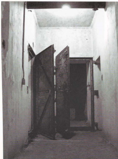
Photo 41. (Above). Gas-proof doors leading straight ahead into dormitory and left into west airlock.
