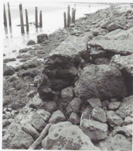
Photos 86-88. (Above and left). Various views of cable protective apron remains. Parts of the cable housing probably date from the first 1911 casemate on this site. A 1944 project added a more secure cable entry point.
