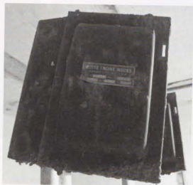
Photos 78, 79 (Above & top center). Views of the control box interiors. These boxes, along with the mine cables, are the only casemate electrical equipment left in place. No additional equipment was found during the clean-up in September 2008.
