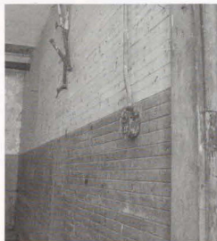
Photo 65. (Above). Several layers of historic paint are visible on the beadboard east partition wall of the dormitory.
