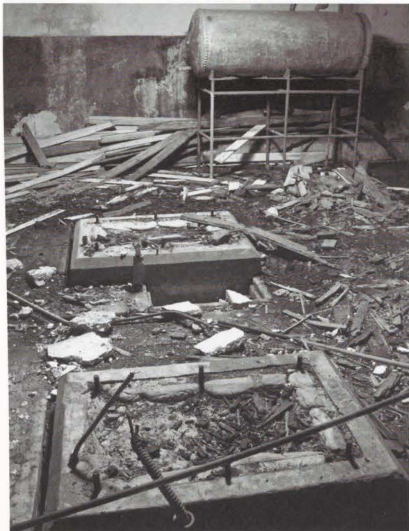
Photo 80. (Above). Concrete bases for engine and generator in front of engine room fuel oil tank. Base in the foreground held the belt driven generator that was powered by the engine.
