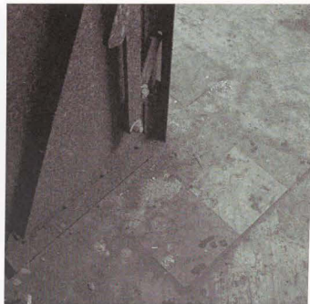
Photo 19. (Above). Steel plotting room door with frame cast in place. Form board impressions on wall. Door reveal is four feet thick in this spot. One foot abutting tunnel is original tunnel wall from 1941-43 building phase. Plotting room wall is three feet thick added in 1944-45. Construction joint where cap has been placed is visible at left of photo.
