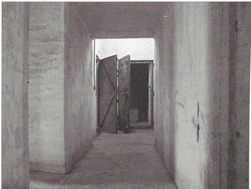
Photo 9. (Above) Looking east from the manhole area in the west tunnel. Door frames have been cast in place throughout the casemate in testimony to the high quality of workmanship. This feature has the potential to create structural problems from steel jacking if corrosion causes expansion of steel elements.
