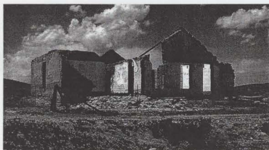
Figure 2. Chatterton House was the home of the post trader at Fort Fred Steel in Wyoming, one of several forts established in the 1860s to protect the Union Pacific Railroad. The walls of the post trader's house were built using stone aggregate and lime, without cement. The use of this material presents special preservation challenges.
