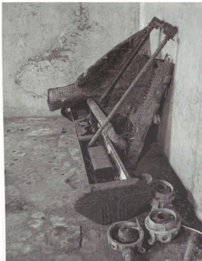
Photo 34. (Left). Light fixtures and acoustic ceiling tiles in corner of plotting room. Of main interest is the fluorescent tube fixture, an early example of this technology. This fixture should be retained and refurbished or used as a model to fabricate reproductions.
