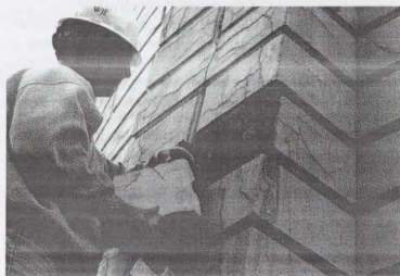
Figures 14. Layers of architectural concrete that have debonded (spalled) from the surface were removed from a historic water tank during the investigation performed to assess existing conditions. Photos: Anita Washko, Wiss, Janney, Elstner Associates, Inc.
