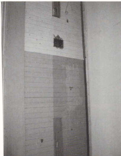
Photo 65. (Above). Several layers of historic paint are visible on the beadboard east partition wall of the dormitory.
