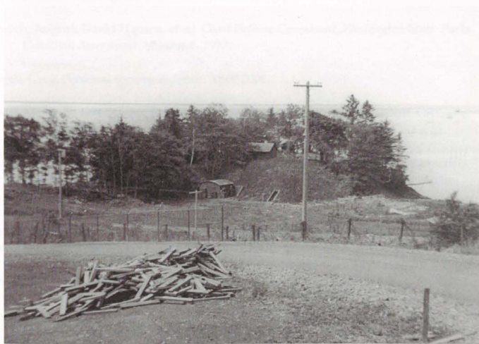
Below: Newly finished casemate. C.1945. Washington State Parks Photo.
