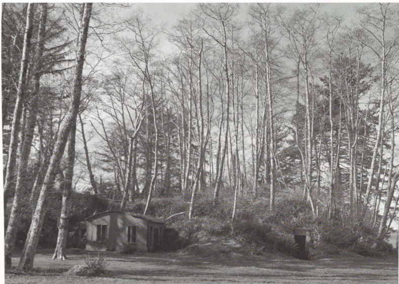
Photo 1. Looking south at Fort Columbia's new mine casemate. The west entry tunnel is seen on the right. On the left is the World War I era searchlight powerhouse, with the casemate's east gate just visible behind it to the left. The trees and native plants covering the earthwork were planted by the Army Corps of Engineers as part of the design of the fortification. The result is an intimate relationship between casemate and landscape. February 2008.
