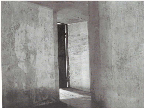
Photo 9. (Above) Looking east from the manhole area in the west tunnel. Door frames have been cast in place throughout the casemate in testimony to the high quality of workmanship. This feature has the potential to create structural problems from steel jacking if corrosion causes expansion of steel elements.
