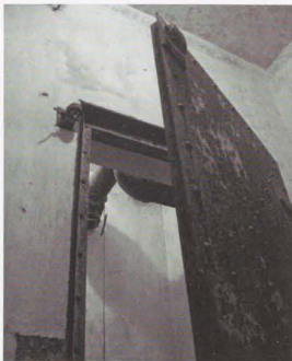
Photo 41. (Above). Gas-proof doors leading straight ahead into dormitory and left into west airlock.
