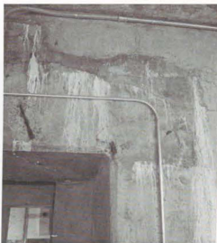
Photo 36. (Left). Detail of construction joint with efflorescence, plotting room south doorway, east side.
