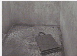
Photos 56-58. Views of gas-proofing apparatus in east air lock. Overhead pipes were connected to the air pumps and canisters on the other side of the wall. The chain hanging from the pipe in the photo at far left was connected to the pipe in the photo at far left was connected to the foot treadle below.
