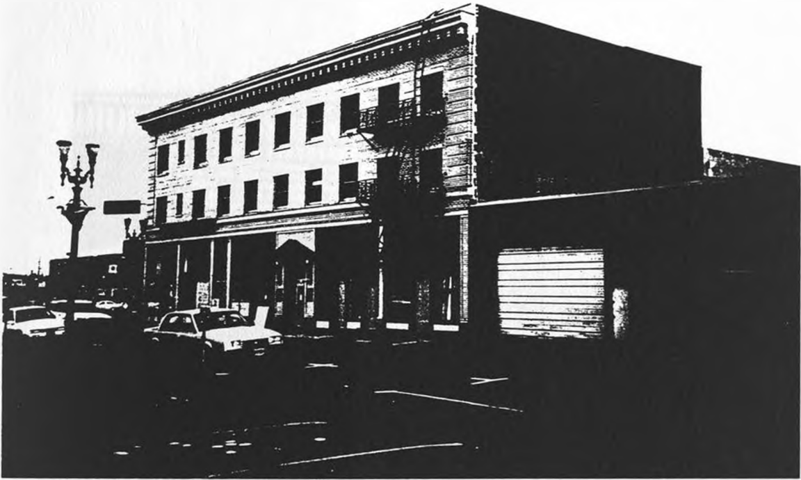
14. Photograph: North Facade of Royal Palms Hotel
