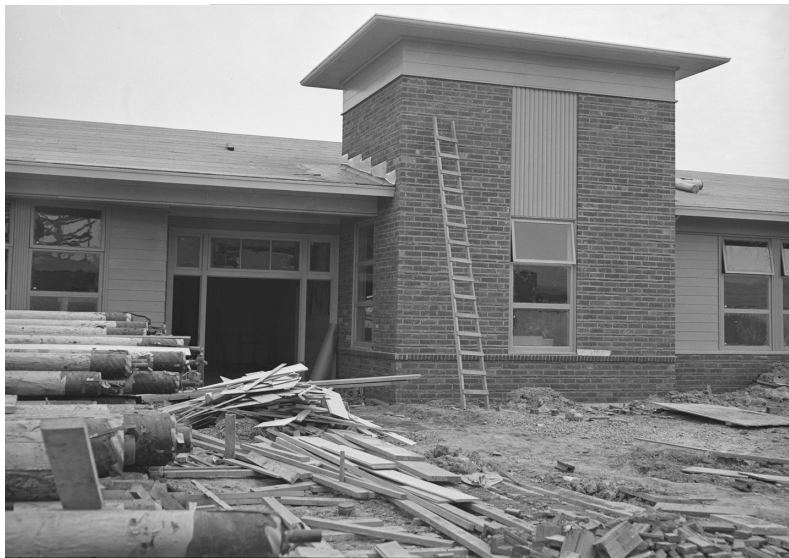
Construction of a school
