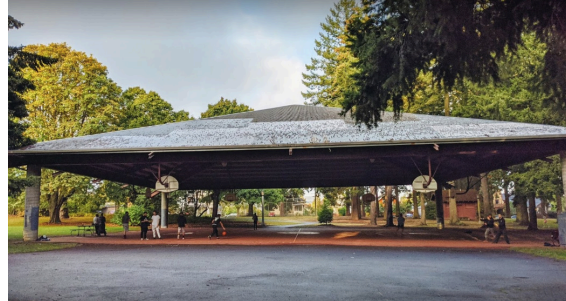
Covered Basketball Courts - Alberta Park PDX
