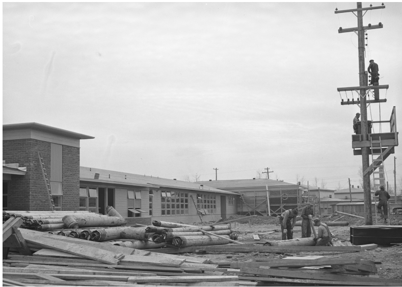
Construction of a school
