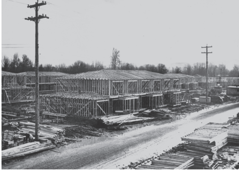
Construction of apartments
