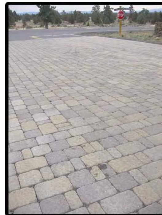
Decorative Intersection Pavers
