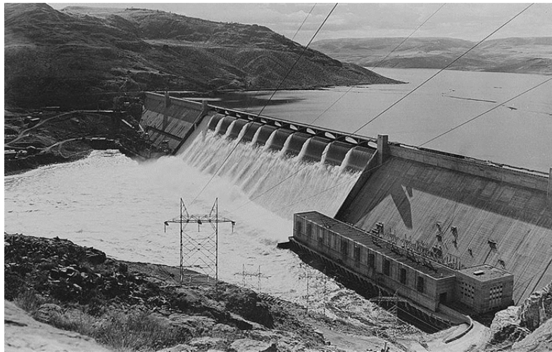
Figure 1: Grand Coulee Dam 1
