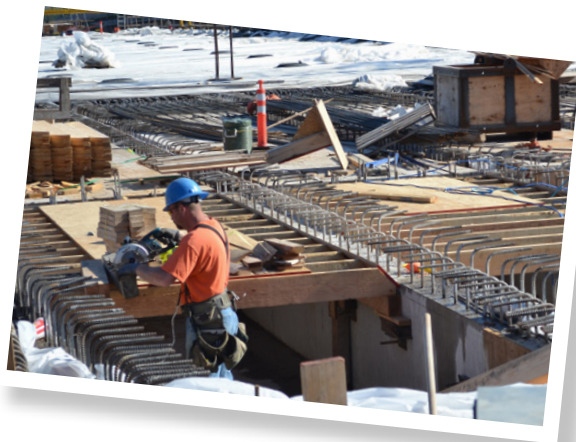
Completing framing of span 6 before deck pour.
