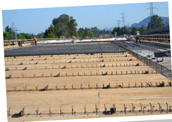
Finishing work before pouring deck from middle of river to south bank.
