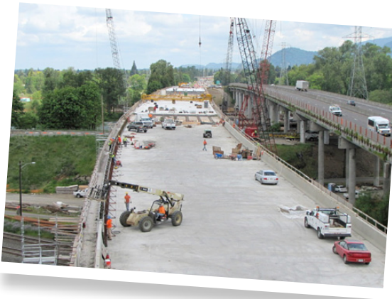
Finishing bridge deck and barriers, south end looking north.
