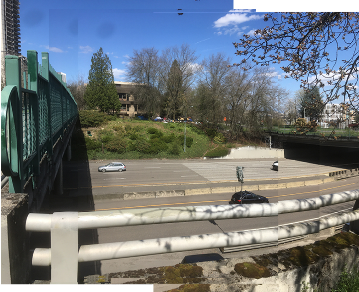
I-405 Underpass - Photo Collage
