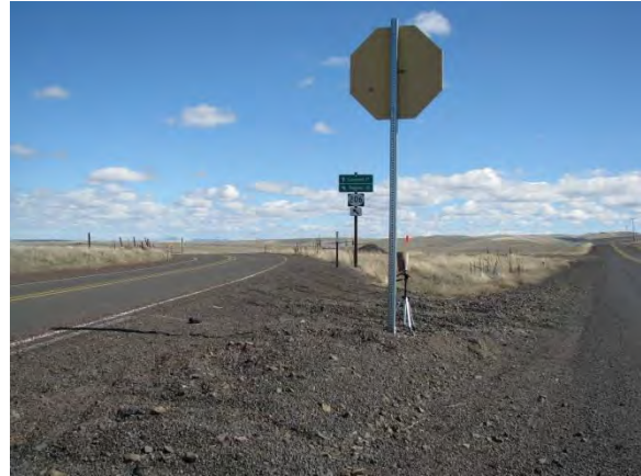
Exhibit 6-2. Restricted Sight Distance at OR 206/Lonerock Road
