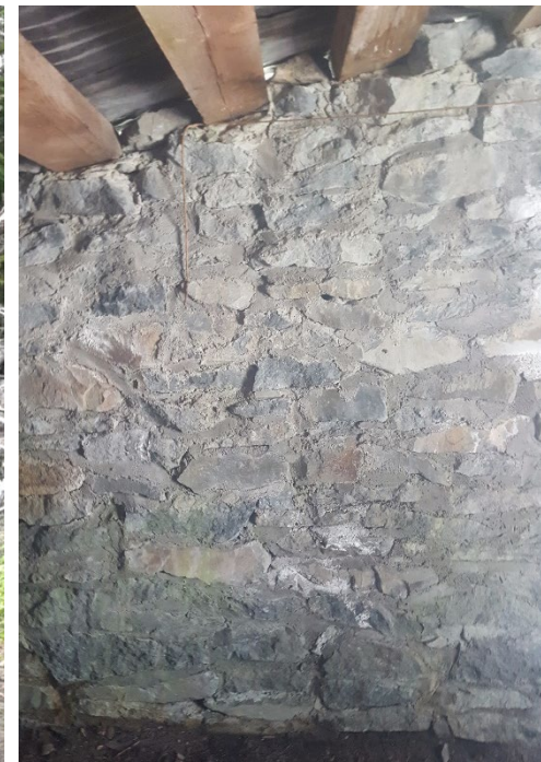
Typical interior construction and condition
