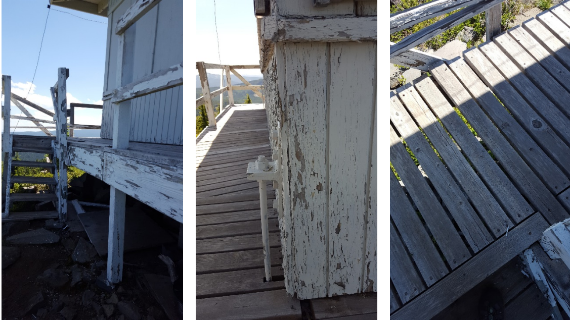
Figure 3. Photo tour of exterior features
