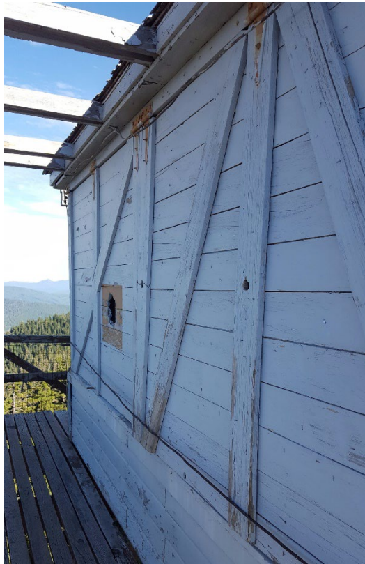
Typical condition, north elevation
