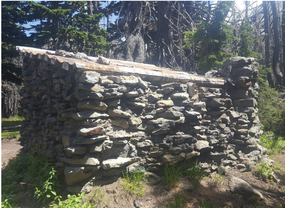
Rear elevation and chimney
