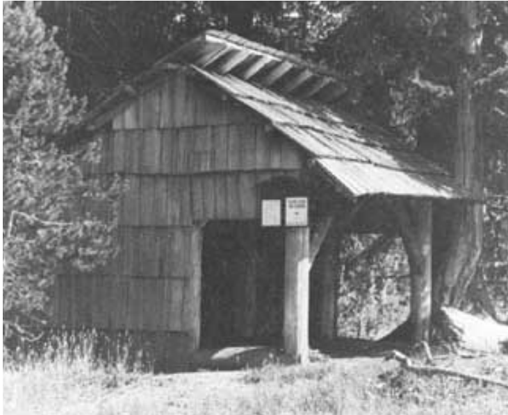
Construction and condition, 1978. Courtesy of USFS.
