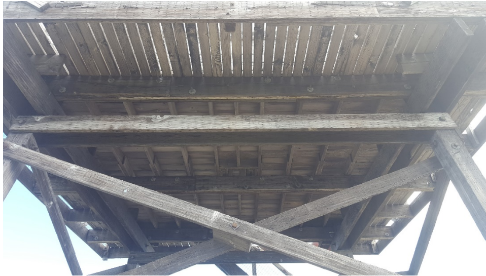
Tower and floor structure
