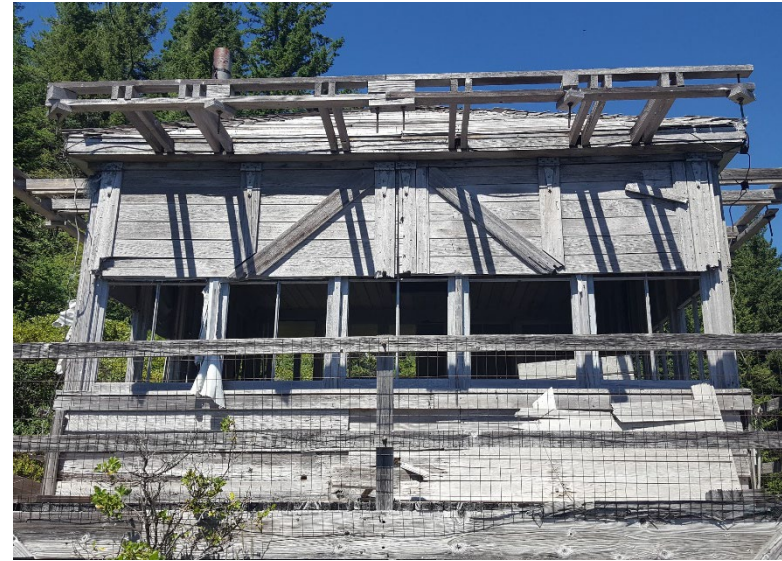
Typical condition, southwest elevation
