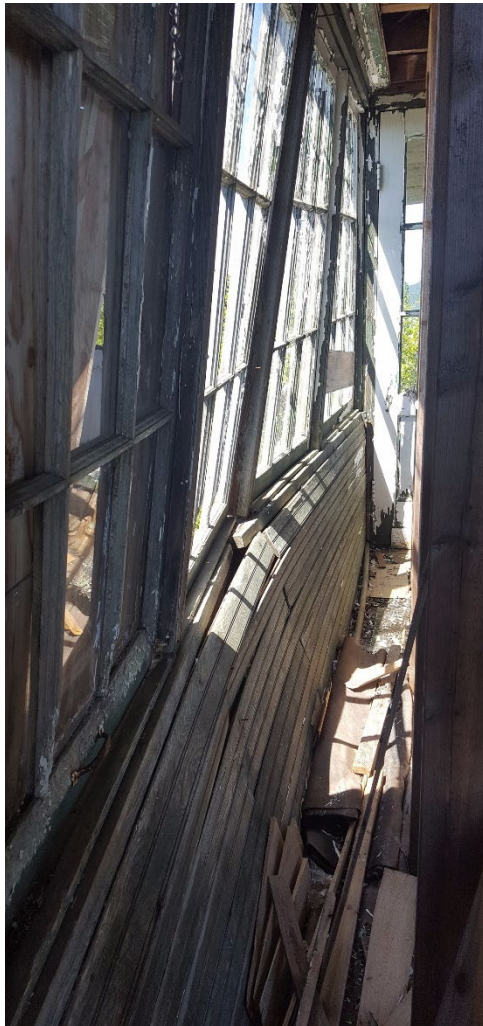
West wall interior
