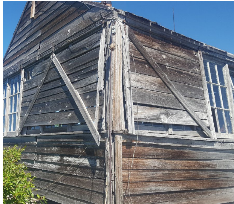
Typical condition of large and medium-sized shutters
