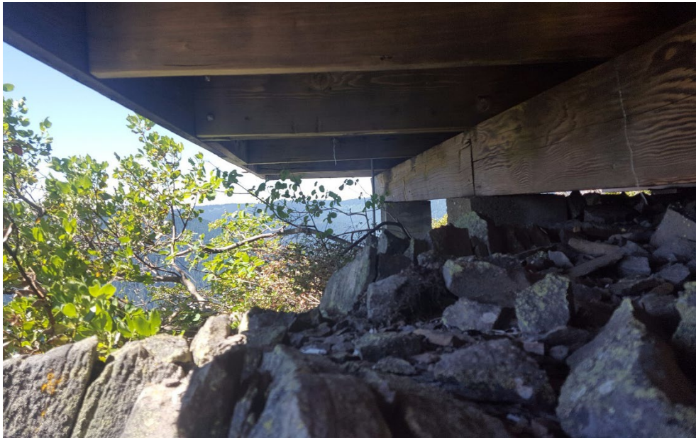
Typical construction and condition, southeast elevation
