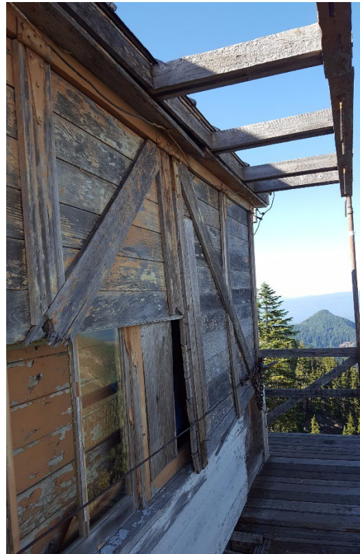
Typical condition, east elevation
