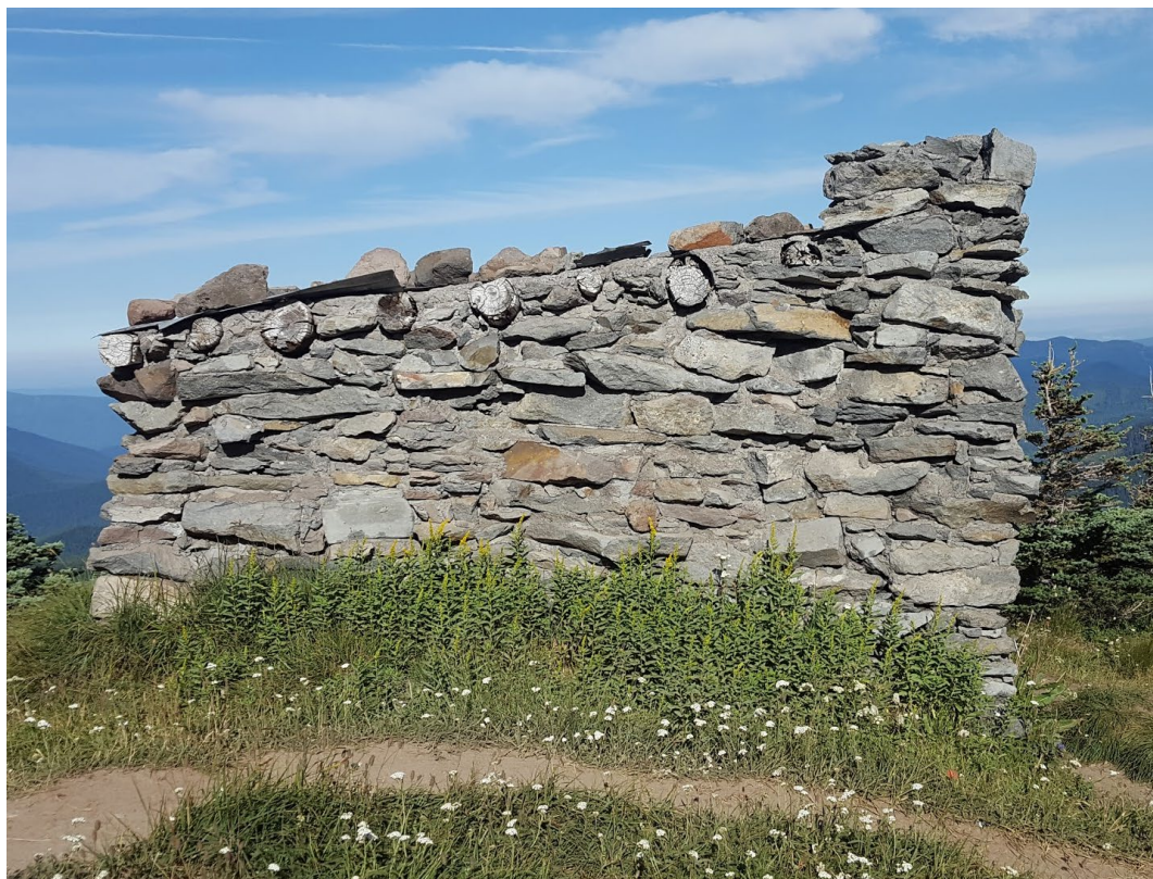
West elevation and chimney
