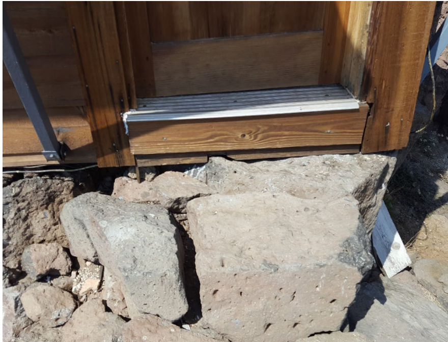
Typical construction and condition of dry-laid stone steps
