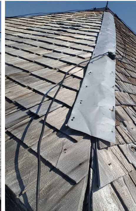
Shingled roof and flashed hip
