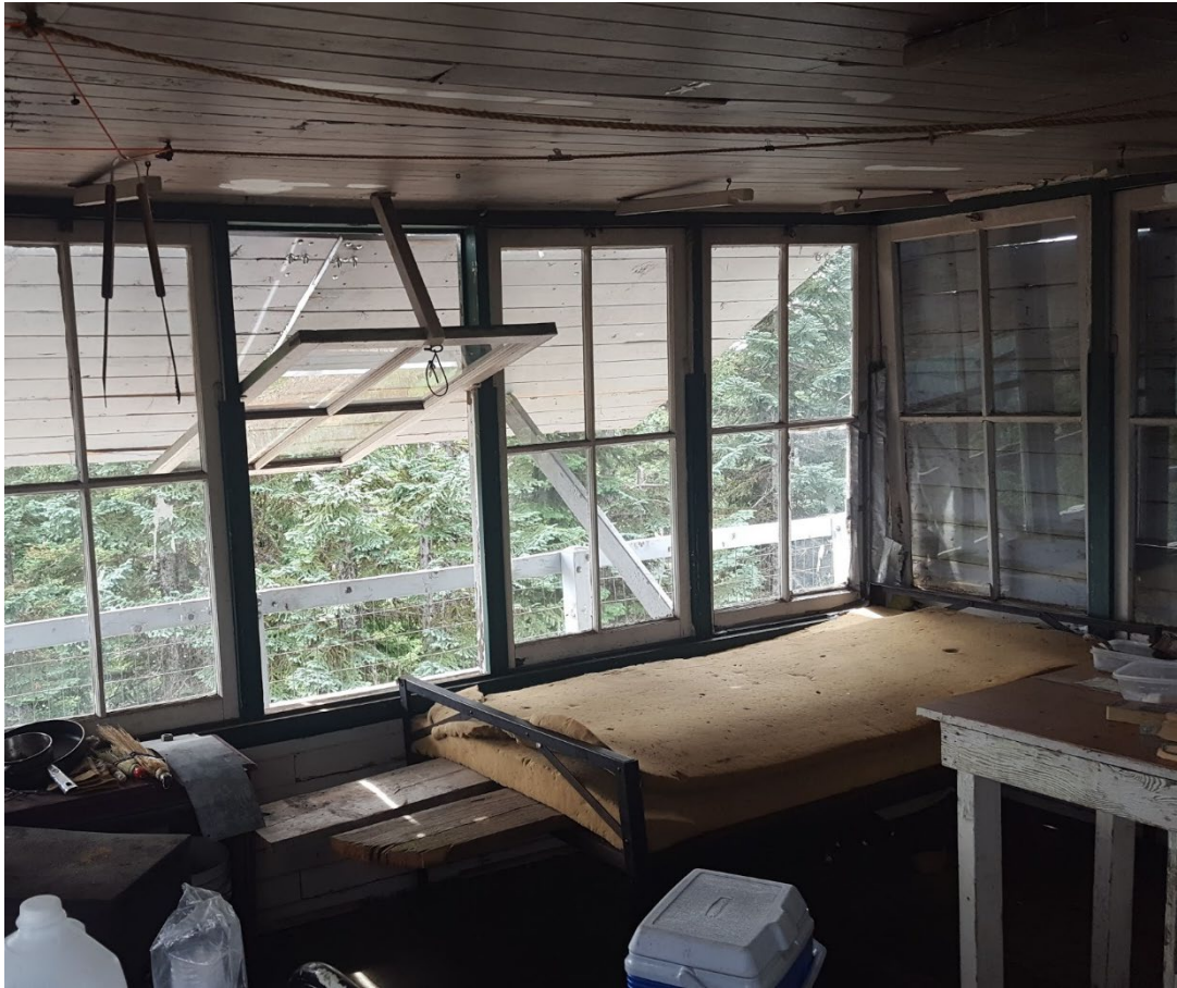
Typical window construction
