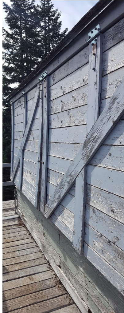
Condition of south shutters
