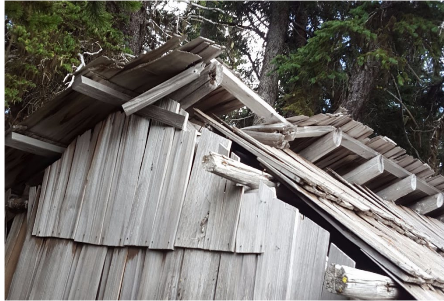
Roof construction and condition
