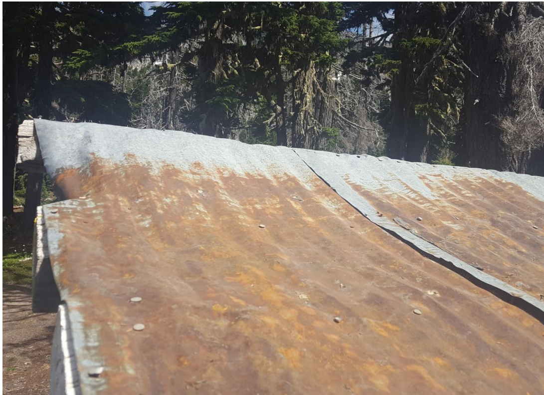
Typical roof construction and condition
