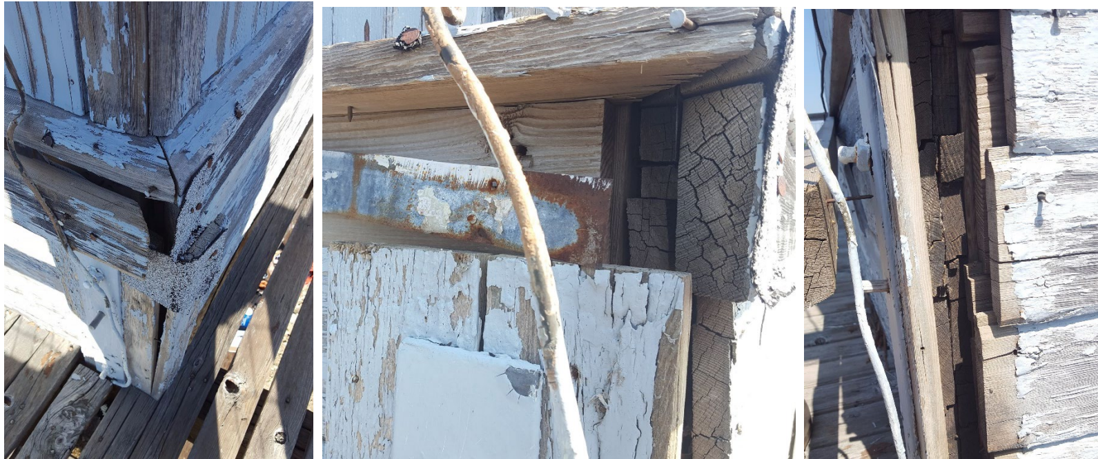
Condition at the southwest corner
