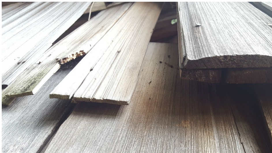
Shingles and shakes, south wall
