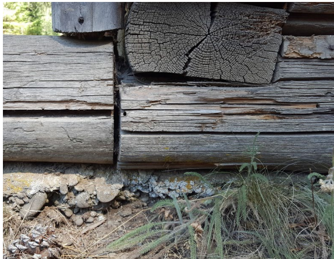
Foundation and sill construction
