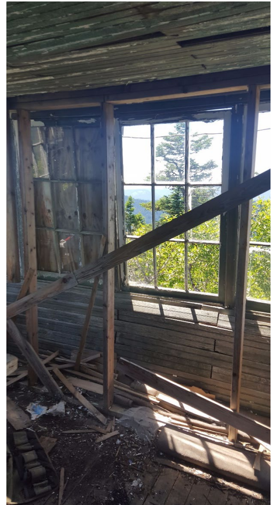
Temporary interior wall
