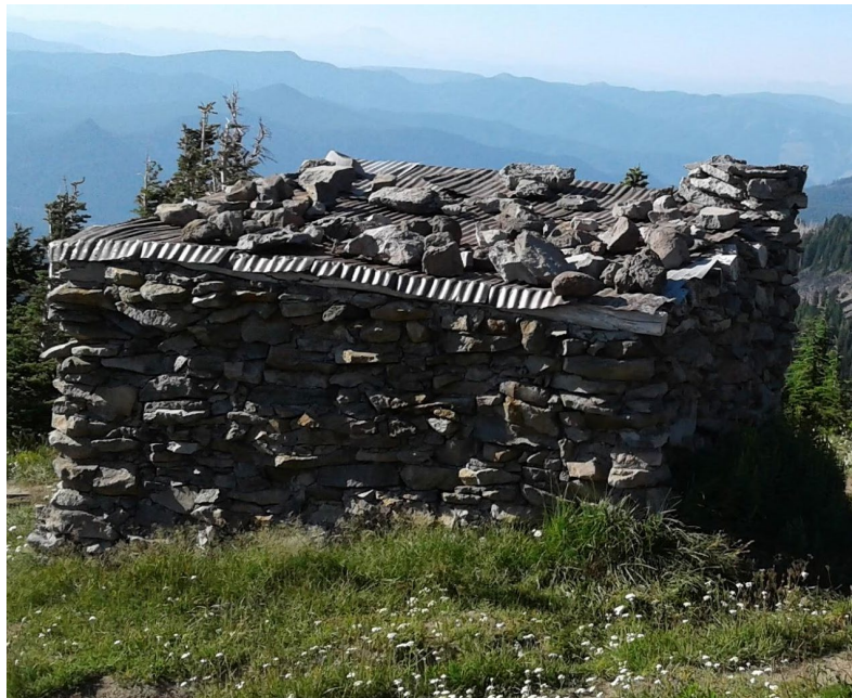
South elevation and roof construction. John Milliken.
