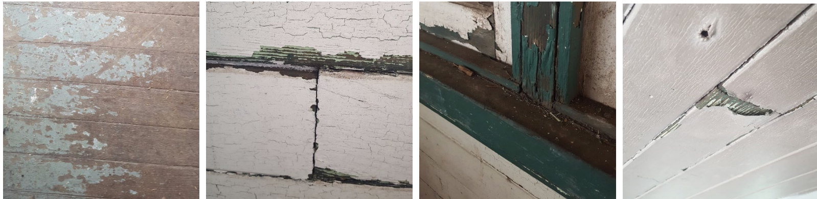
Typical condition of floor, walls, trim, and ceiling finishes
