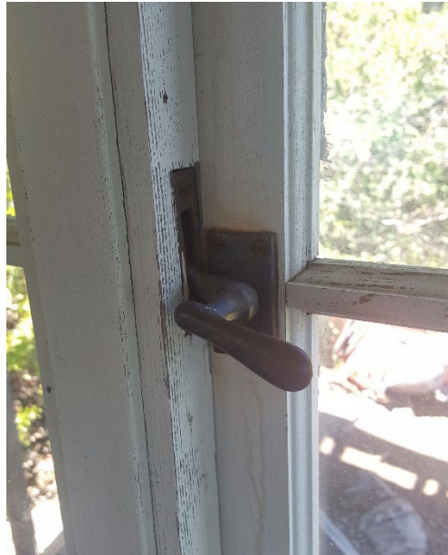
Interior sash and muntin profiles
