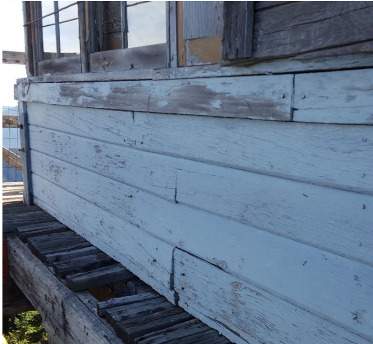
Typical wall condition
