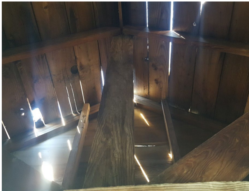
Roof structure construction and condition
