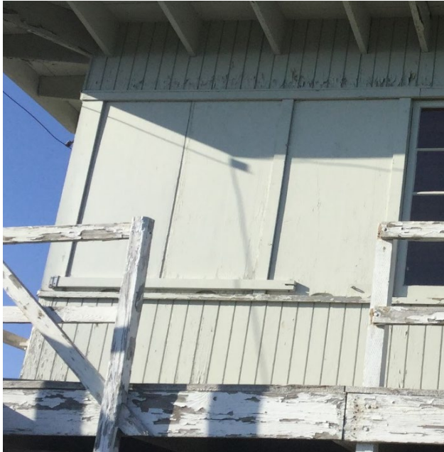
Typical shutter construction and condition
