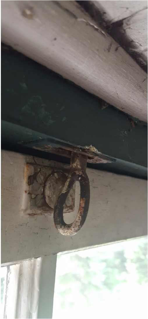
Typical condition, hardware
