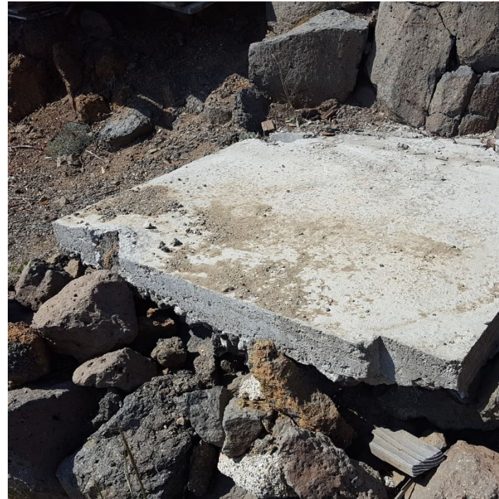
Concrete slab formerly used for propane storage
