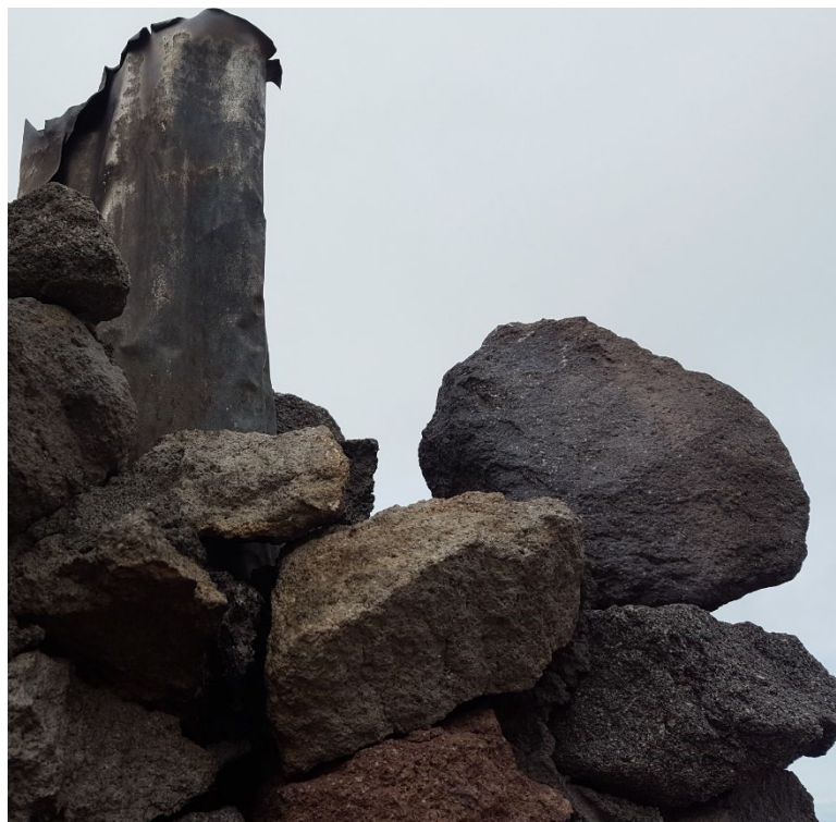
Corrugated steel stovepipe and loose stones
