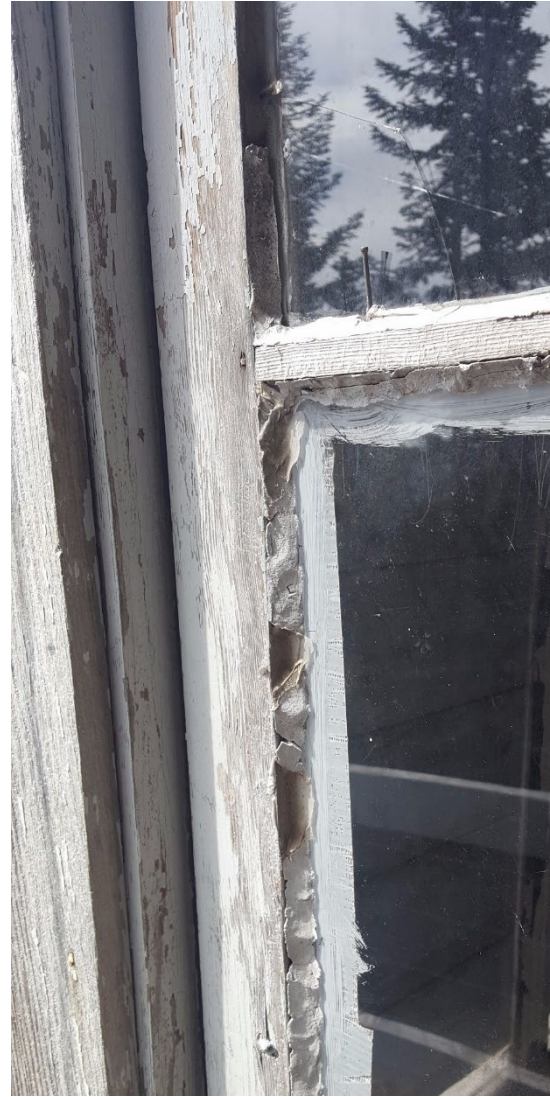
Typical condition, sash and glazing
