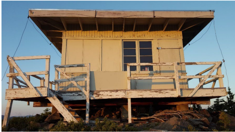
North elevation, railing design
