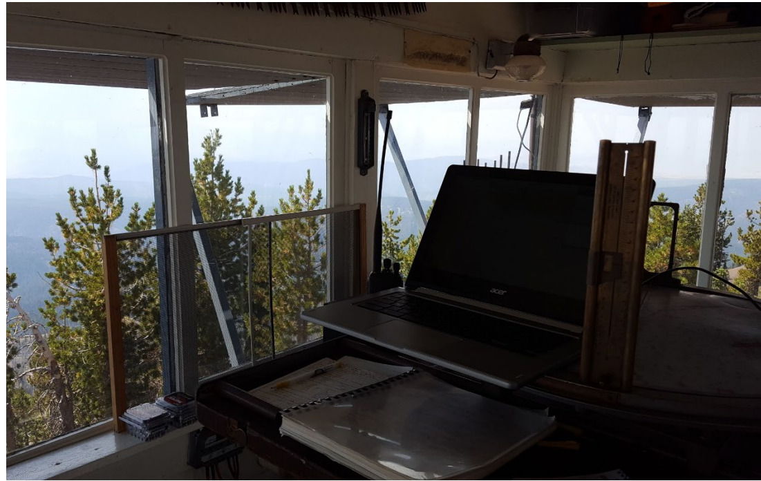
Construction of fixed and sliding sash
