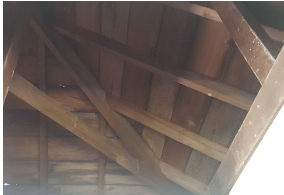
Roof construction and condition
