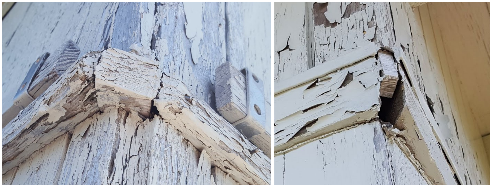
Typical construction and condition of trim below windows, above windows
