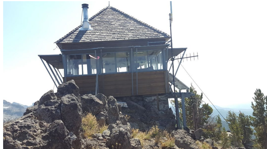
Northwest elevation and site
