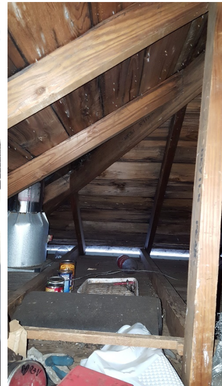
Typical condition, attic
