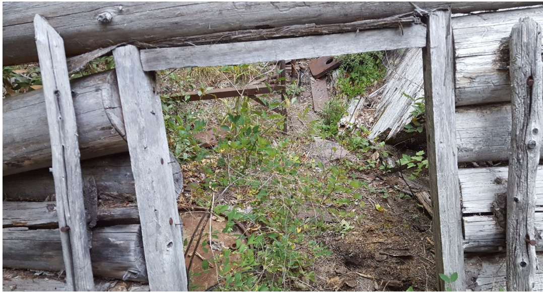
Window construction, east wall
