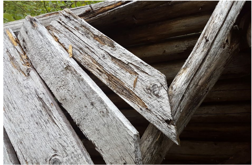
Board and batten construction, south wall
