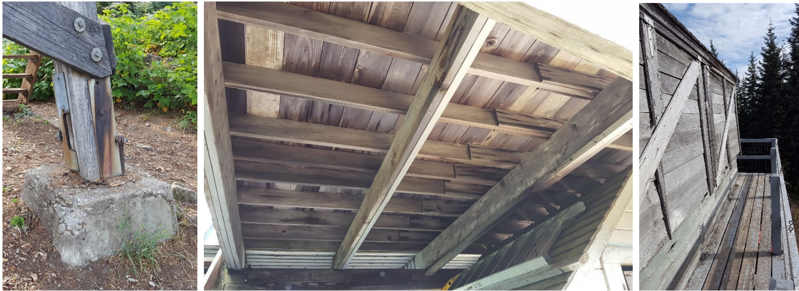
Typical construction and condition of footing, tower, floor structure, and catwalk
