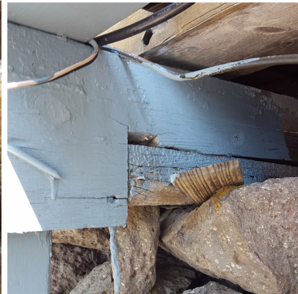
Typical rough construction of solar panel deck
