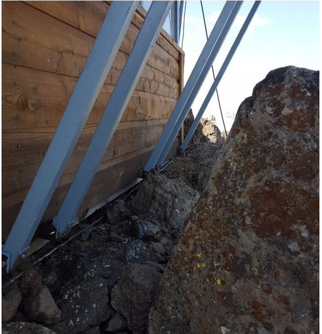
Basalt foundation, northeast side
