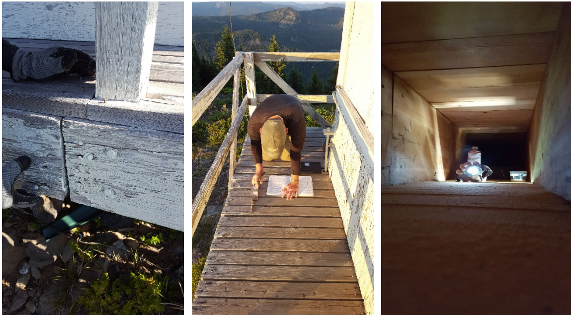
Figure 6. Crew members systematically assess architectural systems (Helmer, 2017)
