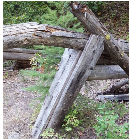
Doorway construction, west wall
