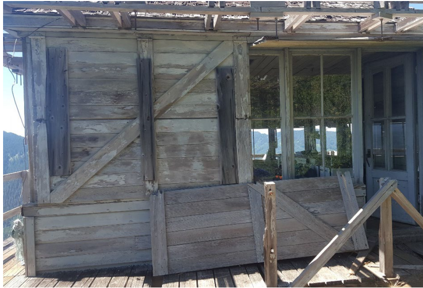
Typical construction (reinforced), northeast elevation
