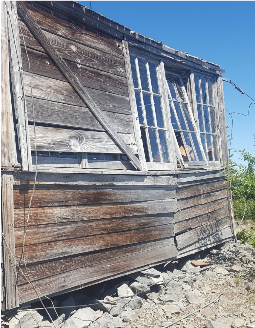
East wall condition
