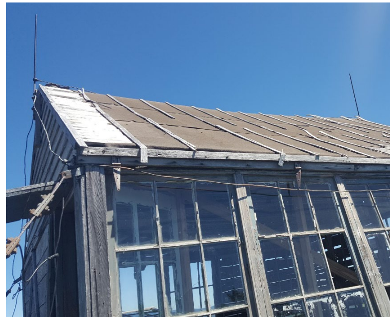
East roof condition
