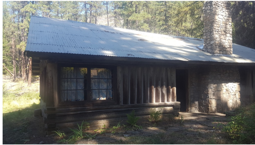
Red's Cabin: exterior
