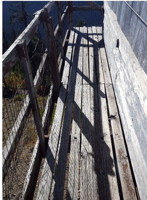
Deck condition, south side
