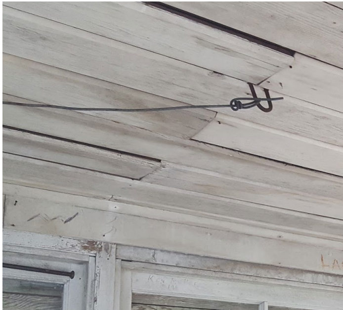
Typical ceiling construction and condition
