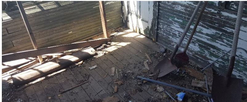
Floor and wall condition
