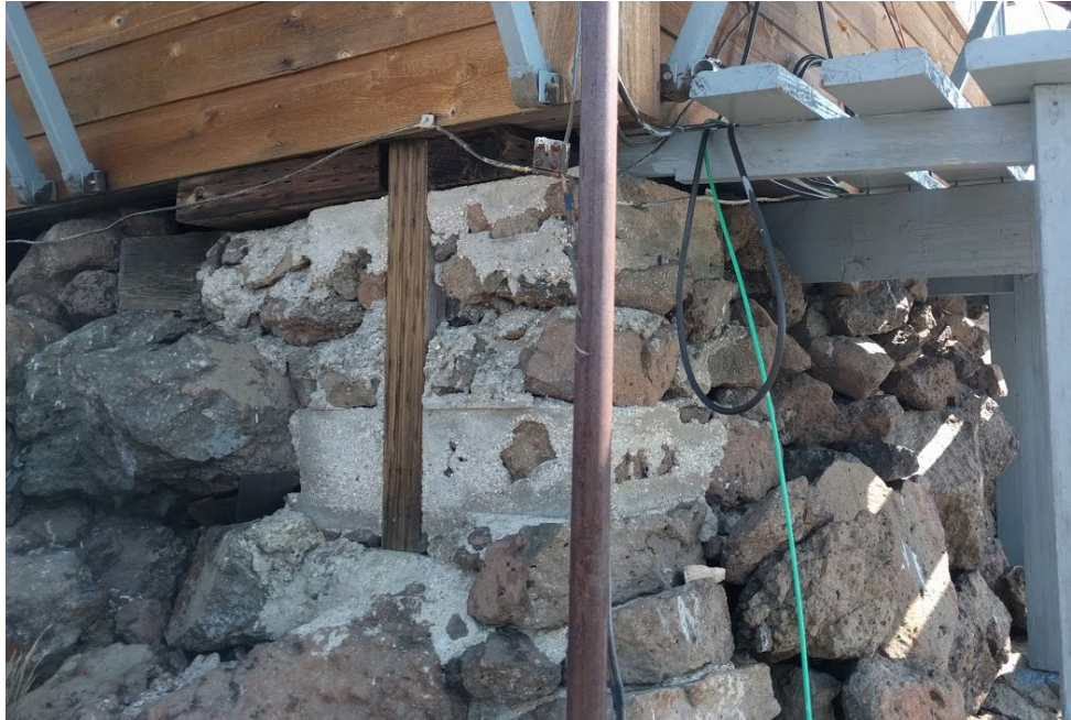
Reinforced foundation, west corner
