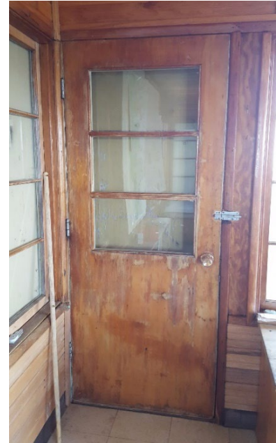
Door construction and condition
