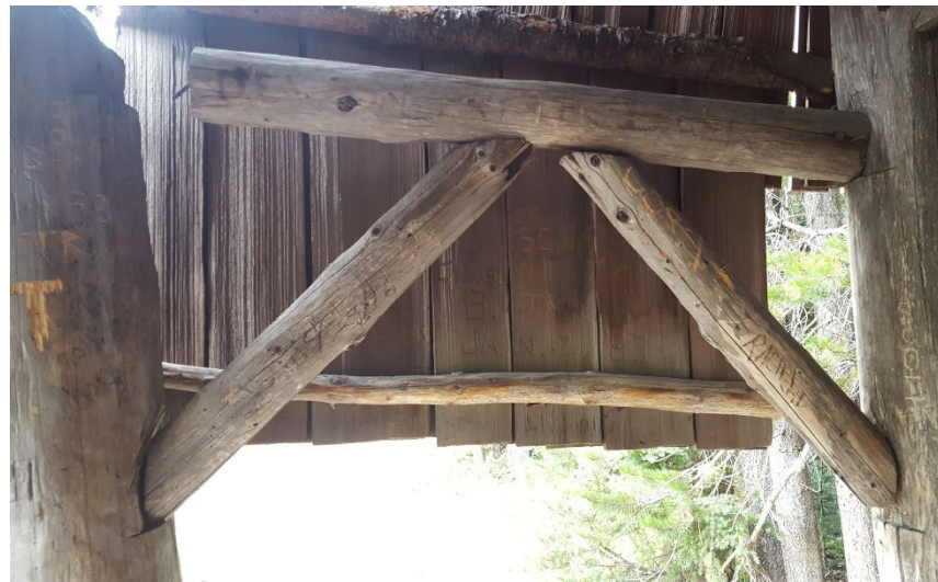
Condition of north wall braces
