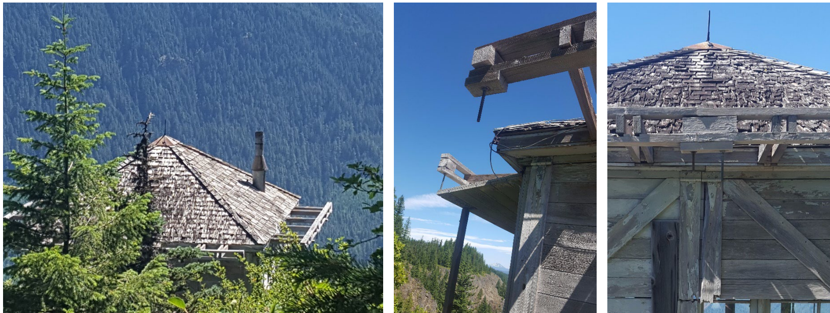
Typical construction and condition of external rafters and shingle roof.
