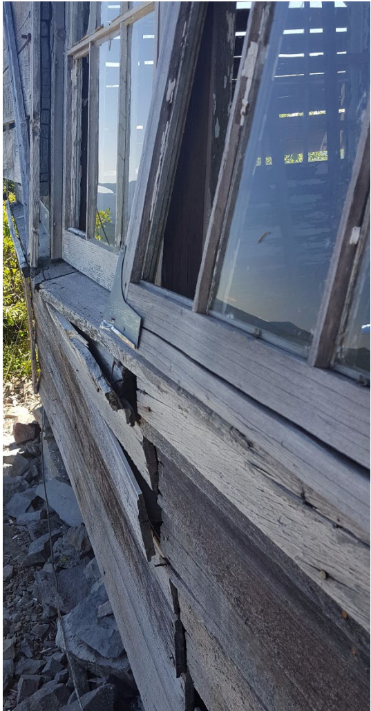
West wall exterior
