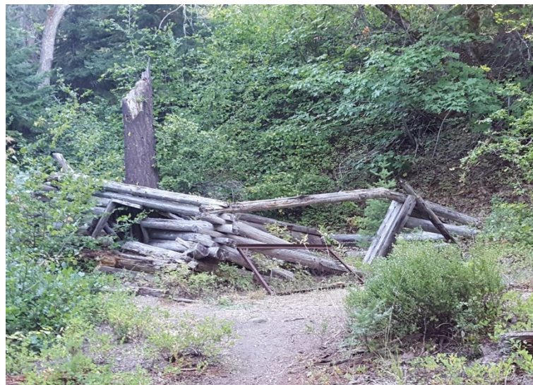
South and east elevations, 2017.
