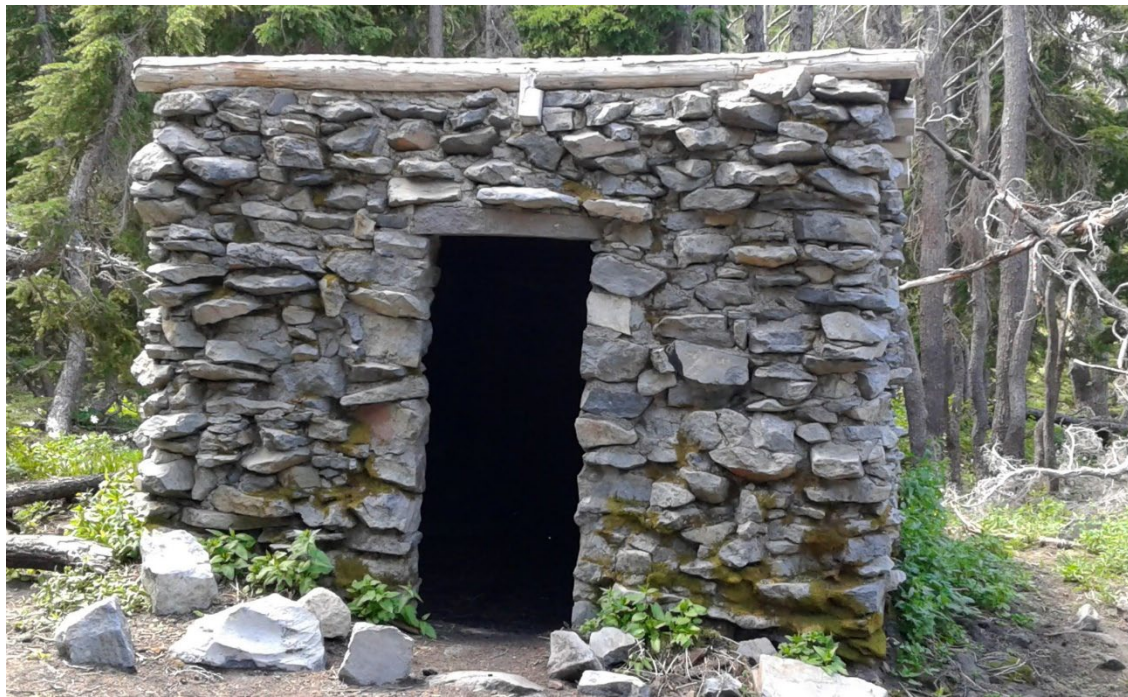
Typical wall construction and condition, north elevation
