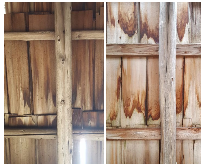
Roof construction: poles, replaced 2x4s, courses
