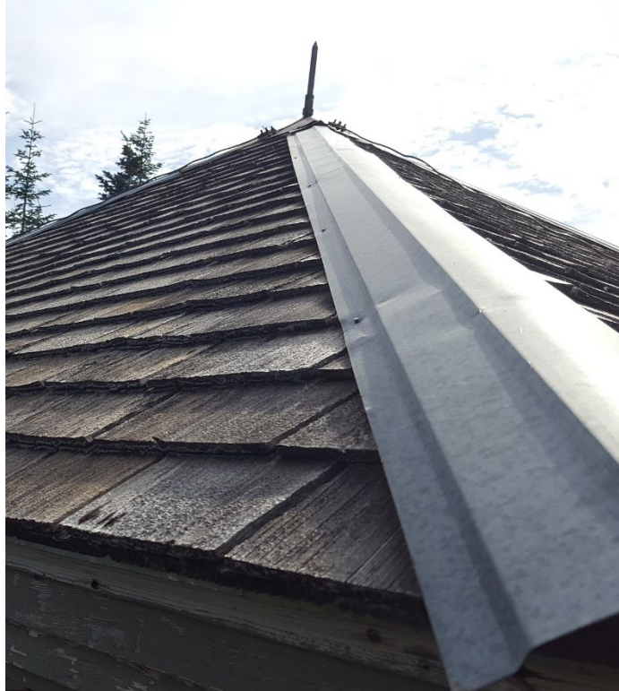
Typical condition, roof
