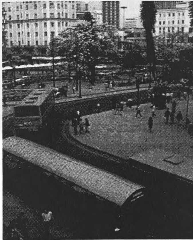
Bus tubes speed loading and unloading of busses in Curitiba, Brazil.
