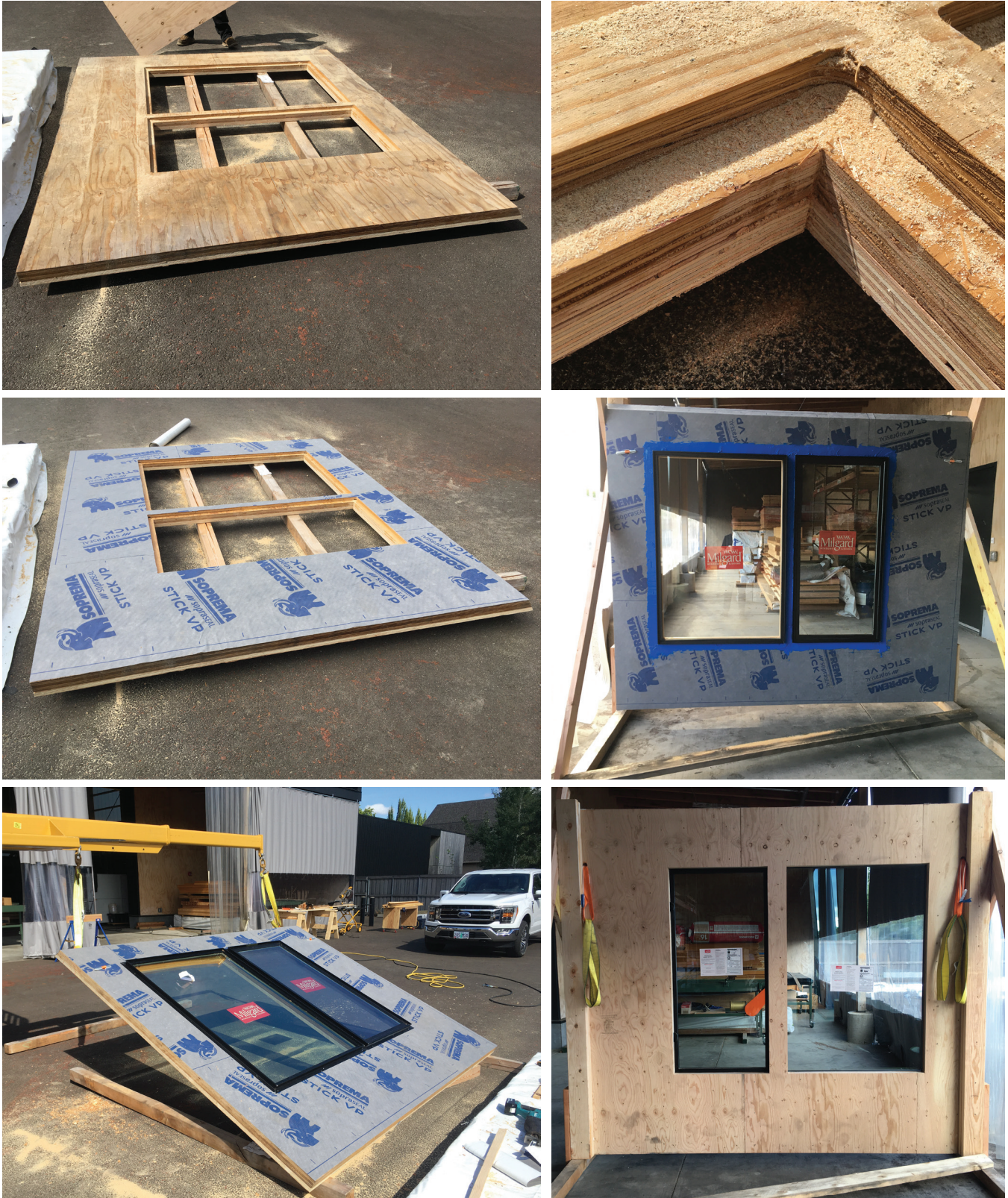
Figure 14: MPP window mock-up construction process photos
