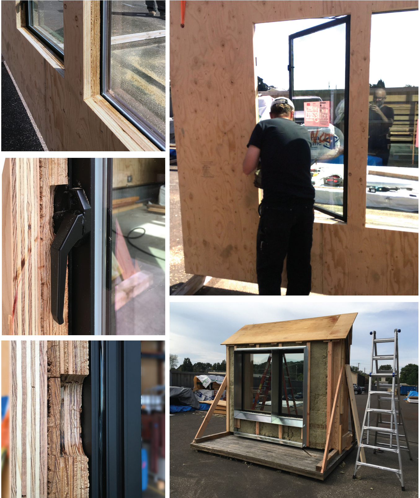
Figure 15: Window installation in MPP mock-up construction process photos
