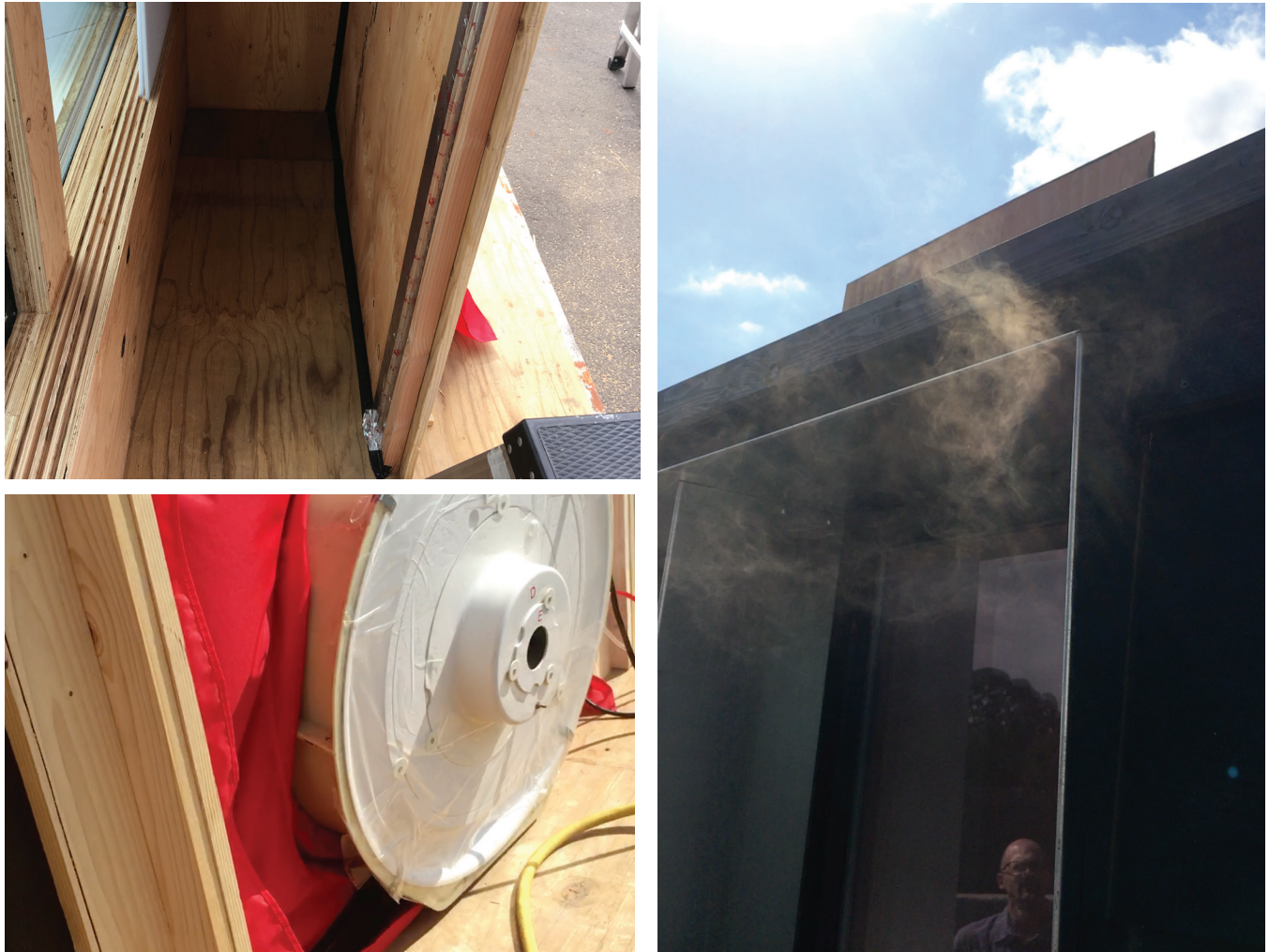
Figure 20: blower door testing and pressurized smoke testing photos
