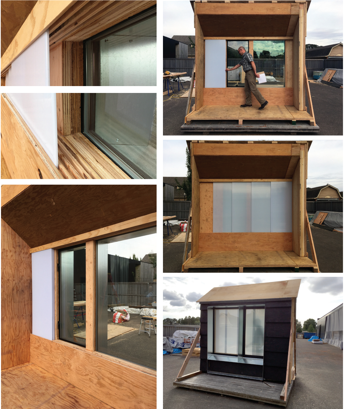
Figure 16: Completed MPP mock-up photos including polycarbonate energy shutter
