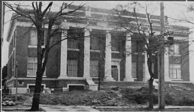
SKINNERS FROM THE ROOF OF VILLARU GRANDSTAND SEATS FOR COMMONWEALTH NEW ADMINISTRATION BUILDING NEARING COMPLETION
