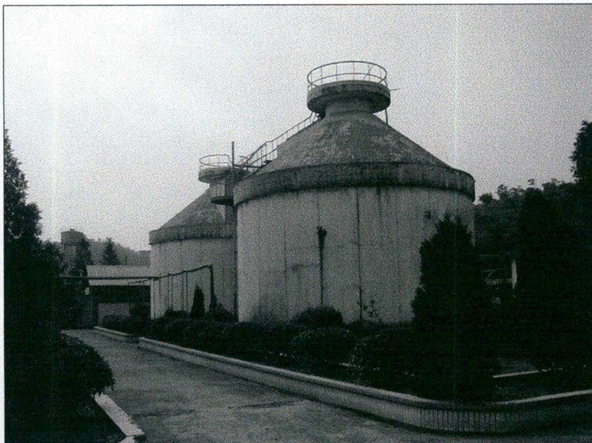
Figure 5. Biogas tanks in Fushan Village, Zhejiang
