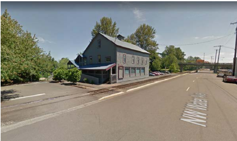
Figure 62: View west back down Water Avenue toward the Senior Center.
