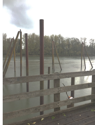
Existing Pilings near Monteith Park
