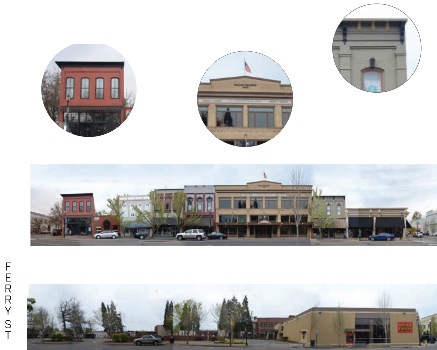
Figure 16: Façade details from Ferry Street to Broadalbin Street.
