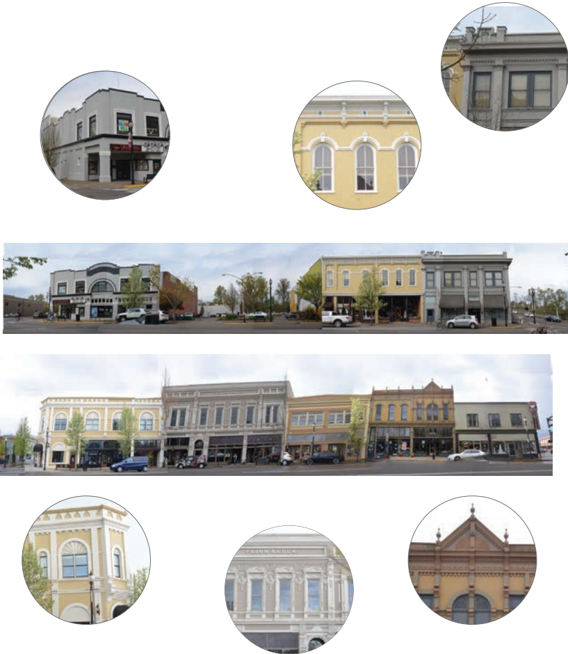
Figure 17: Façade details from Broadalbin Street to Ellsworth Street.
