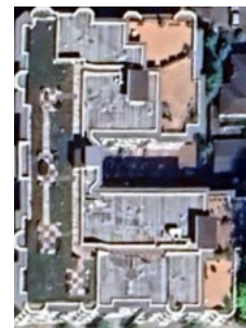
Figure 15: Seattle Post Development - Apartment Complex, April 2024
