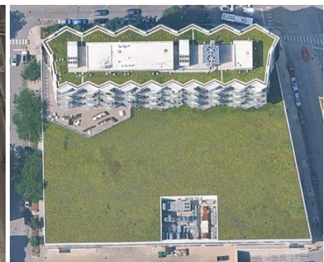
Figure 13: Chicago Post Development - Kenwood Site, May 2021
