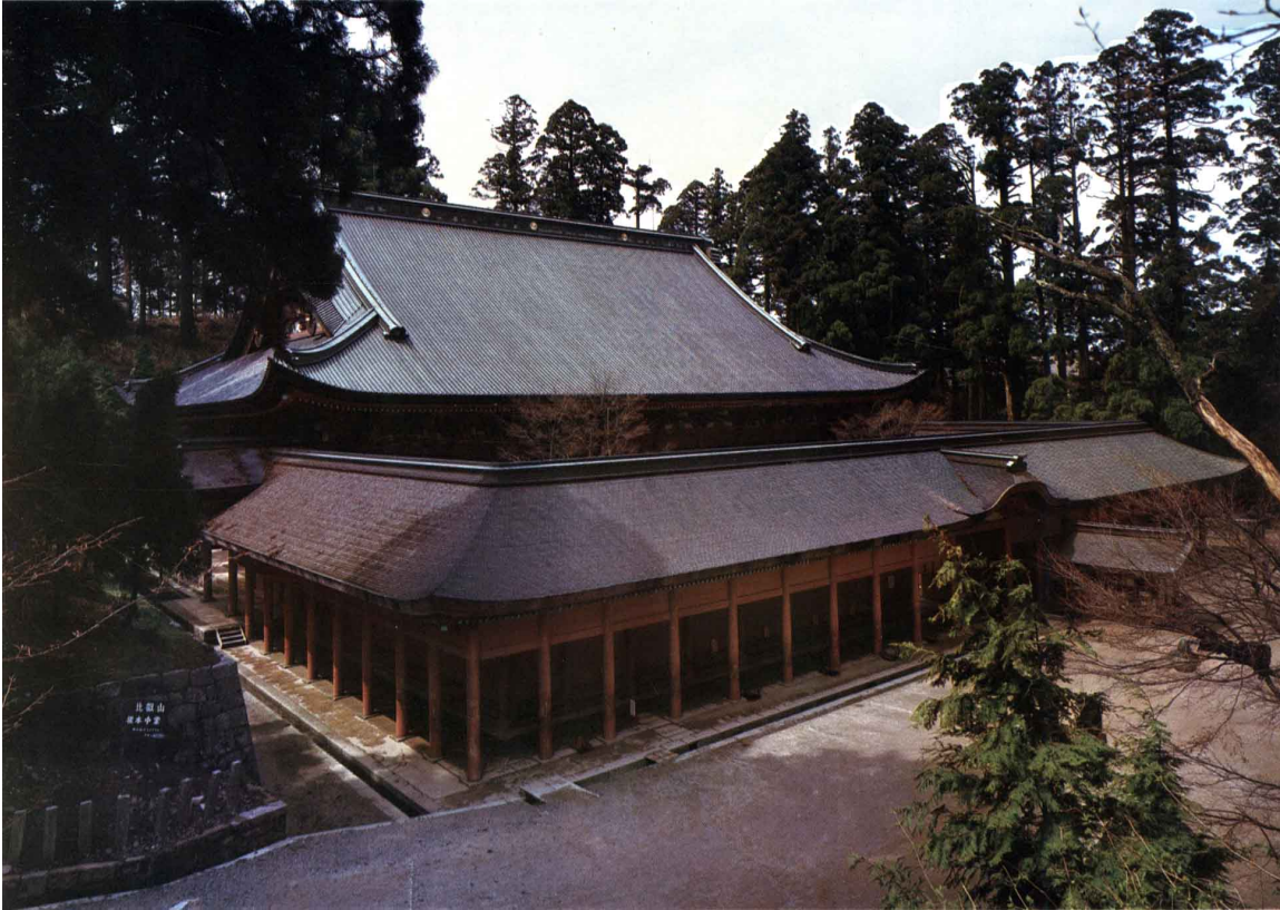
Figure 6. Central Hall of Enryakuji, Mt. Hiei, Shiga. (From Mikkyō jīin to Jōgan no chōkoku , 68)
