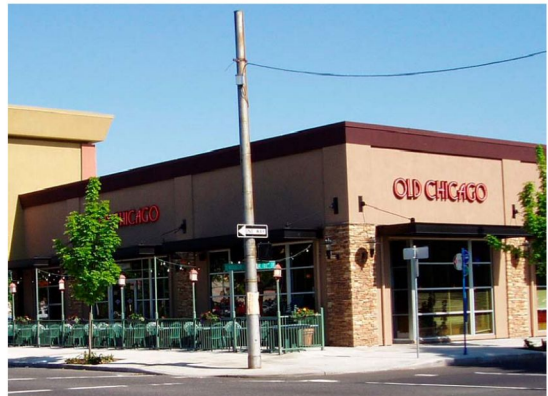
SE Washington at 103 d Avenue
