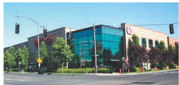
Corner Commercial Development
