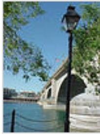
Picturesque Street Light Beside London Bridge , originally uploaded by mharrsch .
