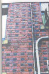
AIR CONDITIONER INTO SERVING PANTRY
