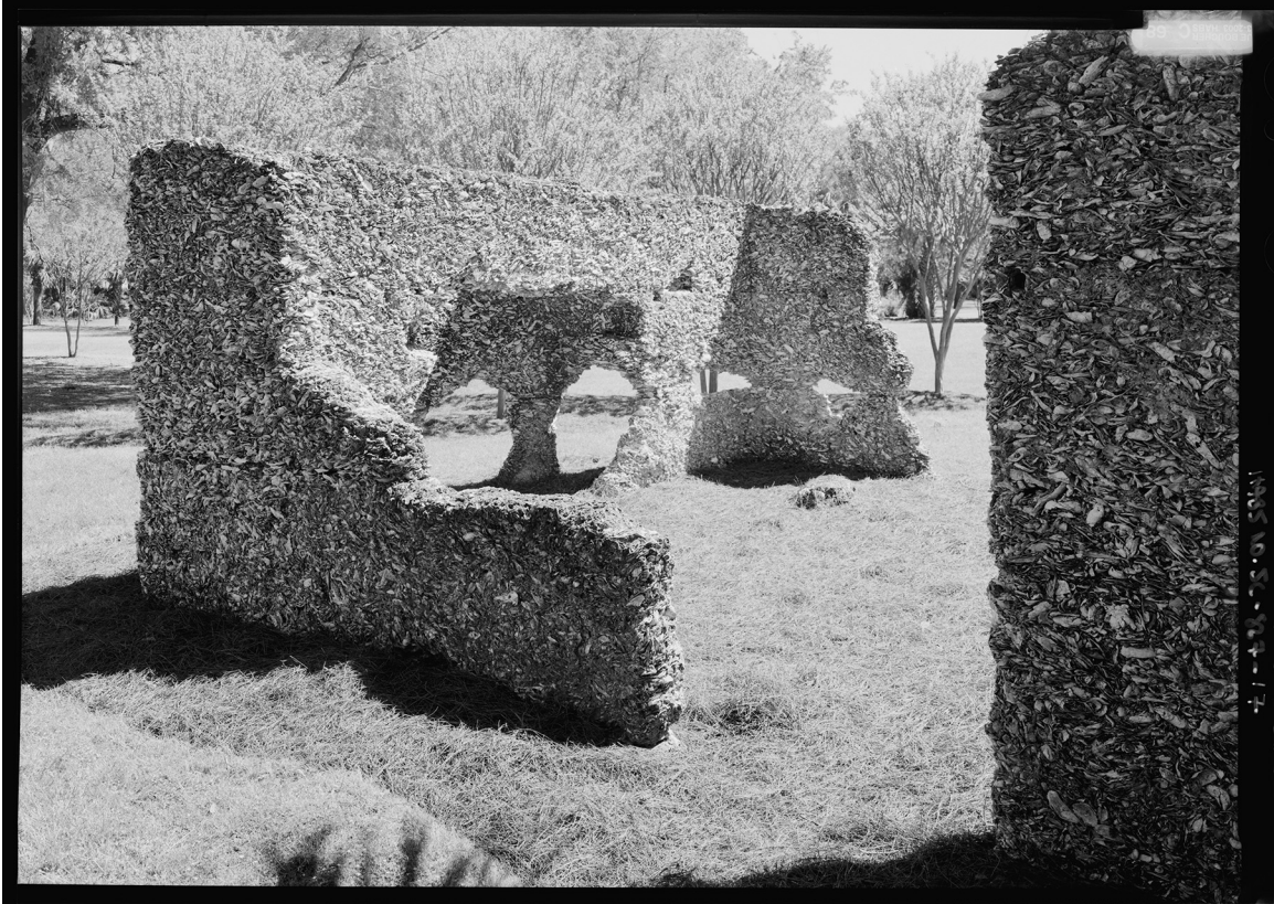
Fig. 11. Ruins of a tabby slave house at Haig Point. Library of Congress, Prints & Photographs Division, HABS SC-867.
