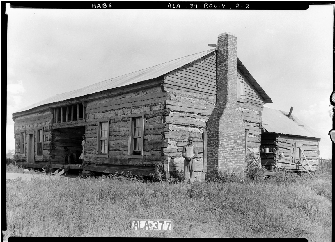
Fig. 42. Photograph showing the high quality of construction of the first Taylor-Cunningham House. Library of Congress, Prints & Photographs Division, HABS AL-377-A.
