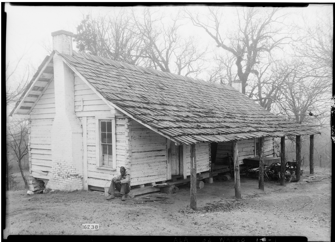
Fig. 26. Log slave house in Green County, Alabama with a strong notching system and white washed logs. The shake roof and double-hung windows were likely added later. Library of Congress, Prints & Photographs Division, HABS AL-238.
