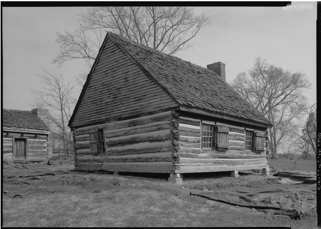
Fig. 17. West Cabin at The Hermitage. An example of a single-pen form type. Library of Congress, Prints & Photographs Division, HABS TN-52-A.
