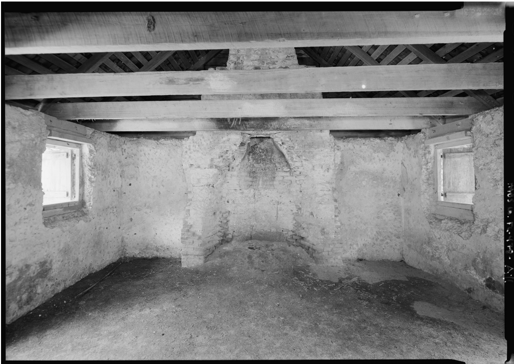
Fig. 9. Interior view of a slave house at Kingsley Plantation. Library of Congress, Prints & Photographs Division, HABS FL-478-A.
