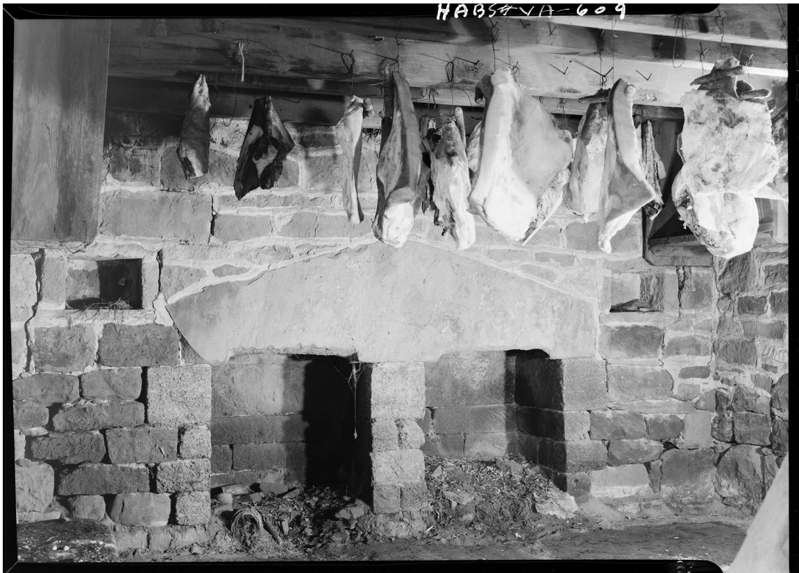
Fig. 32. Interior view of a slave house from Campbell County, Virginia showing the use of exposed ceiling joists to support meat hooks. Library of Congress, Prints & Photographs Division, HABS VA-609.
