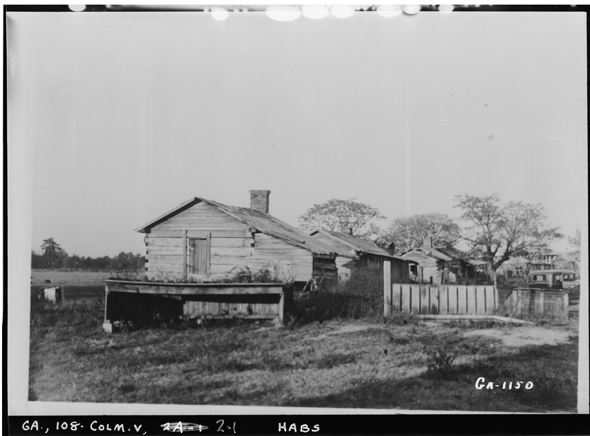
Fig. 50. Single-pen slave houses at the Bass Place. Library of Congress, Prints & Photographs Division, HABS GA-1150.
