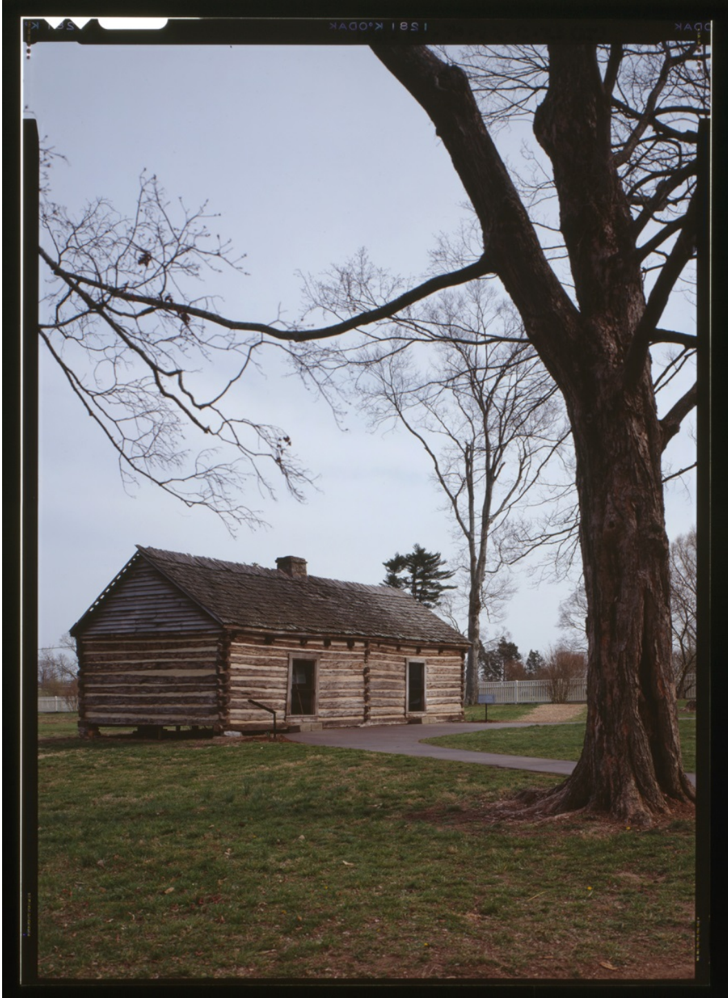
Fig. 15. Alfred's Cabin at The Hermitage. An example of a saddle-bag form type. Library of Congress, Prints & Photographs Division, HABS TN-52-C.
