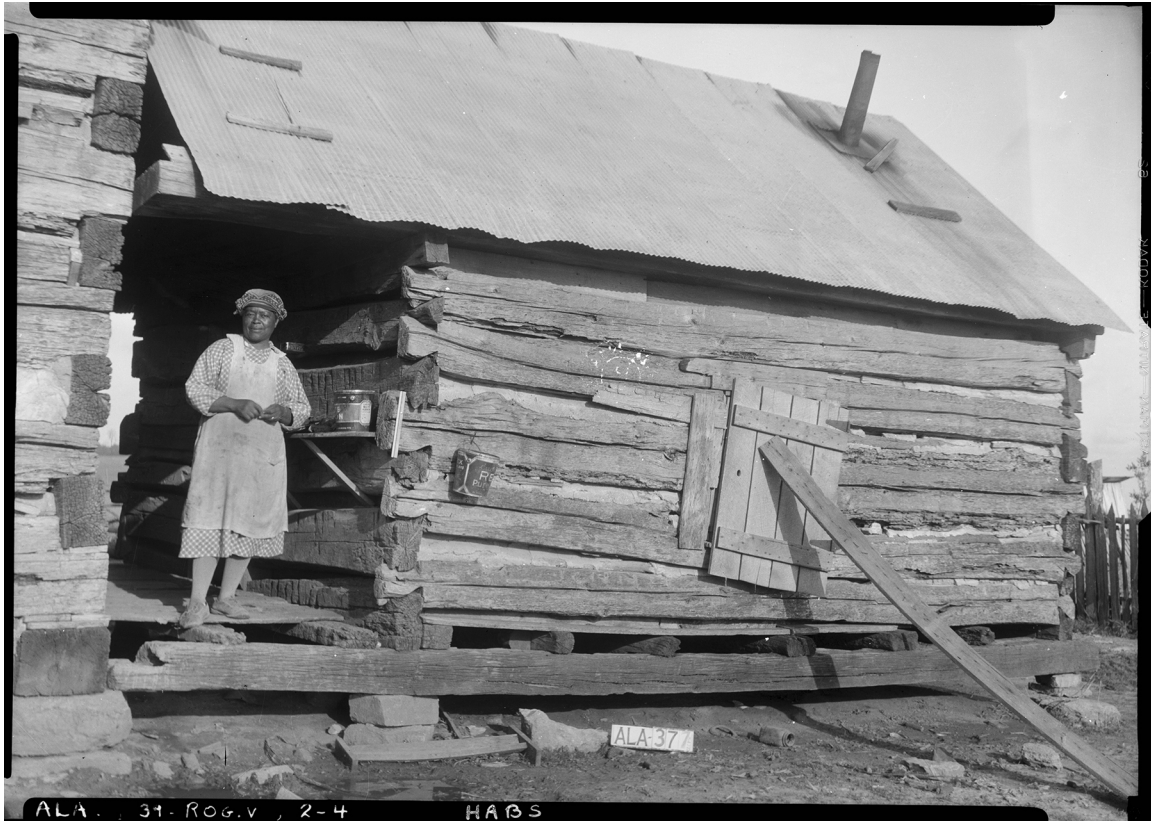
Fig. 45. Detail of the first Taylor-Cunningham House showing half-lap corner notching on the dogtrot house and half-dovetail notching on the kitchen addition (likely a later). Library of Congress, Prints & Photographs Division, HABS AL-377-A.
