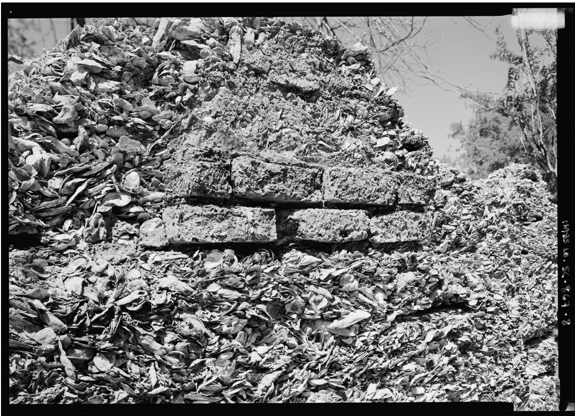
Fig. 10. Detail of tabby construction at Haig Point, Beaufort County, South Carolina. Library of Congress, Prints & Photographs Division, HABS SC-867.
