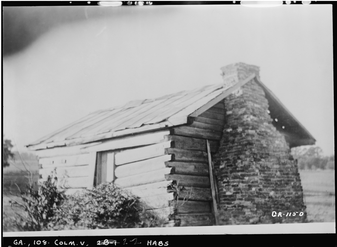
Fig. 51. Detail of a log slave house with half-lap square notching, a brick chimney and a plank roof at the Bass Place. Library of Congress, Prints & Photographs Division, HABS GA-1150.
