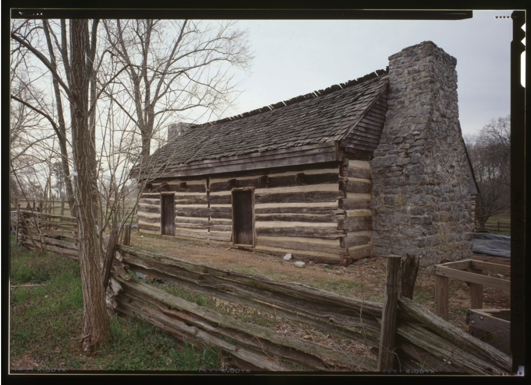
Fig. 16. East Cabin at The Hermitage. An example of a double-pen form type. Library of Congress, Prints & Photographs Division, HABS TN-52-B.
