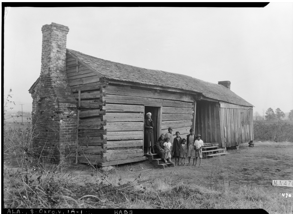
Fig. 29. Dogtrot house in Calhoun County, Alabama with half-dovetail notching and a brick chimney with a family of eight living in the house. Library of Congress, Prints & Photographs Division, HABS AL-470.
