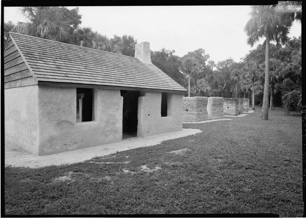
Fig. 8. Exterior view of a reconstructed slave house at Kingsley Plantation, Monroe County, Florida. Library of Congress, Prints & Photographs Division, HABS FL-478-A.
