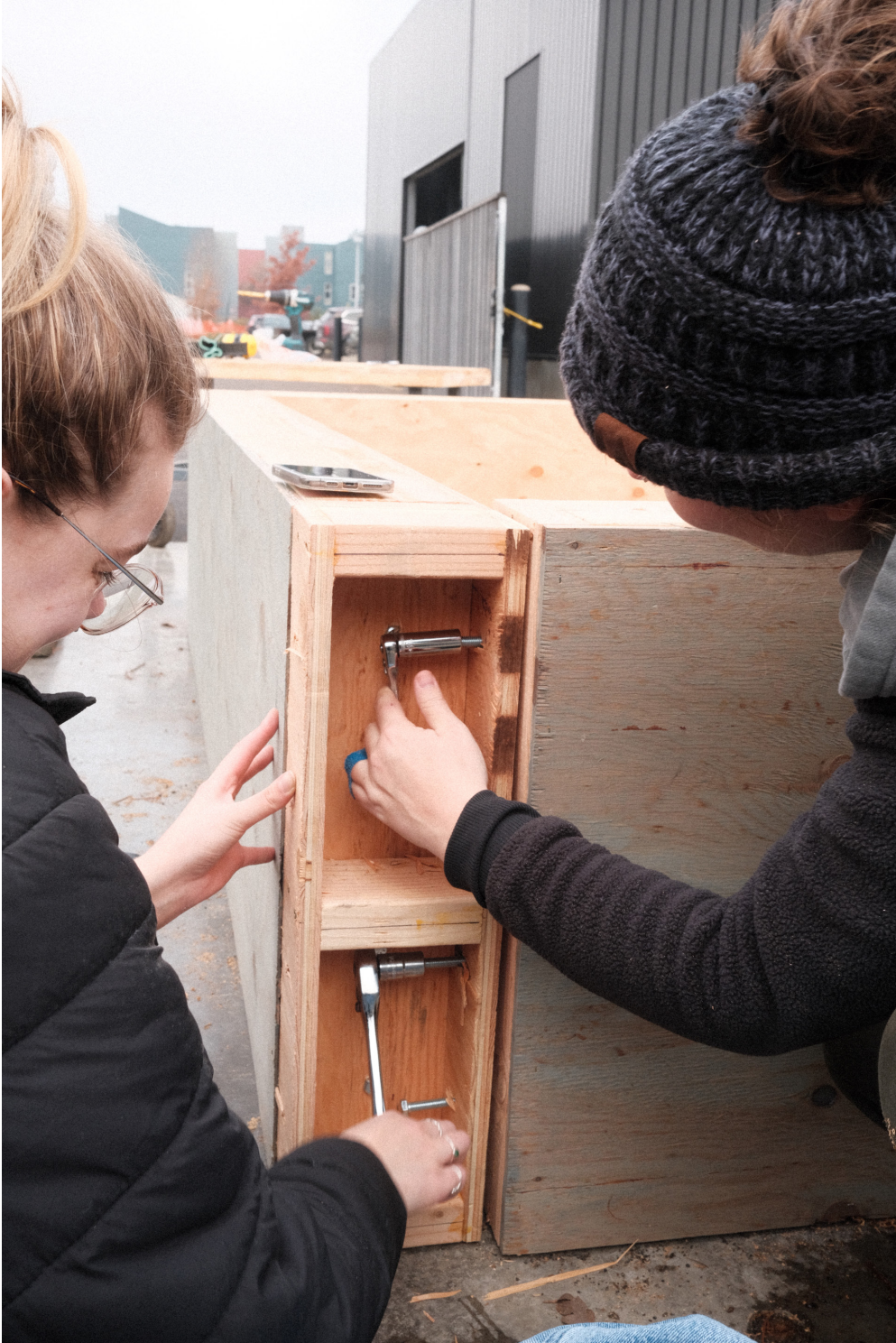
FIG. 41 Connection of panels through the bracket connections.
