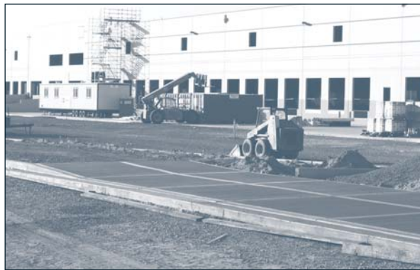
New construction in Rivergate
