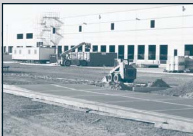
New construction near Terminal 6.
