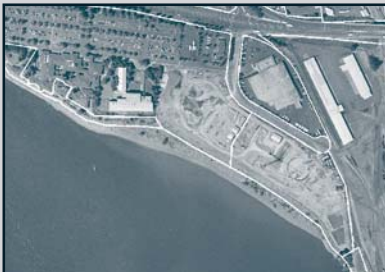
Vacant site currently used for City's "Big Pipe" project.
