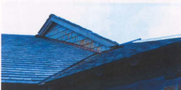
Fig. 81 Copper flashing on gable wall and east wing connection, flashing trough in roof connection. View facing SE
