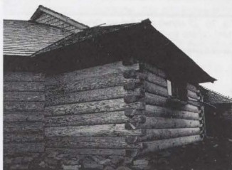
Fig. 30 Note unweathered replacement logs under eaves and patina of original logs protected by eaves. Stones replicating the historic dry-stacked foundation cover a contemporary concrete foundation. E Pavilion, view facing west.
