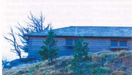
Fig. 85 Single-lite hopper windows on east wing. View Facing W
