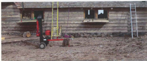
Fig. 60 The east wing foundation is in good condition from repairs in 2006. Facing NE
