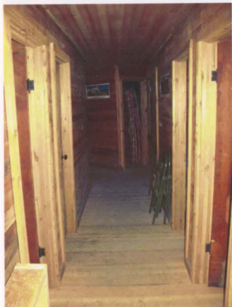
Fig. 93 Douglas fir tongue and groove on floors, walls, and ceilings in the east wing. This wing is in excellent condition as it was repaired in 2006. Note lack of light fixtures. View down east wing hallway. View facing E
