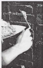
This mortar is the proper consistency for repointing historic brick. Photo: John P. Speweik.
