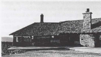
Fig. 25 The south elevation of the west wing View facing north. OHS collection photo
