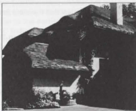
With the popularity of the revival of historic styles in the late 19th and early 20th centuries, a new technique was developed to imitate English thatch roofs. Photo: C.H. Roofing.
