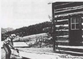
A log to replace the deteriorated sill is being hewn in the traditional manner with a broad axe. Photo: NPS files.
