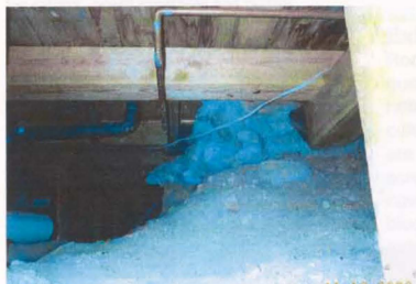
Fig. 68 2002 photo by Nancy Niedernhofer, from Oregon SHPO collection. Notice timber floor joists at chimney footing. Facing E
