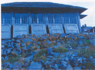
Fig. 9 West wing 18 pane wood sash case-ment windows c. 1930 replaced two pairs of 4-over-4 double hung windows. Brick chimney from 1940.
