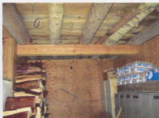
Fig. 22 Log floor joists are visible from wood storage area. The tops are flattened and bottoms notched to fit timber girder.
