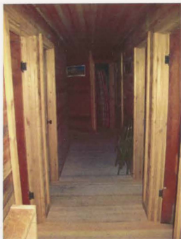
Fig. 15. East wing hallway with Douglas fir tongue and groove ceiling, walls, and floor.
