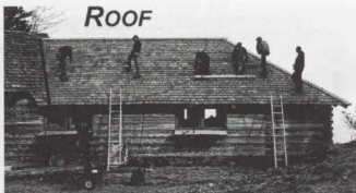
Fig. 32 Crag Rats assess roof conditions for winterization at the end of the 2011 season. View facing NE
