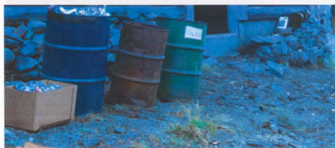
Fig.63 The foundation on the north side of the west wing is in good condition. Rocks applied to the outside of the modern concrete foundation should be reapplied around the basement doorway. Facing SW
