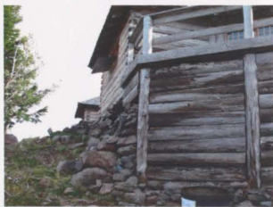
Fig. 10 Wood retaining wall outside basement wood storage area with north deck above.
