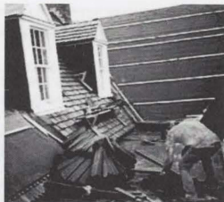
The replacement shingles matched the historic shingles and were of such high quality that little hand dressing was needed at the site. Photo: John Ingle.
