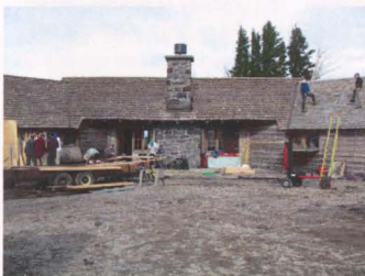
Fig. 53 South side facing north. This location was historically barren.
