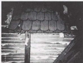
These weathered historic 19th-century handsplit and dressed shingles were found in place under a later altered roof. See also, below. Photo: John Ingle.
