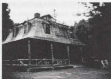
This lodge constructed of logs in the 1880s is an example of the Adirondack style of rustic camp architecture. Photo: NPS files.
