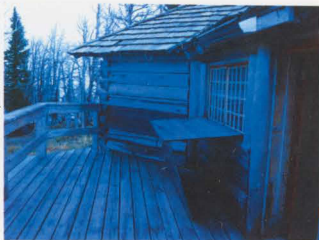
Fig. 71 North deck in good condition. View facing east.
