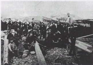
Fig. 8 Hand hewing heavy timbers for log construction 1888. Photo from Crags Rats' collection.
