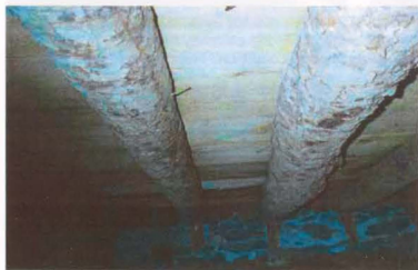
Fig. 69 2002 photo by Nancy Niedernhofer, from Oregon SHPO collection. Floor joists in west wing. Facing W
