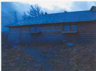
Fig. 7 East wing, east elevation. Note log ends protrude from the extension to wing in 1928. This element has been replaced in-kind to interpret the alteration. Shuttered single plan hopper windows.
