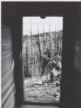
Fig. 49 The proximity of fire damage to the inn is currently highly visible. View SE out the west wing doorway.
