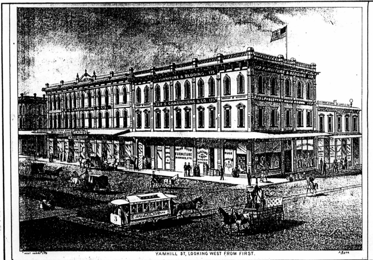
Fig. 67. Visual material which should be photocopied for the Project's files. (Source. A. Burr, "Stowbridge Building, Yamhill St., Looking West from First," Lithograph, West Shore , 1883, as reproduced in William John Hawkins, III, The Grand Era of Cast-Iron Architecture in Portland . (Portland: Binford and Mort, 1976), 82.)
